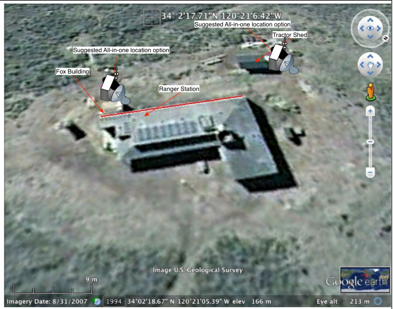
Figure 3.2: San Miguel Ranger Station Aerial view. Provides view of buildings identifying two possible all-in-one unit installation locations.
