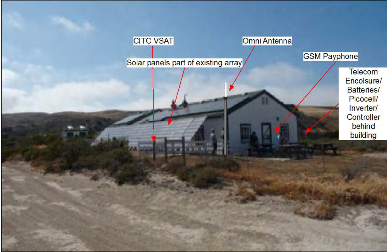
Figure 17.2: Santa Rosa Island Power/Generator Station Photograph.
