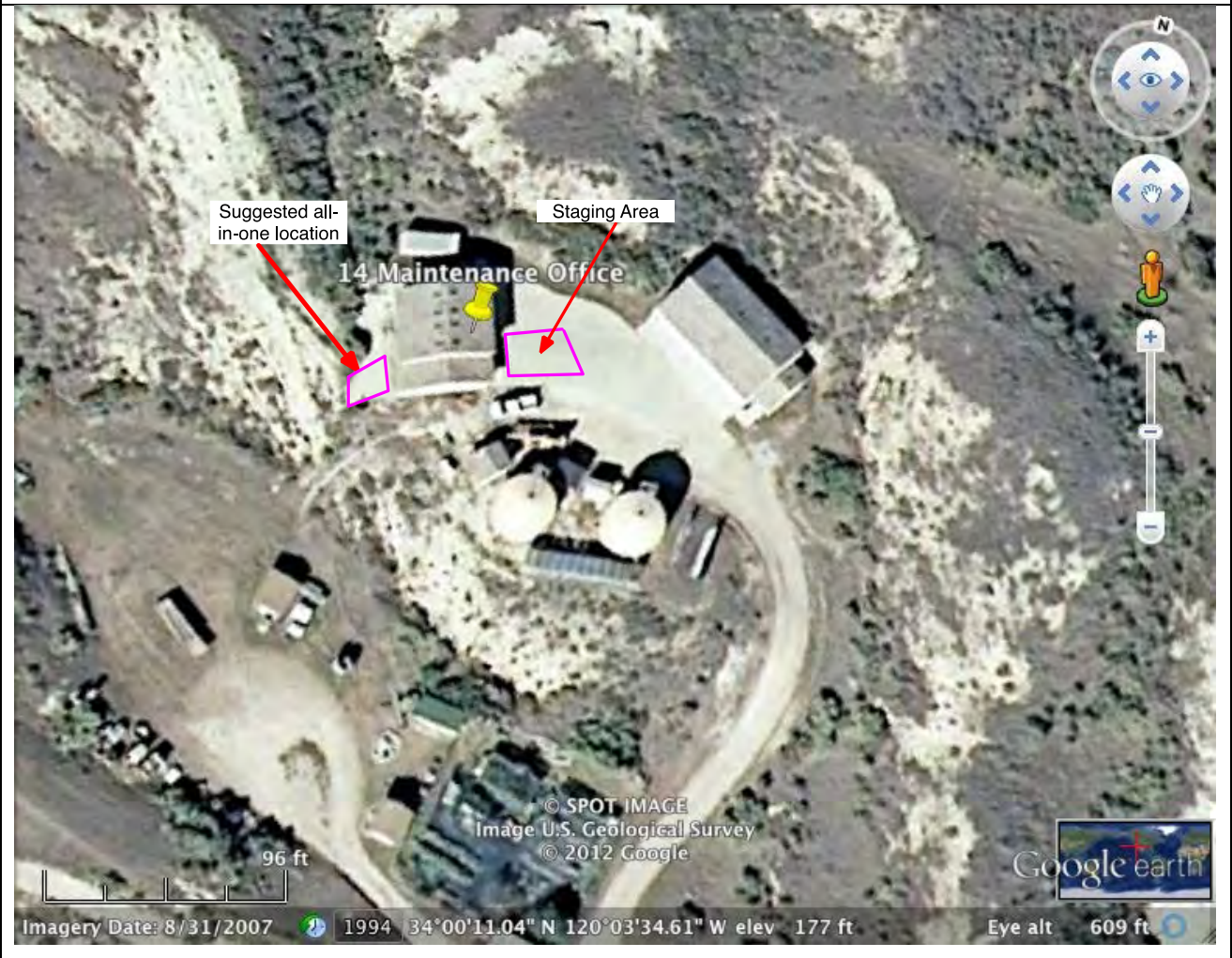
Figure 14.3: Maintenance office staging area. No digging required for wiring. All options require no wire suspension, aboveground conduit, or trenching to connect equipment because the telecom enclosure, CITC VSAT, antenna, and solar panels are all seated on the all-in-one solution or structure. All wiring would be affixed to the structure using cable mounts.
