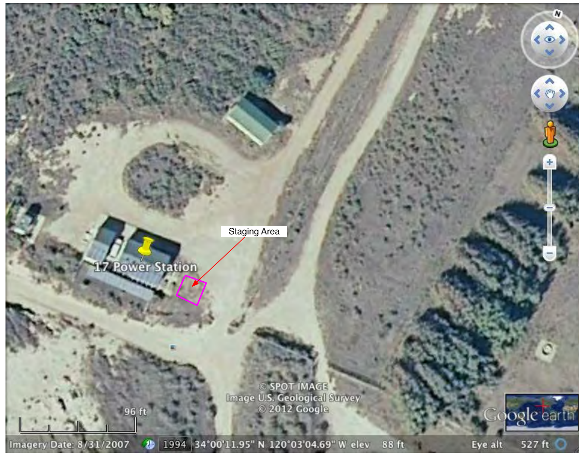
Figure 17.3: Power station staging area. No digging required for wiring. All options require no wire suspension, aboveground conduit, or trenching to connect equipment because the telecom enclosure, CITC VSAT, antenna, and solar panels are all seated on or around the structure. All wiring would be affixed to the structure using cable mounts.
