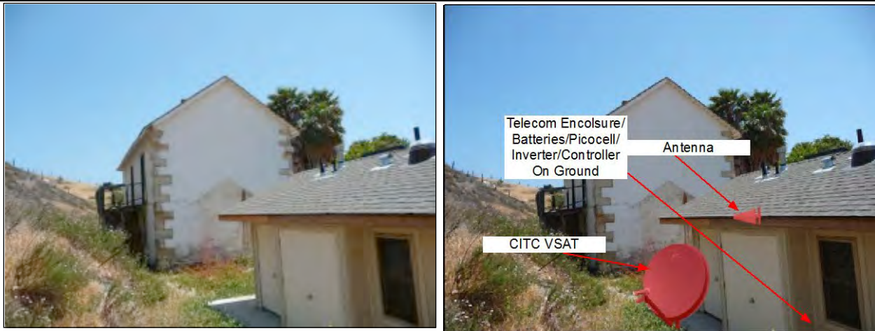
Figure 9.3: Santa Cruz Island Smugglers Adobe Photograph #2 with Existing Condition (left) and with Proposed VSAT Dish and Yagi Antenna Added (right).
