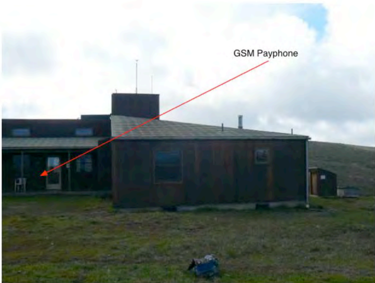
Figure 3.1: San Miguel Island Ranger Station Photograph Front view showing GSM payphone location and southwest view of building.
