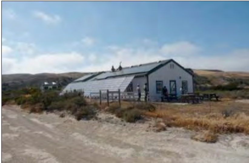
Figure 17.1: Santa Rosa Island Power/Generator Station Photograph.
