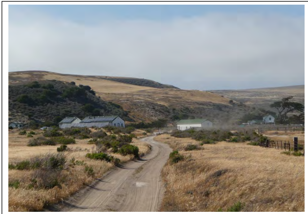
Photograph 2. Southern end of the main ranch cluster, facing northwest. From left to right: non-contributing NPS generator complex (power station), World War II-era storage building (non-contributing), and Upper Ranch House (contributing).
