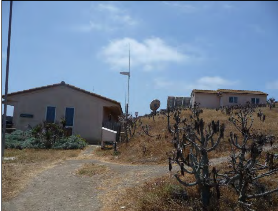
Photograph 1. Santa Barbara Island Ranger Station, showing main building at left and maintenance shop at right, view facing south. (JRP Historical Consulting, LLC)
