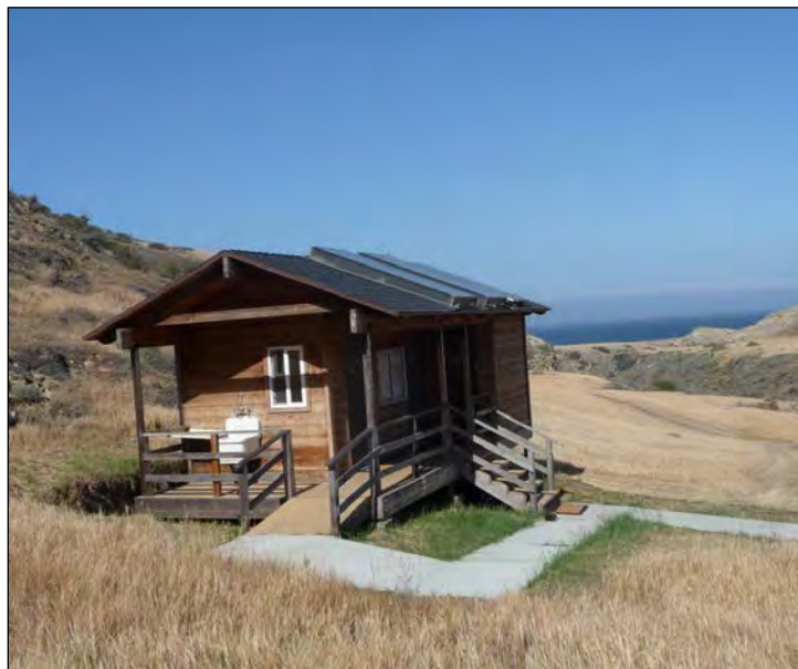
Photograph 19. Campground restroom, view facing northeast along trail to Bechers Bay (right). (JRP Historical Consulting, LLC)
