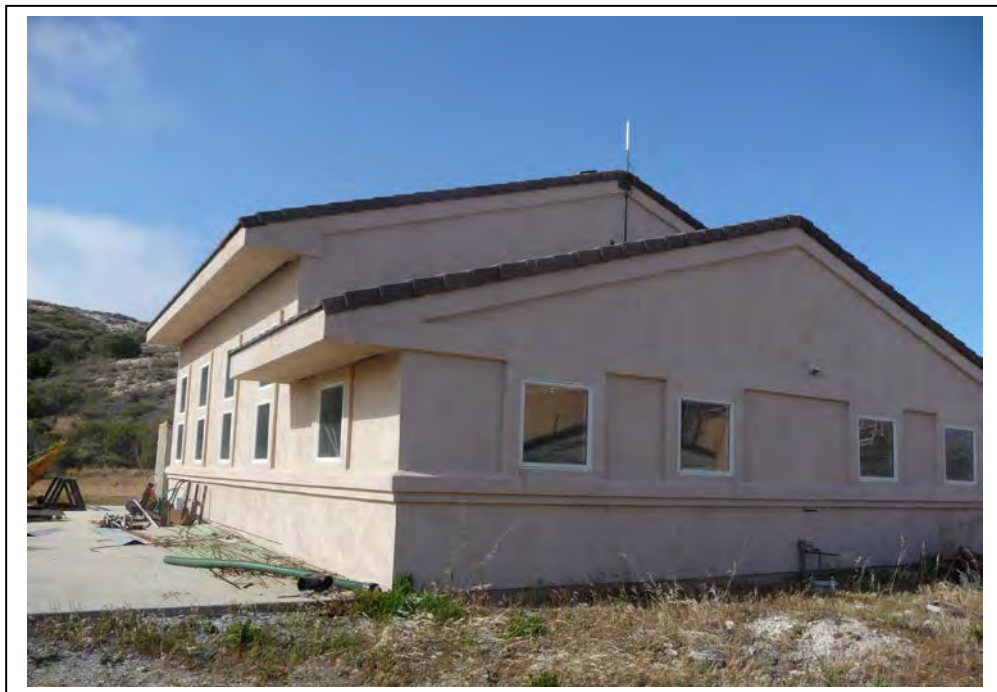
Photograph 5. Maintenance office in non-contributing cluster, view facing west.
