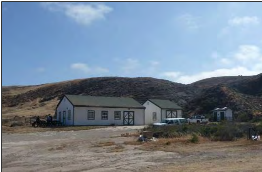
Photograph 26. From left to right, generator building, fuel storage building, and two restrooms, view facing southwest. (JRP Historical Consulting, LLC)
