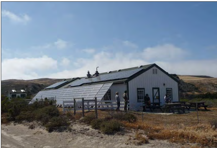
Photograph 25. Rear of generator building (power station), view facing northwest. (JRP Historical Consulting, LLC)
