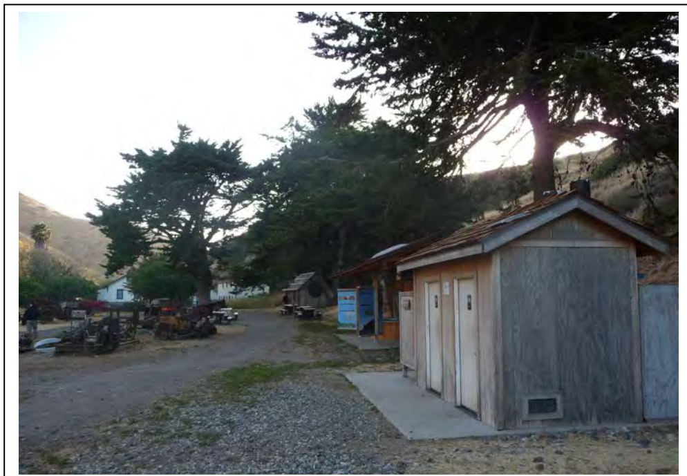
Photograph 3. Eastern end of Scorpion Ranch Cluster, showing non-contributing restroom and kiosk in the foreground, contributing ranch house complex in the background; view facing west.
