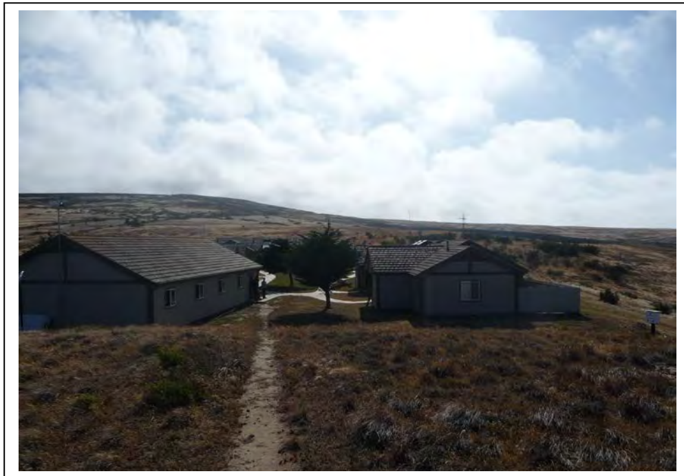
Photograph 6. Santa Rosa Island Housing Area (non-contributing cluster), view facing west.
