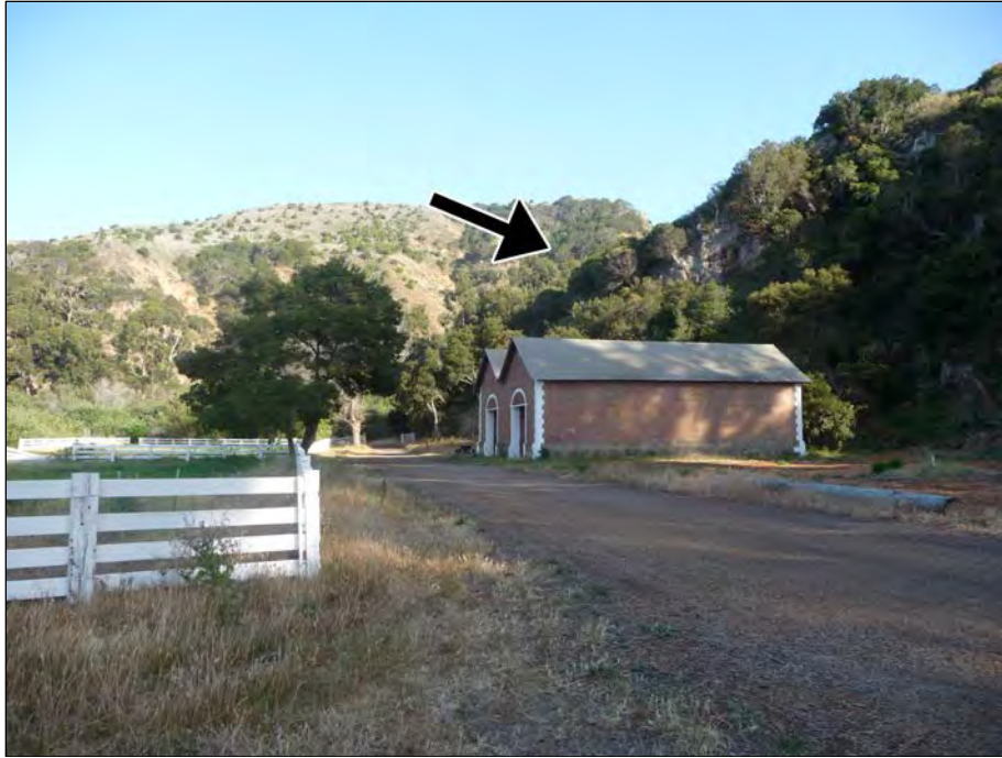
Exhibit 7. Proposed installation site for all-in-one unit, located in the valley behind the ridge indicated by the black arrow. (JRP Historical Consulting, LLC)
