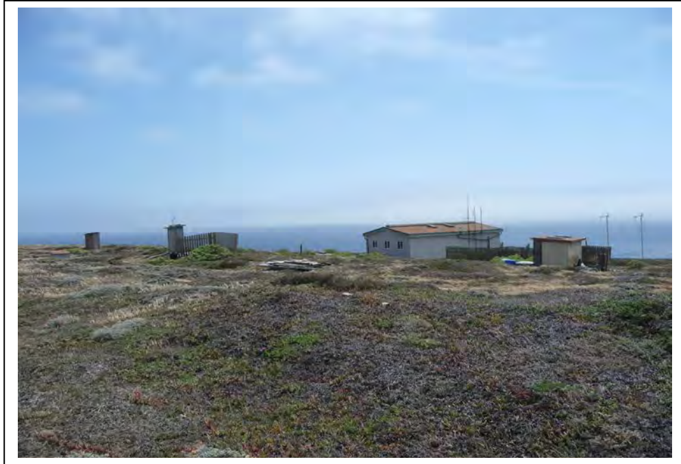
Photograph 2. Overview, showing main station building and small ancillary structures, facing southwest.
