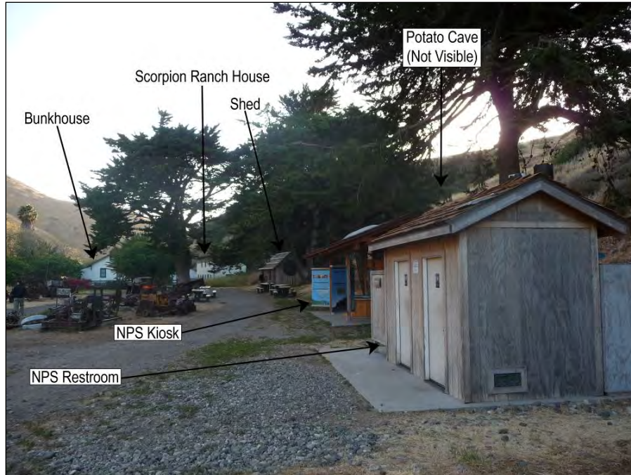
Photograph 8. East end Scorpion Ranch Cluster, facing southwest. The Bunkhouse, Scorpion Ranch House, Shed, and Potato Cave are contributors to the district; the NPS restrooms and kiosk (foreground) are non-contributors. (JRP Historical Consulting, LLC)
