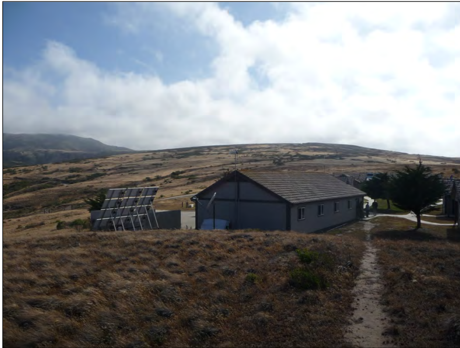
Exhibit 19. Proposed installation site for the all-in-one telecommunications unit, on the ground to the right of the garage building (center). View facing west, away from Main Ranch cluster, which is located about one mile away. (JRP Historical Consulting, LLC)
