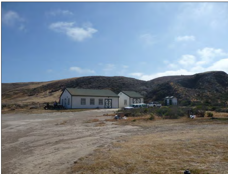
Exhibit 23. View toward the generator complex from the non-contributing World War II-era shed, facing south. The VSAT dish and equipment cabinet would be installed behind the generator building (at left), and the payphone and omni-directional antenna would be installed on the east (left) side of the building. (JRP Historical Consulting, LLC)
