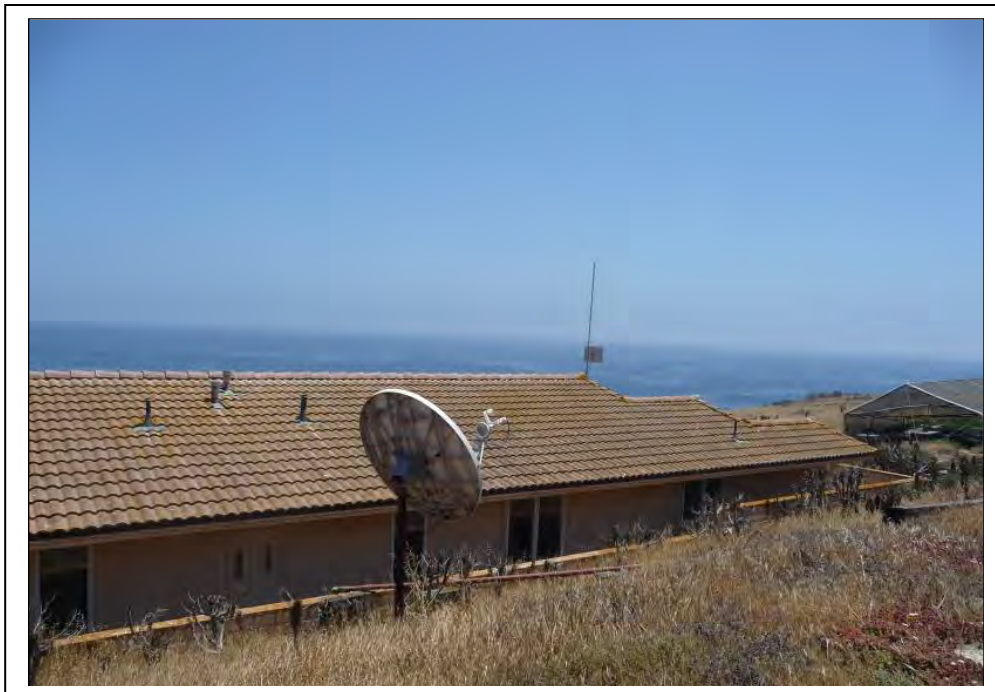
Photograph 2. West side of ranger station building, greenhouse visible at far right, facing southeast.
