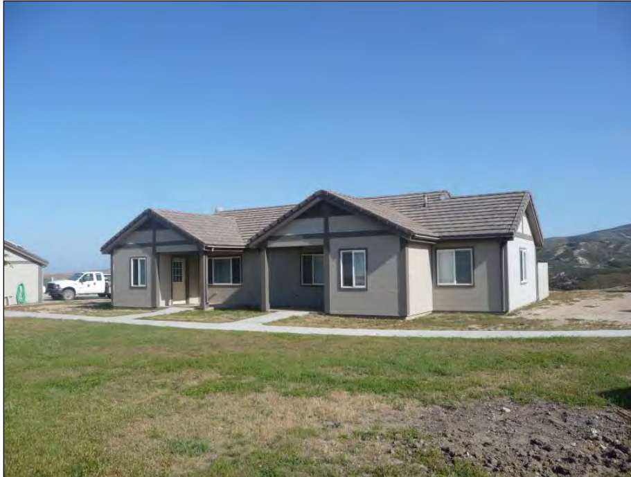
Photograph 23. Representative duplex in the Santa Rosa Island Housing Area, facing south. (JRP Historical Consulting, LLC)
