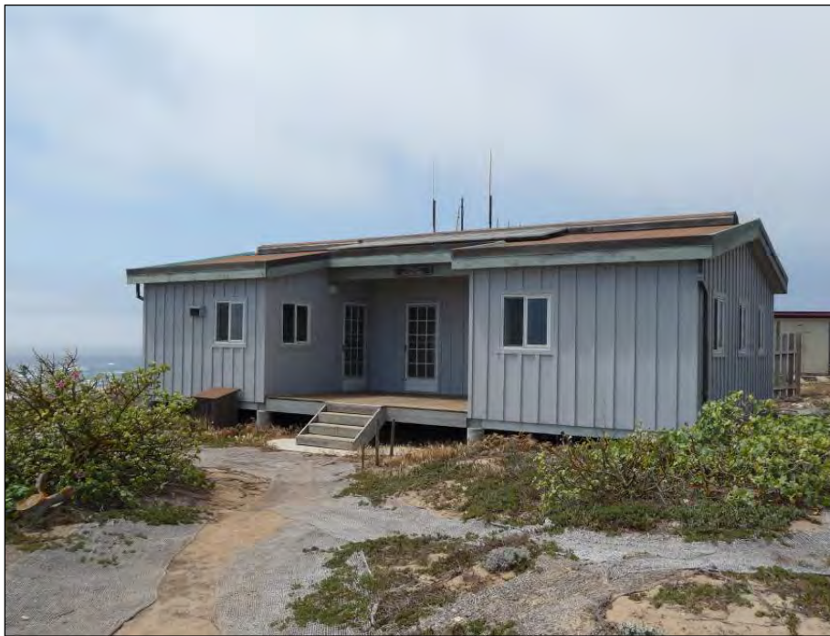
Photograph 4. San Miguel Island Marine Mammal Research Station, facing northwest. (JRP Historical Consulting, LLC)
