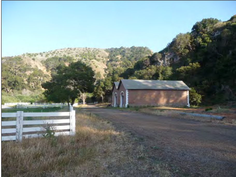
Photograph 11. View of warehouse at Prisoners Harbor cluster, facing east from east edge of pier and picnic area. (JRP Historical Consulting, LLC)
