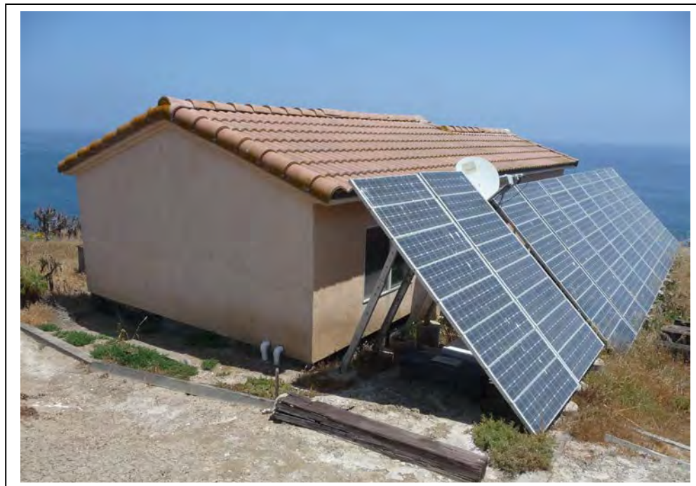
Photograph 3. Rear view of maintenance shop and solar panel array, facing northeast.
