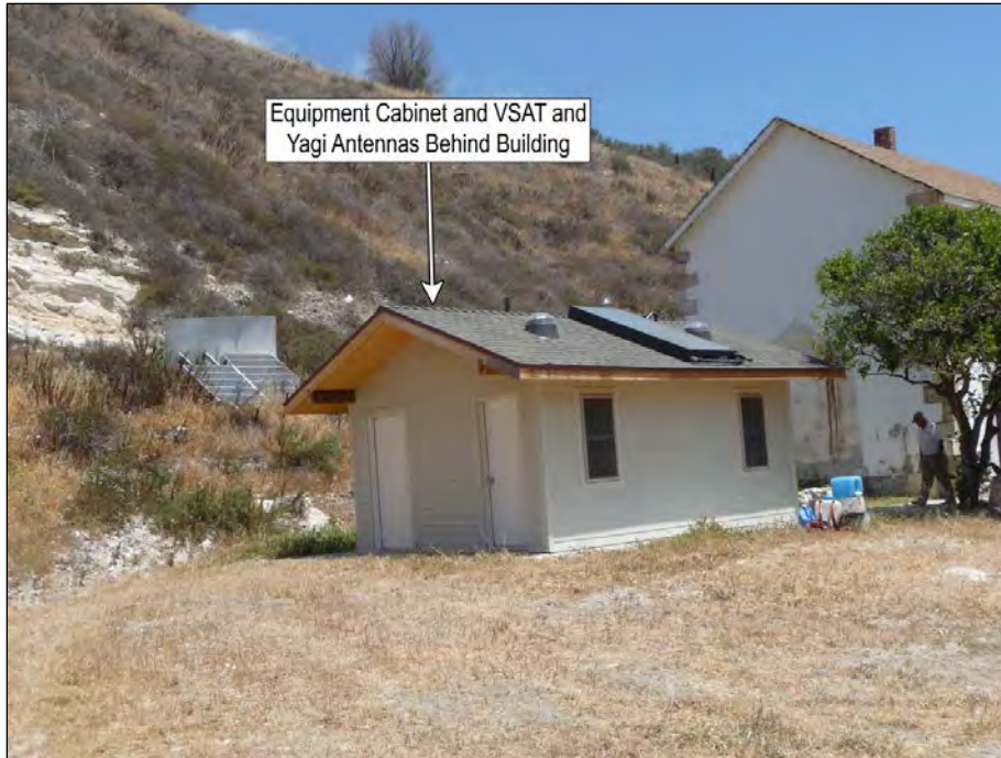
Exhibit 9. Placement of equipment installations behind NPS restroom building, facing northeast toward ranch house (at right). (JRP Historical Consulting, LLC)
