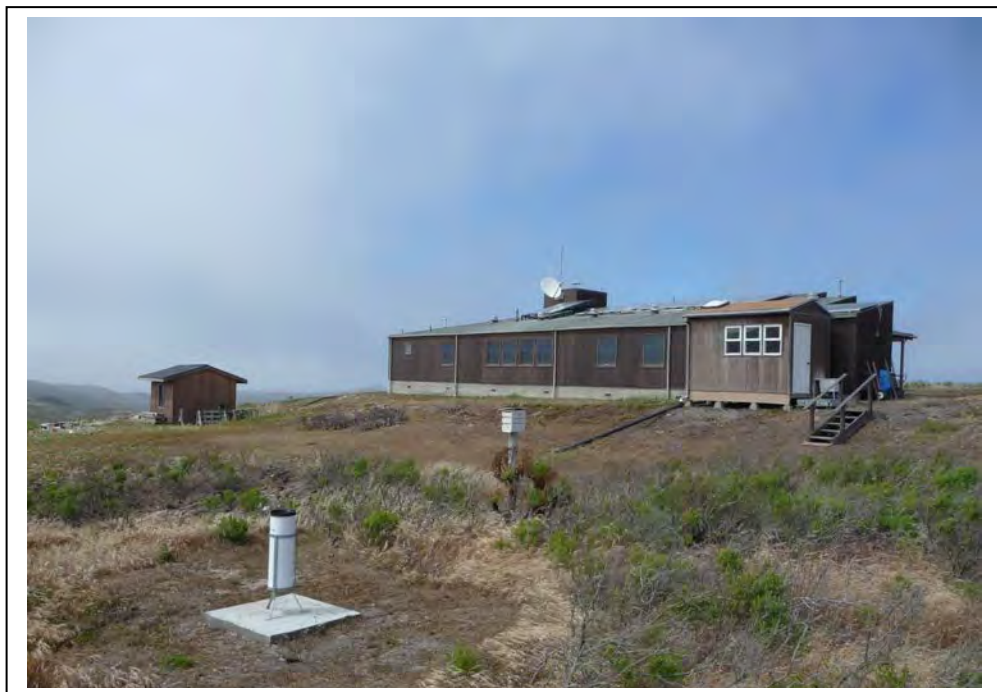
Photograph 3. Tractor shed (left) and fox building (right) at rear of ranger station, view facing north.
