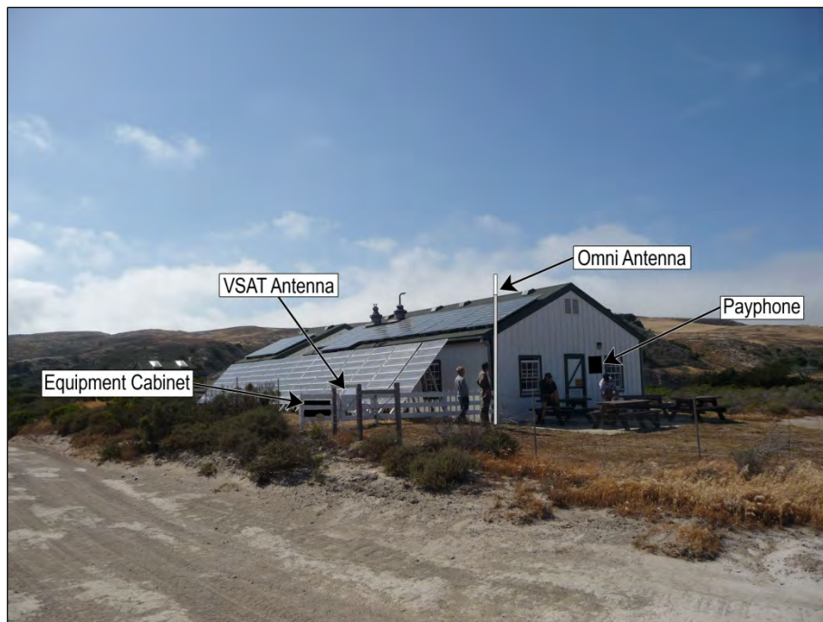
Exhibit 21. Simulated view of proposed telecommunication equipment at generator complex, facing northwest. (JRP Historical Consulting, LLC)
