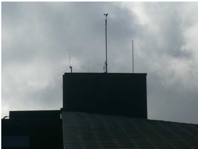
San Miguel Ranger Station Front View Lat 34° 2'17.71"N Long 120°21'6.42"W
