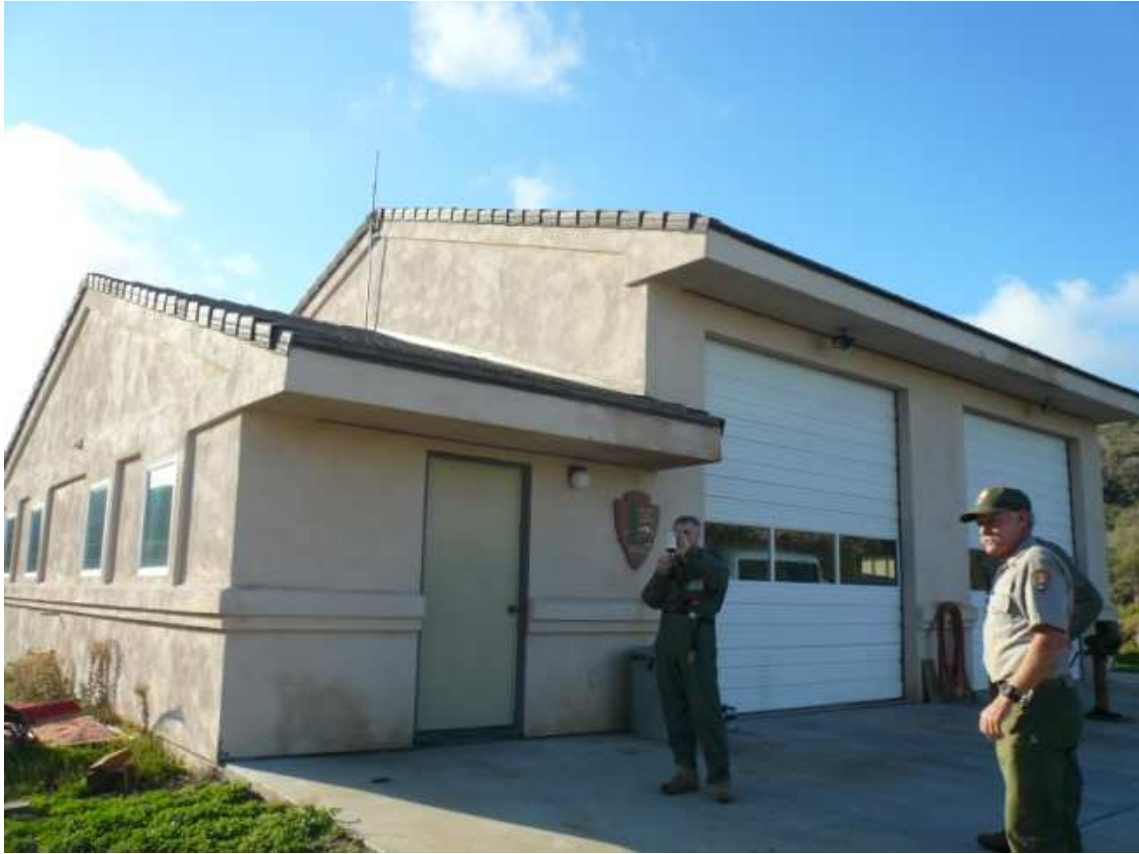
Figure 19 A – Santa Rosa Maintenance Office
