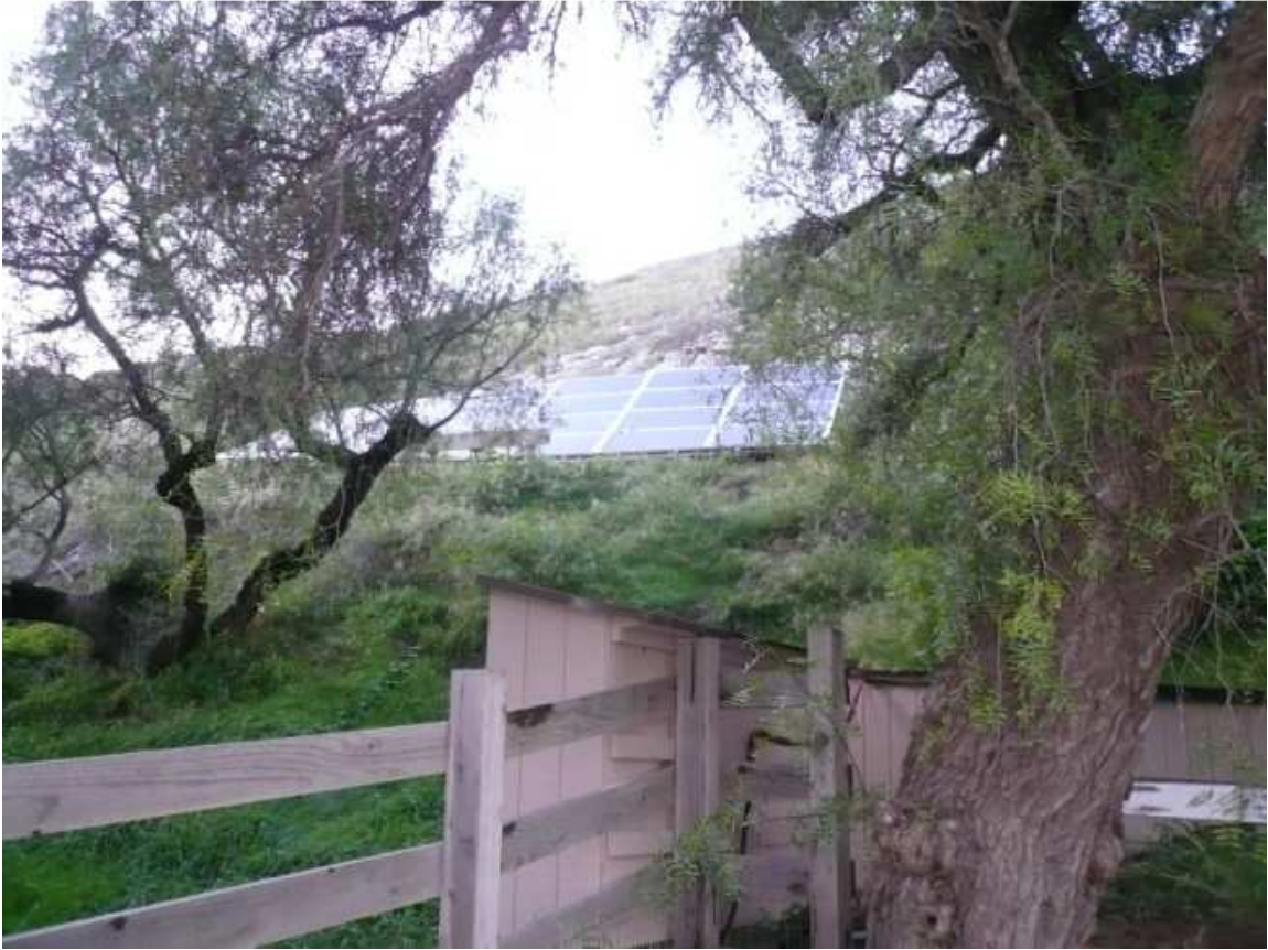
Figure 28 B – solar panel and housing at Scorpion Adobe
