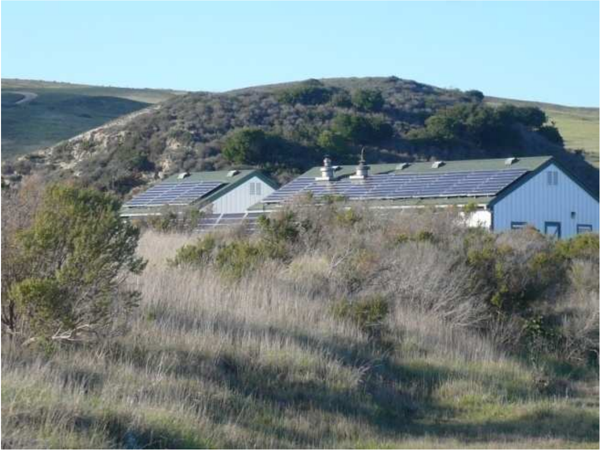
Figure 14 B – Santa Rosa Power Station (another view)
