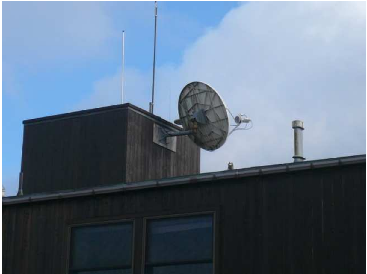
Figure 6 A – San Miguel Ranger Station existing Internet VSAT system Lat 34° 2'17.71"N Long 120°21'6.42"W
