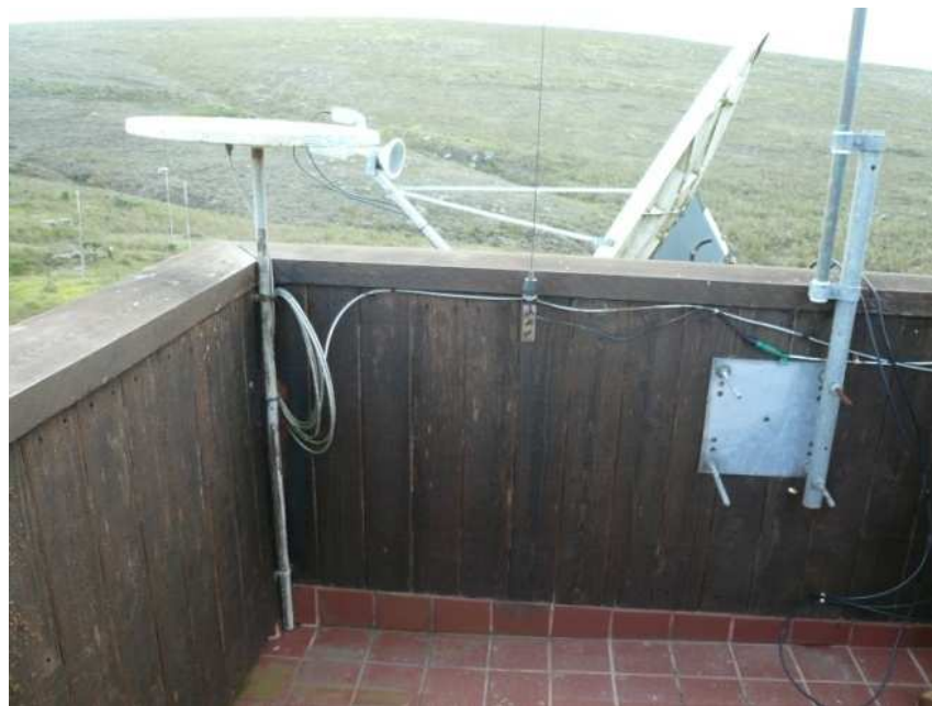
Figure 5 – San Miguel Ranger Station roof Lat 34° 2'17.71"N Long 120°21'6.42"W
