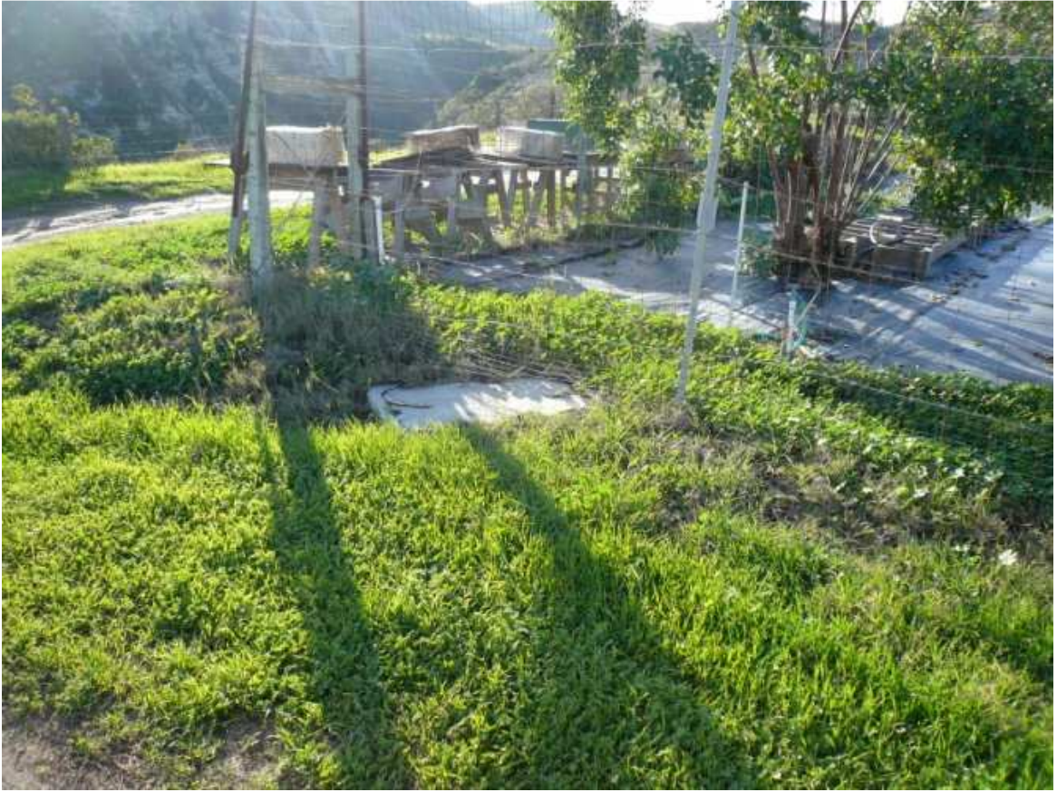
Figure 20 – ¾ inch conduit ingress/egress from power plant to maintenance area
