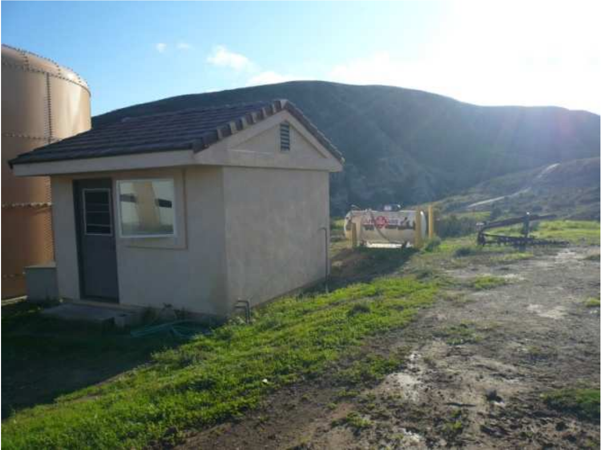
Figure 21 A – propane shed and generator
