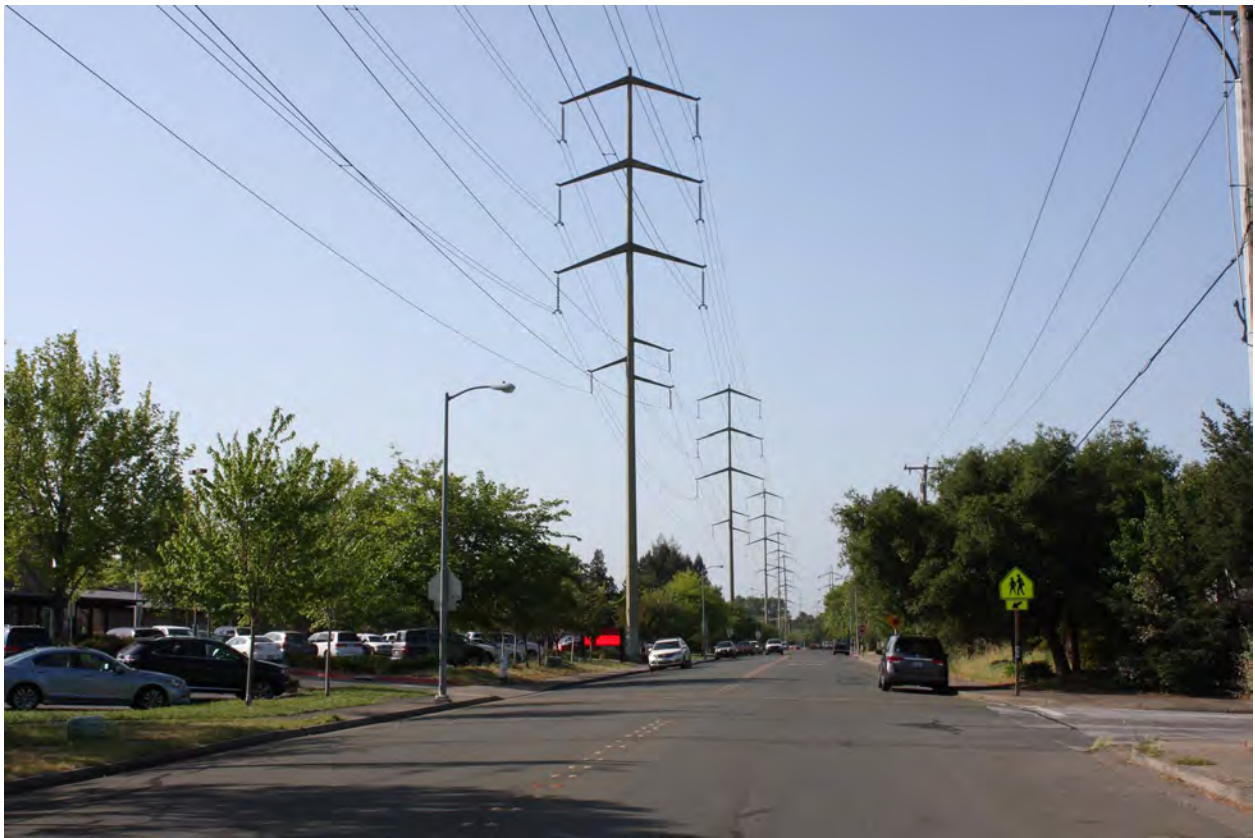
D. Faught Road near Corbett Circle looking south
