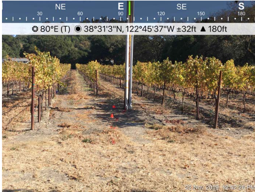
Figure 4: Photograph of Distribution Pole Work Area
