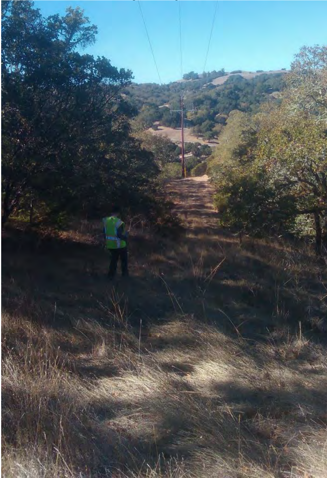
FFW14/15 – PS10; Pole 62; SW3 (photo facing north)
