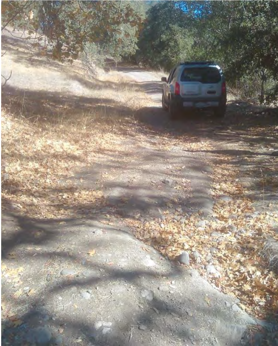
FFX4 – SEW45; Ephemeral water course which crosses the roadway (photo facing east)
