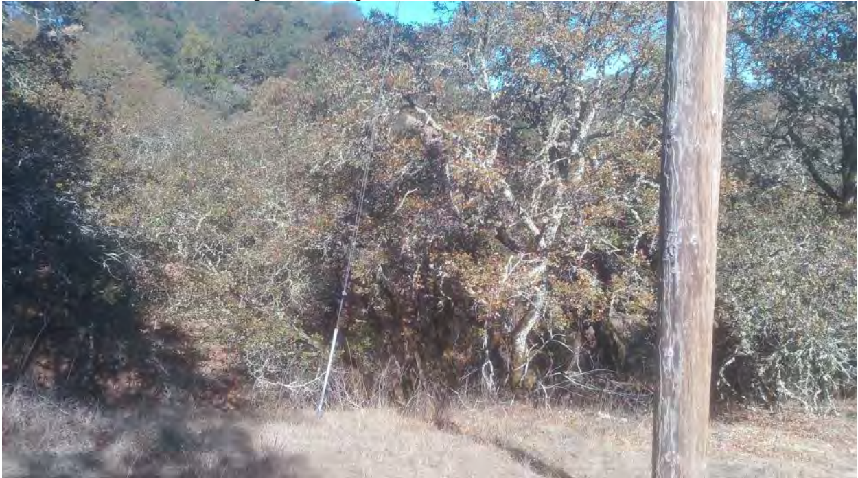
FFW10 – Pole 46; SEW16 (photo facing north)
