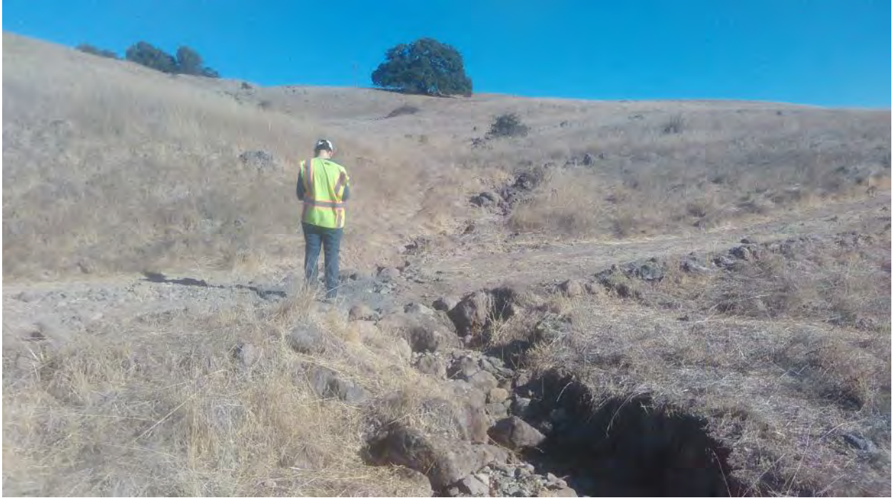
FFX21 – SEW5; Crossing point for seasonal watercourse (photo facing southeast)
