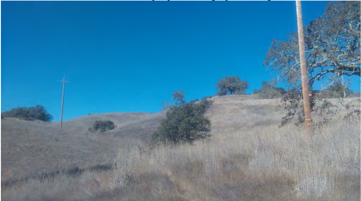
FFW19 – Pole 71; SEW35; Work area upslope of drainage (photo facing northeast)
