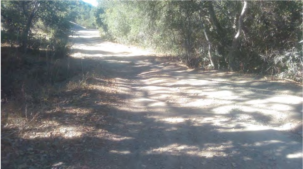
FFX12 – RIWO9; Culvert crossing on vineyard access road (photo facing west)
