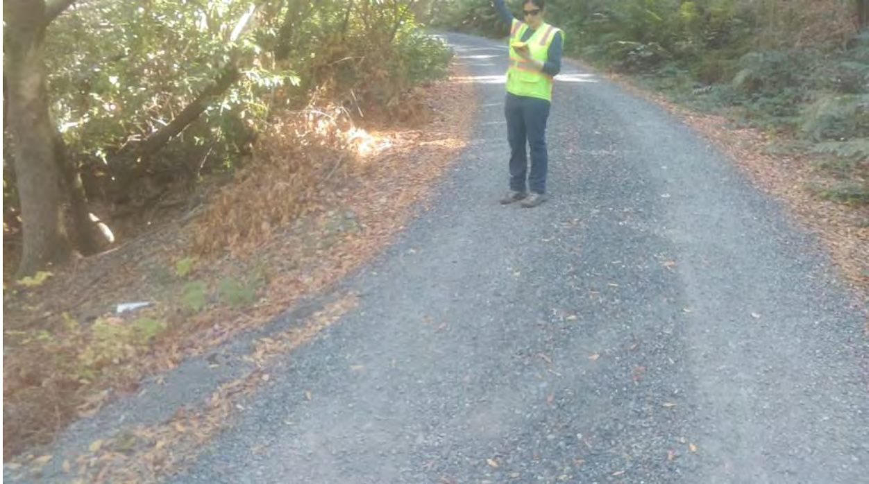
FFX18 – SEW46; Culvert crossing under improved road (photo facing east)
