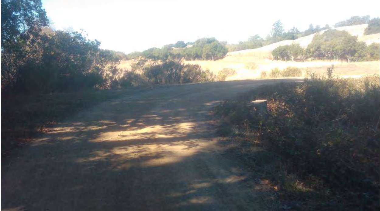
FFX13 – RIWO10; Culvert crossing occurs immediately downstream of perennial pond (photo facing northwest)
