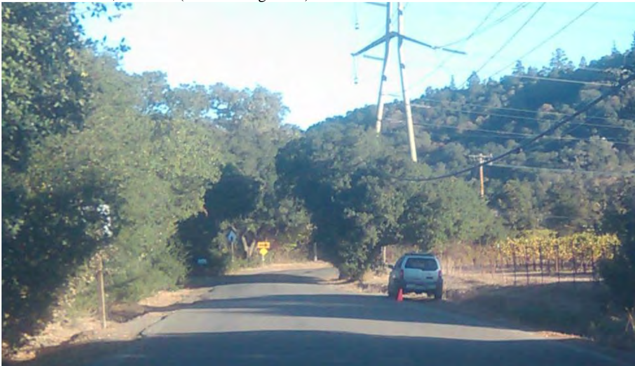
FFW4 – Pole 21; SEW9A (Photo facing north)
