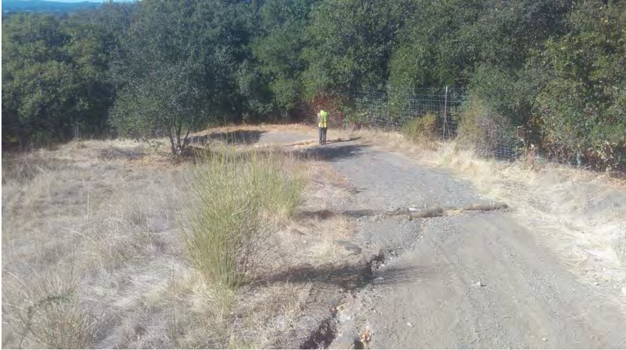
FFX1 – SEW44; Access road with seasonal surface flow and wattles (photo facing west)
