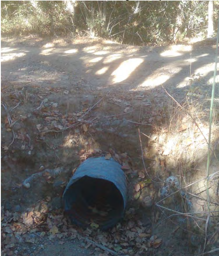
FFX12 – RIWO9; Culvert crossing on vineyard access road (photo facing west)
