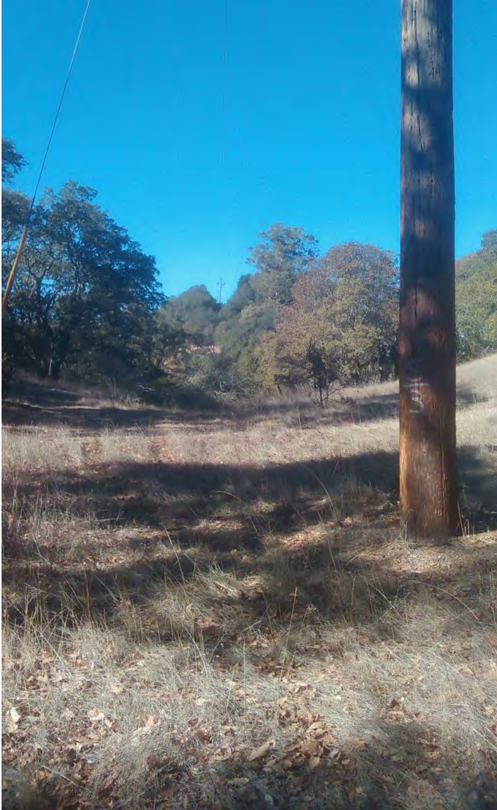
FFW13 – Pole 57; SEW24; Work area upslope from seasonal watercourse (photo facing north)
