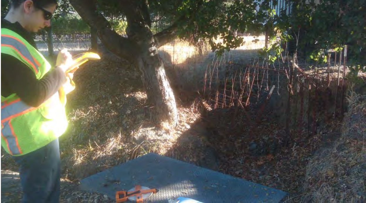
FFW1 – Pole 20; SEW41 Culvert at terminus of drainage (photo facing east)
