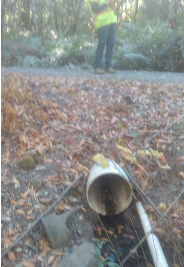
FFX18 – SEW46; Culvert crossing under improved road (photo facing east)
