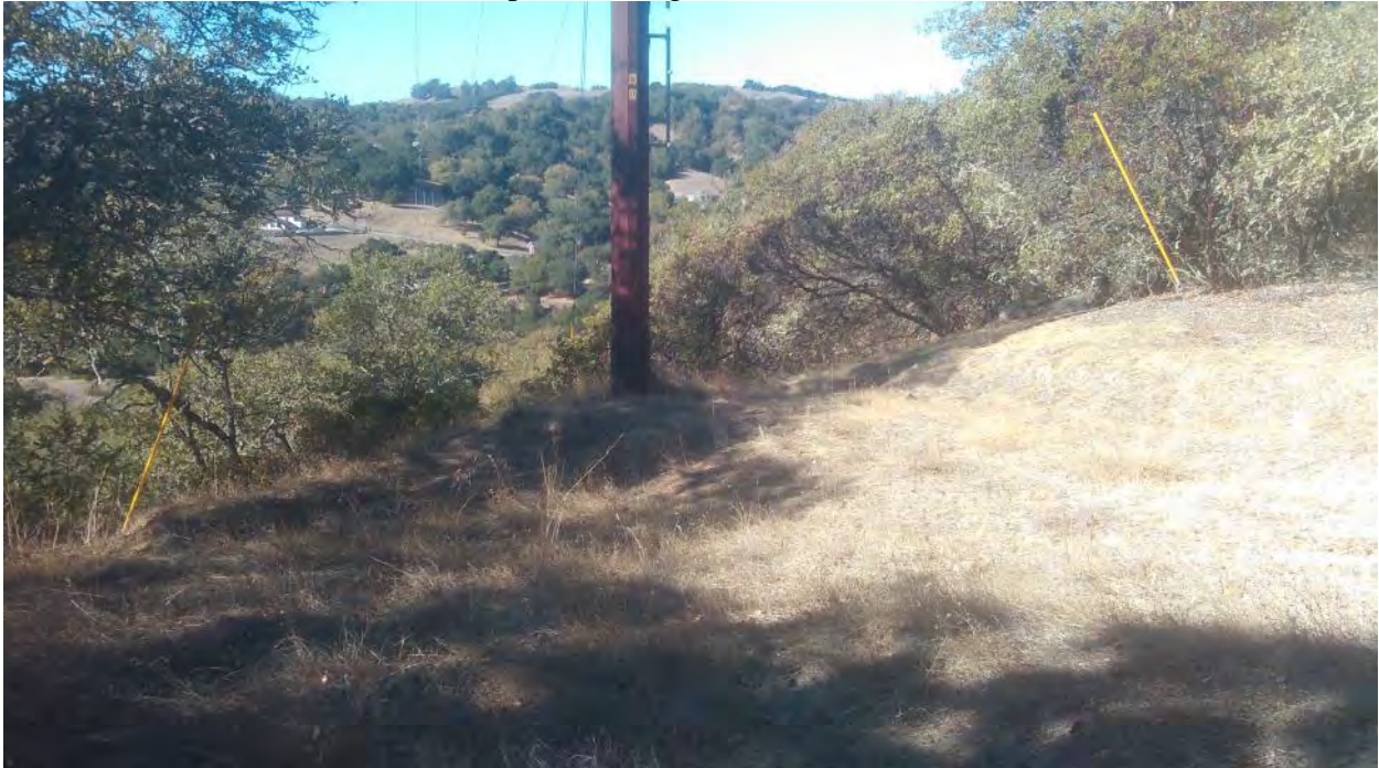
FFW14/15 – PS10; Pole 62; SW3 (photo facing north)
