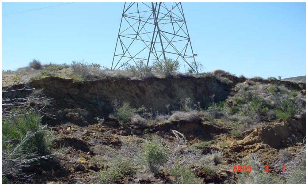
Midway-Vincent 500KV T/L M76-T1 Rotational Slide
