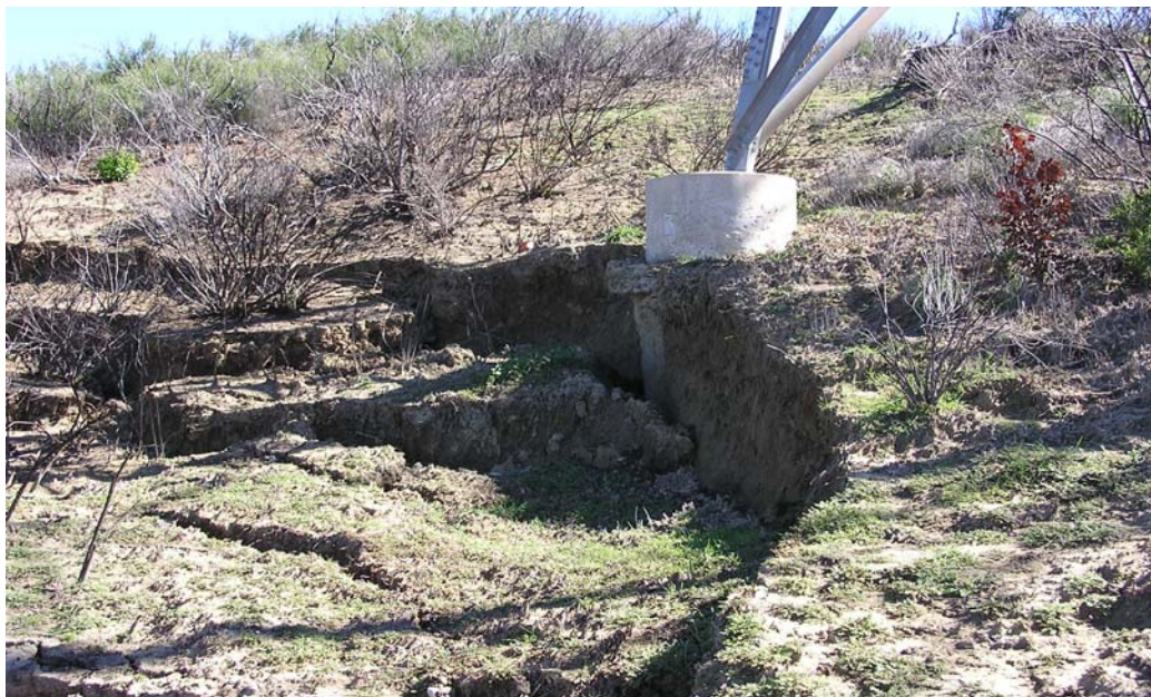
Midway-Vincent 500KV T/L M76-T1 Rotational Slide
