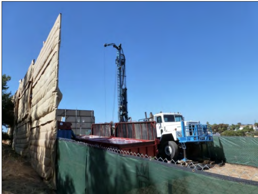
Figure 10 Sample Site-Erected Curtain-type Noise Barrier
