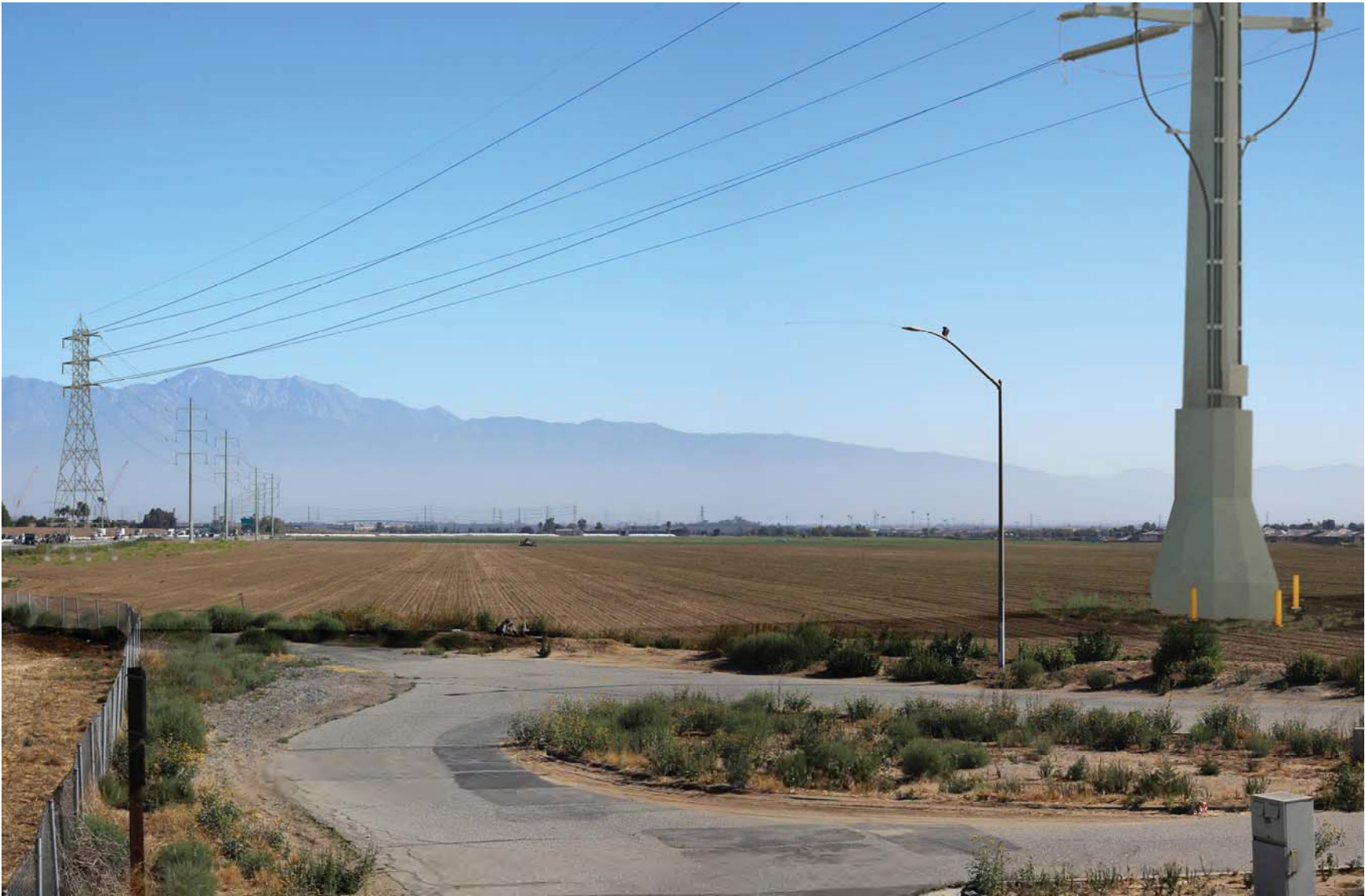
Figure 4.1-13 KOP 5 – Photosimulation (After Revised Project) – Limonite Avenue Park-and-Ride Looking North
