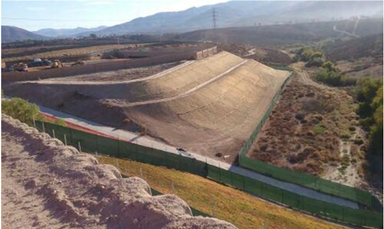
Figure 2.2-3 Site Development (November 4, 2016)
