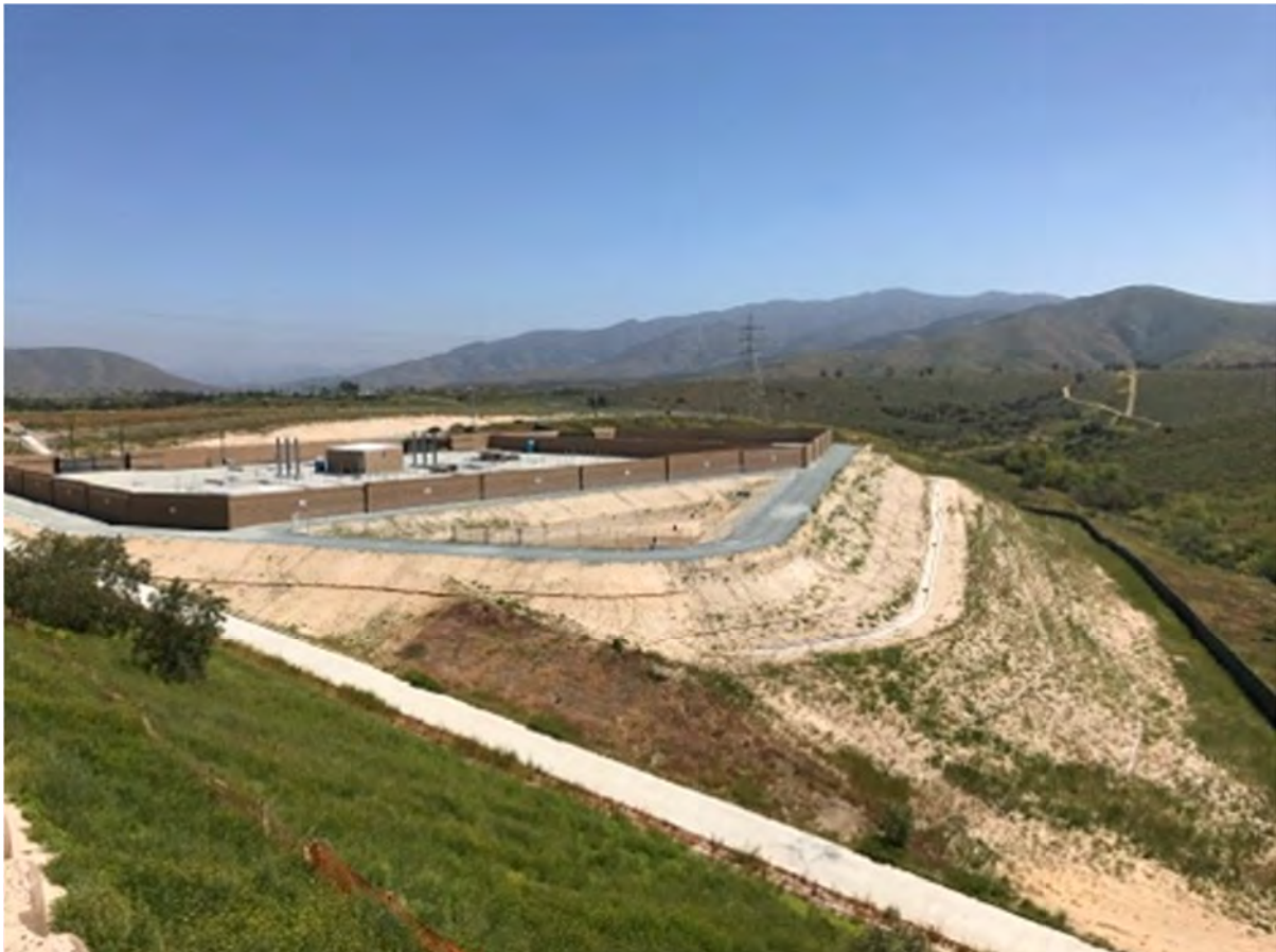
Figure 6.1-1 Conclusion of Site Development Phase
