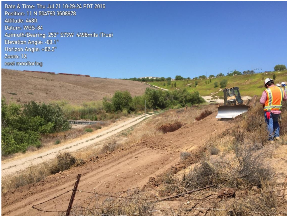
Fence access road (07/21/16)
