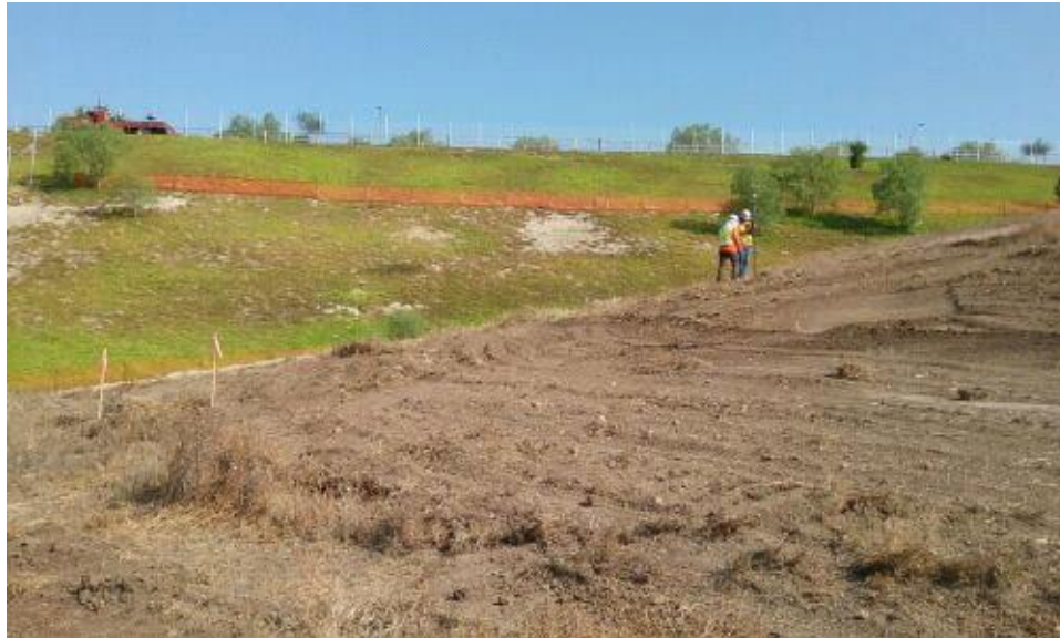
Caption Surveying for slope construction.
