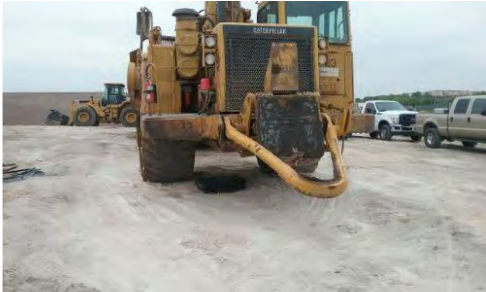
Caption Drip pans in place beneath equipment kept onsite overnight.
