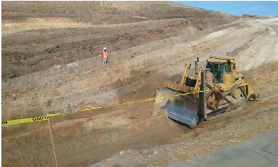
Caption Paleontological monitor observing excavation.
