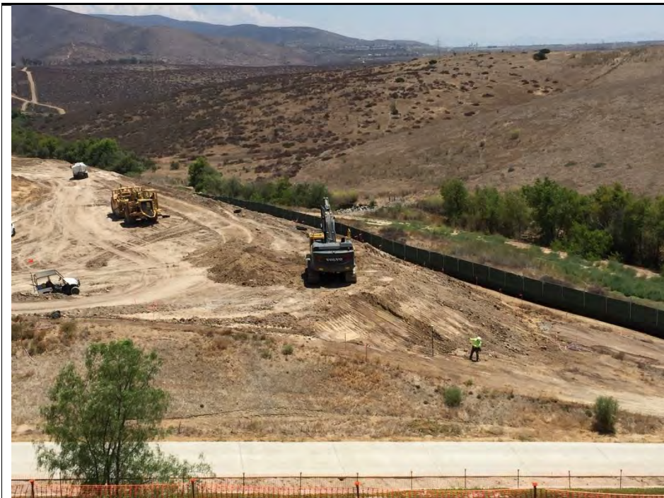
Photograph 4: Excavator working on substation pad slopes on August 12, 2016.
