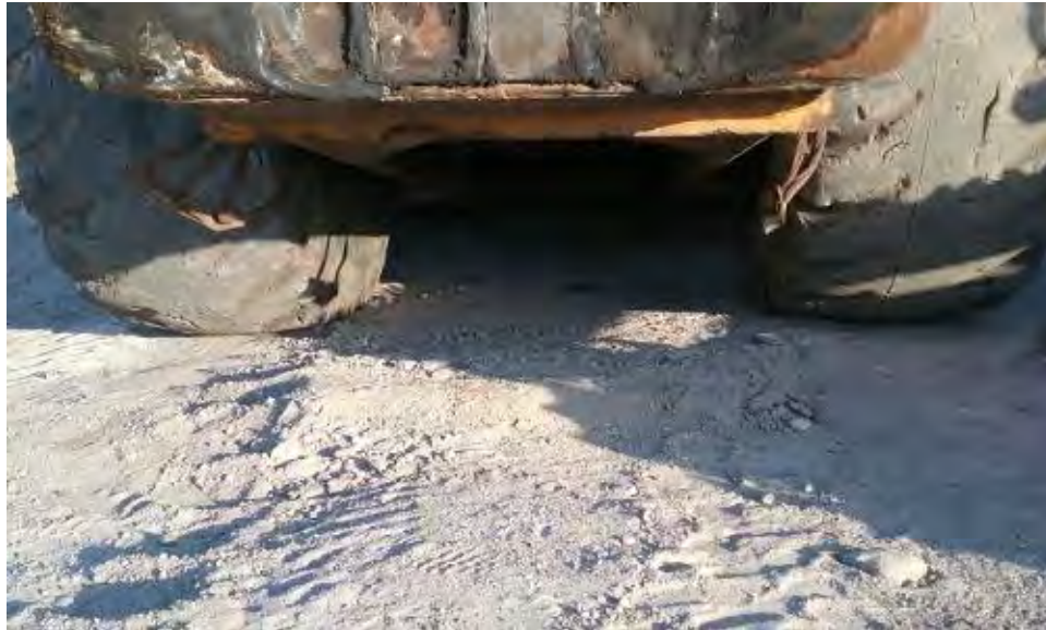
Caption Drips with no pan beneath W623 DG 9B56 Photo Attributes~ Capture Date/Time: Fri Aug 12 2016 07:28:42 GMT-0700 (MST) Coordinates: 32.619585, -116.94952 View Direction: East
