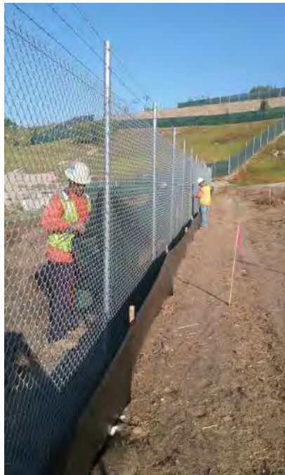
Caption Fence installation on south side.
