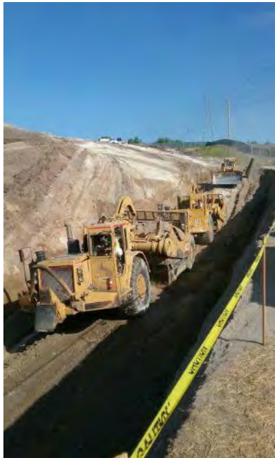
Caption Excavating keyway on north part of site.
