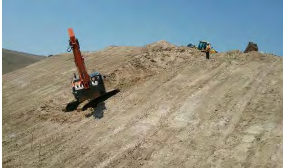
Caption Digging trench for drain in NE part of site.
