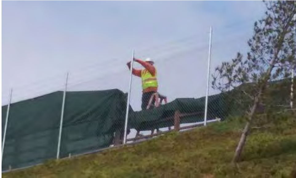
Caption Screen being installed on fencing on west edge of site.
