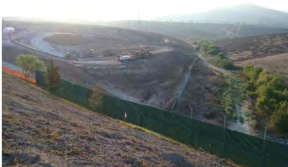
Caption Site overview at start of day.
