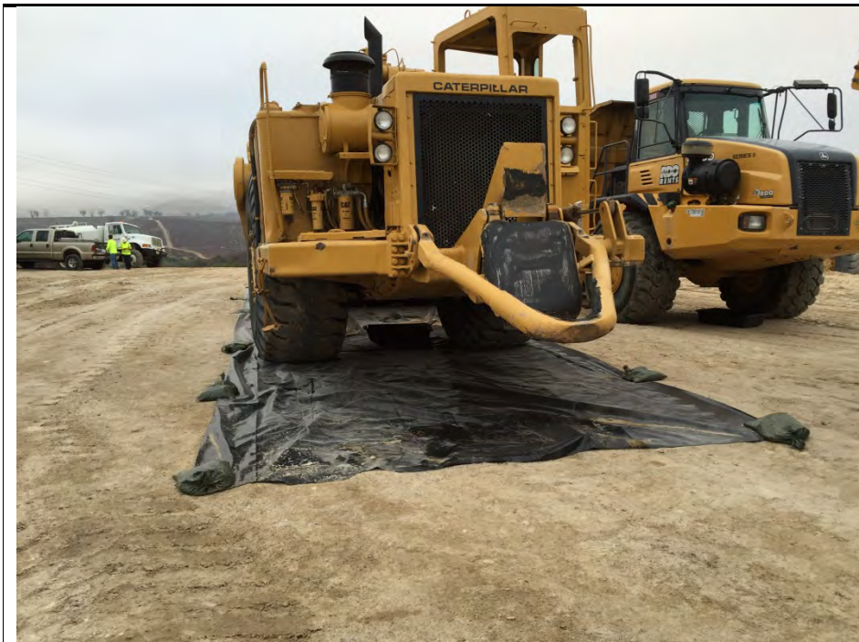
Photograph 4: Additional leak protection was added beneath the scrapers on August 19, 2016.
