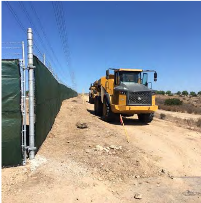
Caption Dump trucks accessing site
