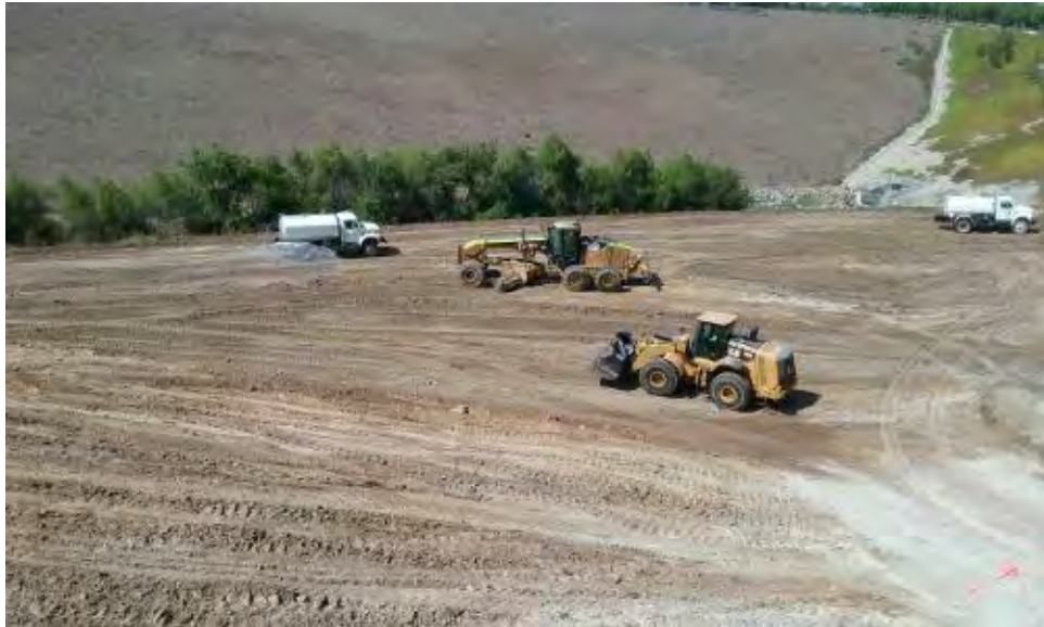
Caption Mixing and compacting fill dirt on southern part of site.
