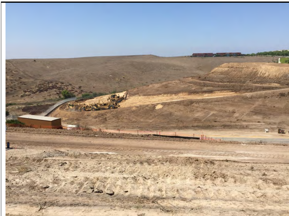
Photograph 2: Cut and fill activities on August 4, 2016.
