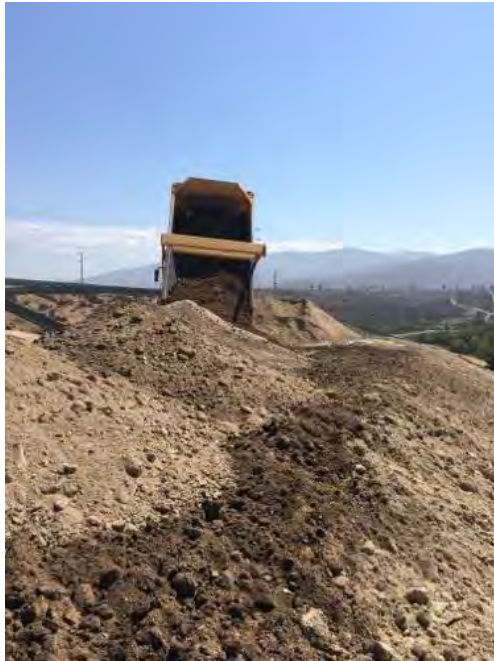
Caption Fill being dumped on western pad
