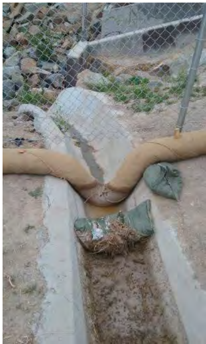
Caption Erosion control BMPs effectively capture runoff.
