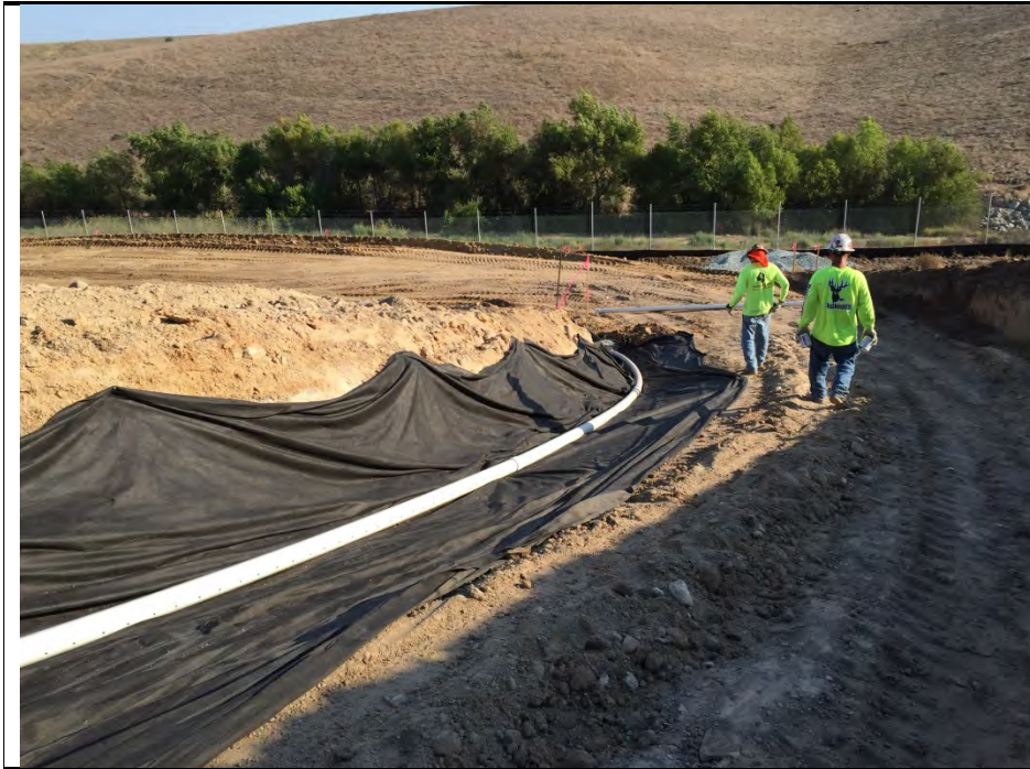
Photograph 1: Installation of perforated drainage pipeline on Monday August 3, 2016.
