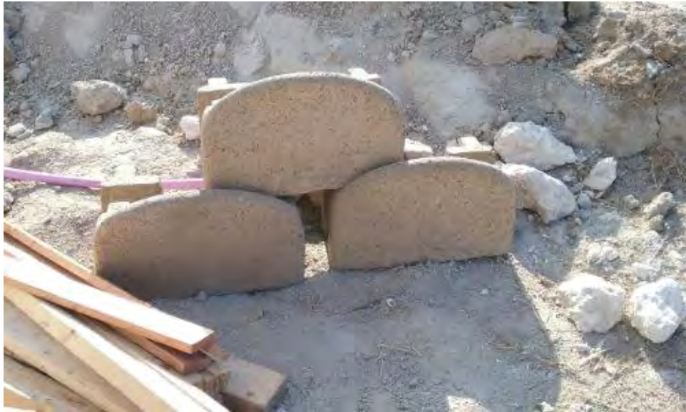
Caption Buff-colored blocks for Verdura retaining wall.
