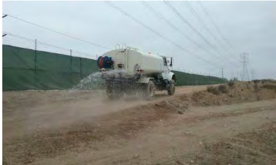
Caption Dust control on exterior access road.
