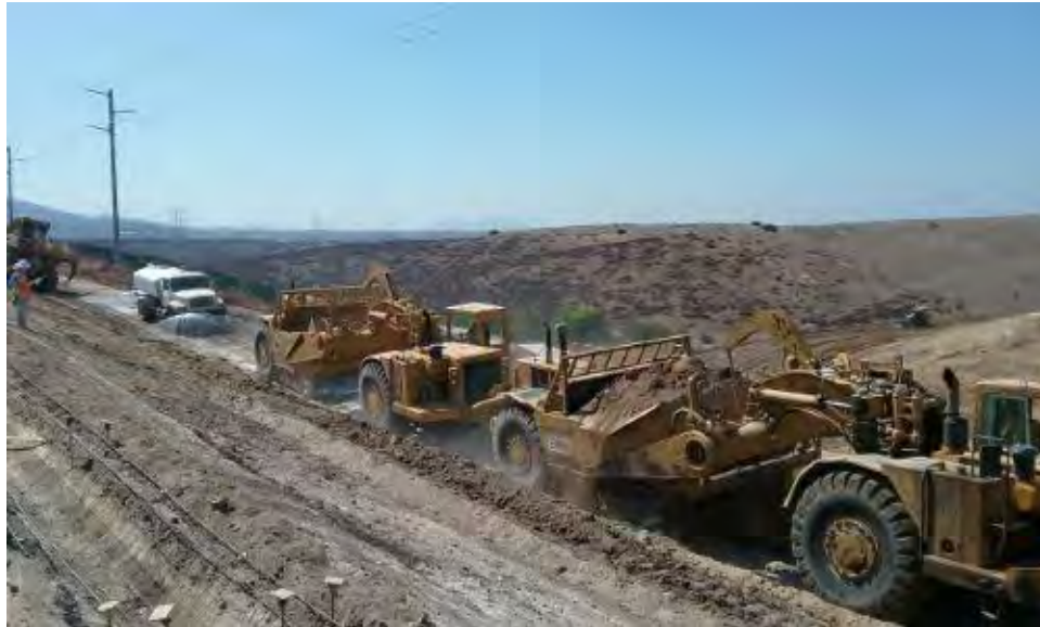
Caption Grading for new access road.
