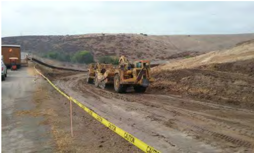
Caption D9s excavating keyway on north part of site.
