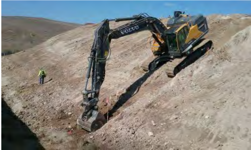
Caption Trenching for drain pipe in northeast corner.
