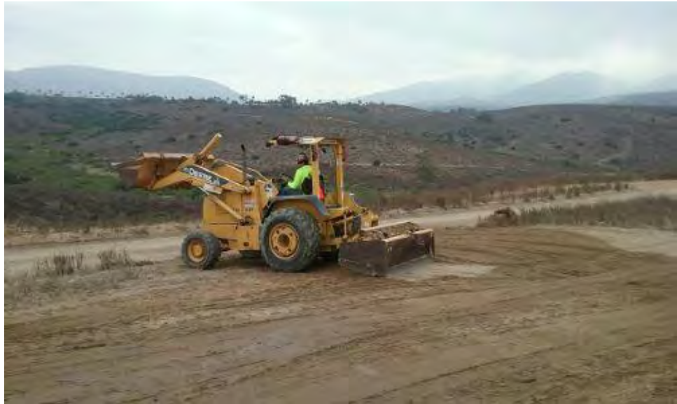
Caption Dozer clearing crossover (MPR3) outside north gate.
