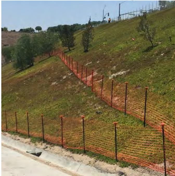
Caption Orange fencing marking limits of disturbance
