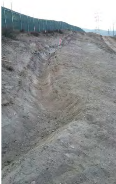
Caption Low point along brow ditch along north edge of site would allow wildlife egress.
