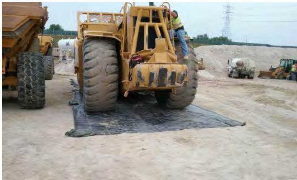
Caption Visqueen sheet beneath inactive equipment.
