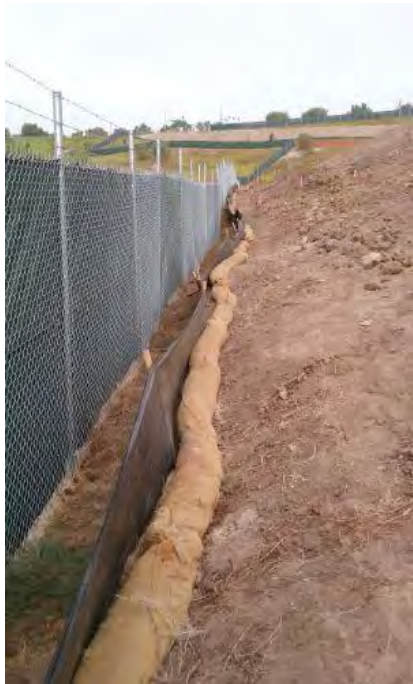
Caption Silt fence reinforced with straw wattles along southeast edge.
