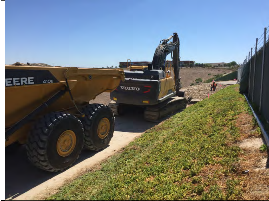
Photograph 3: Removal of the asphalt access road began on August 18, 2016.
