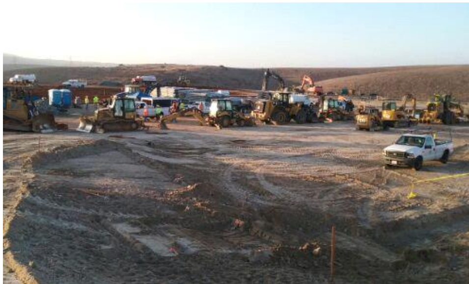
Caption Staging area / construction yard.
