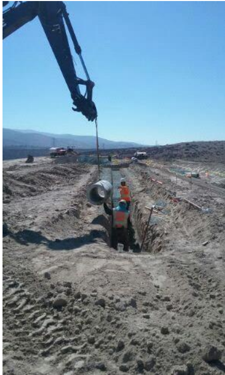
Crew installing drainpipe.
