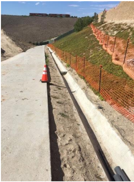
Caption Brow ditch with sand bags
