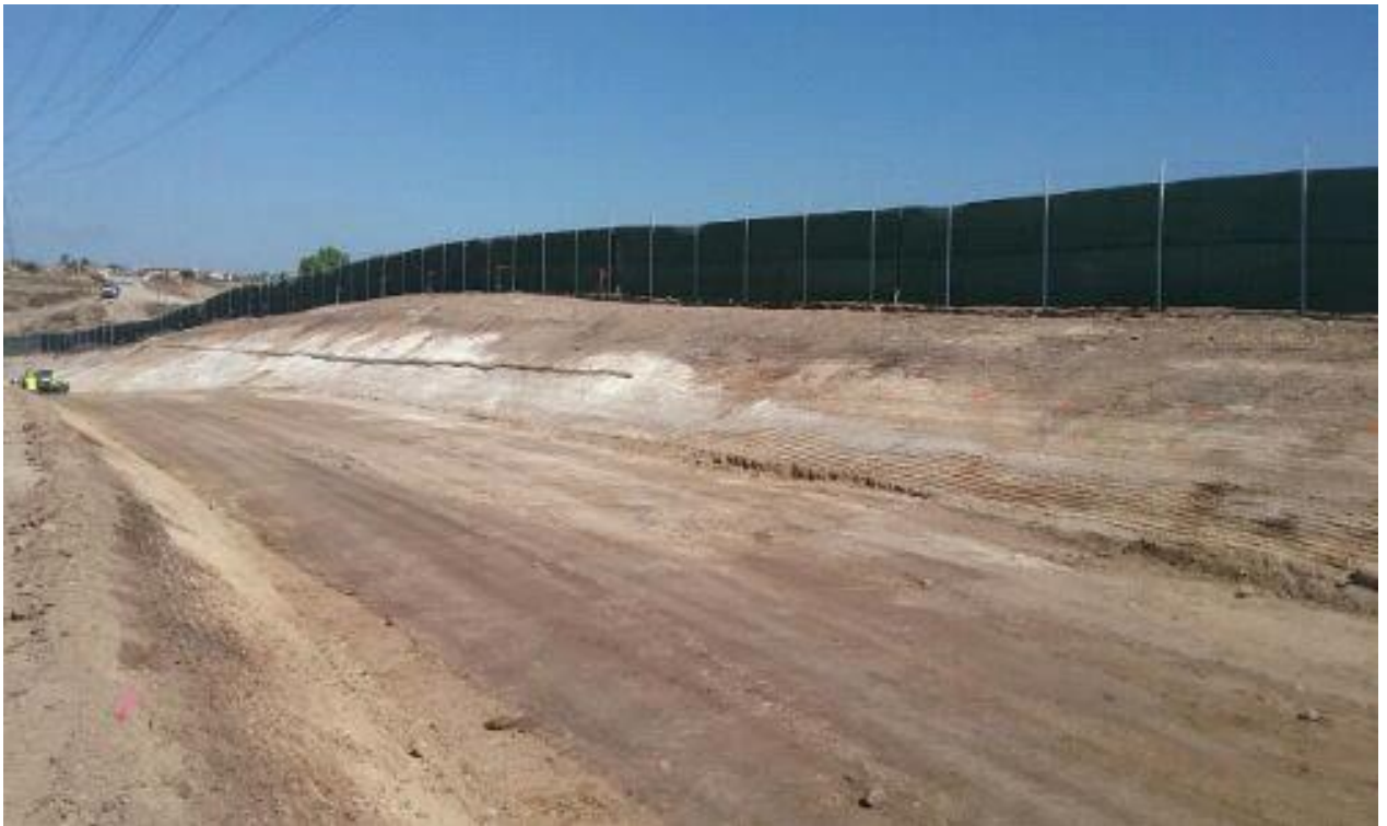
Caption Silt Fence being installed on north part of site.
