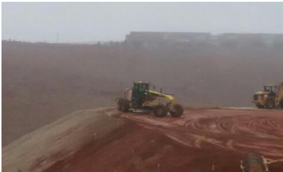
Caption Slope grading.
