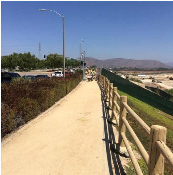
Caption Fencing work at northwest corner of project site
