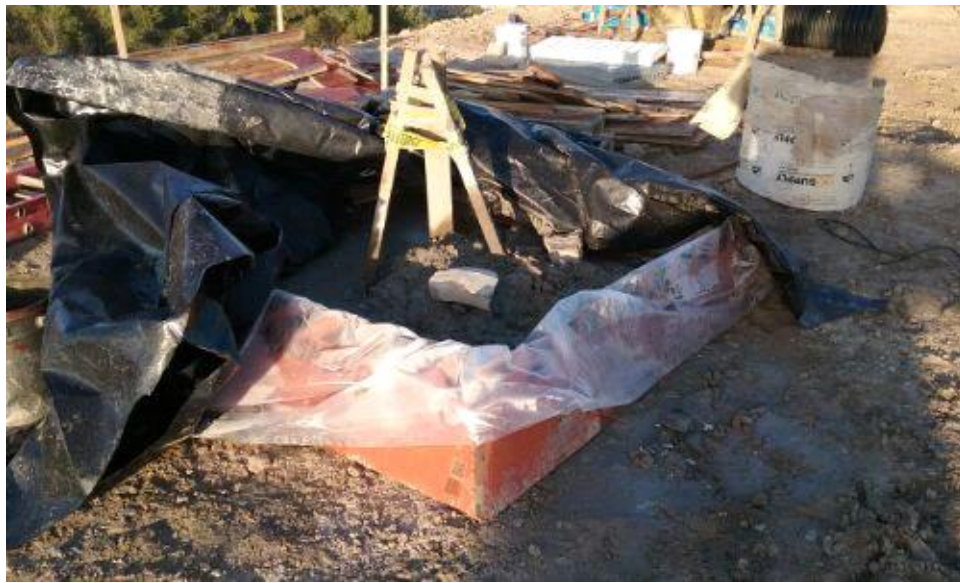
Caption Concrete washout basin.
