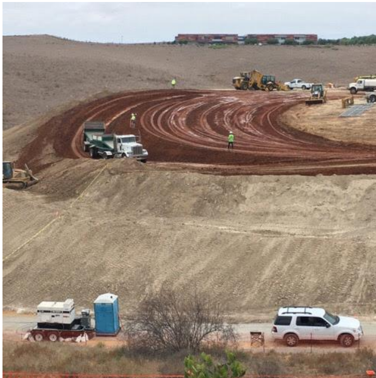
Caption Fill and grading
