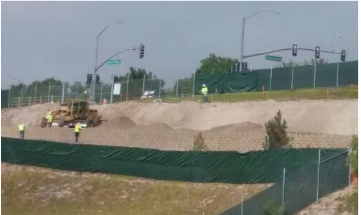
Caption Verdura wall being installed.
