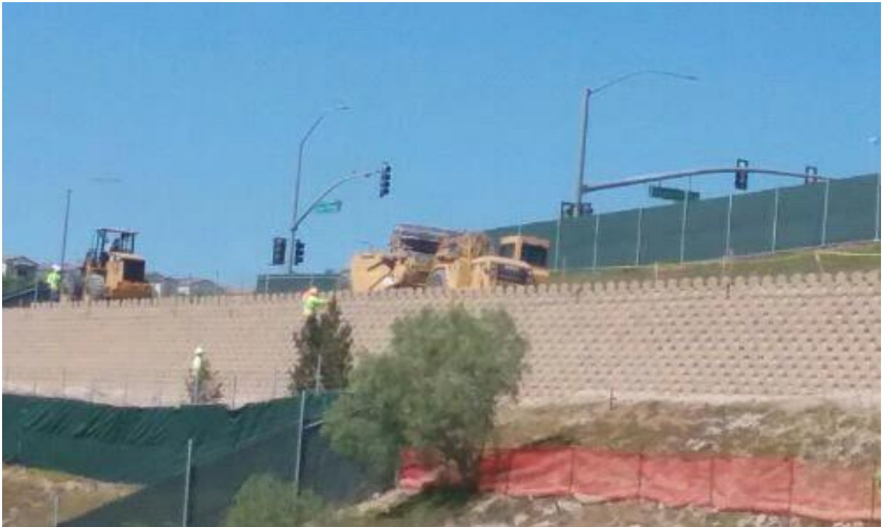
Verdura wall construction below west access road.
