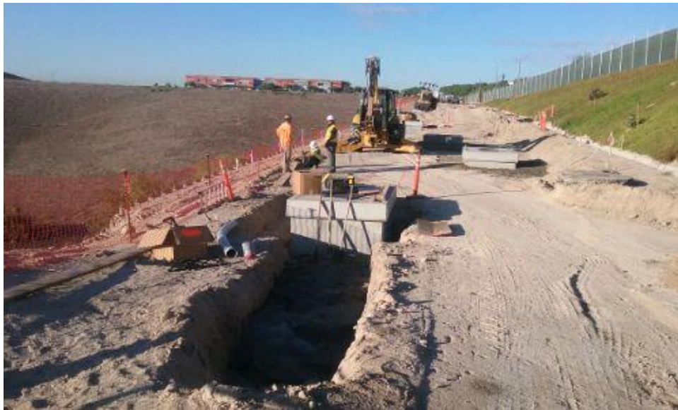
Caption Work on box for conduits in entrance road.
