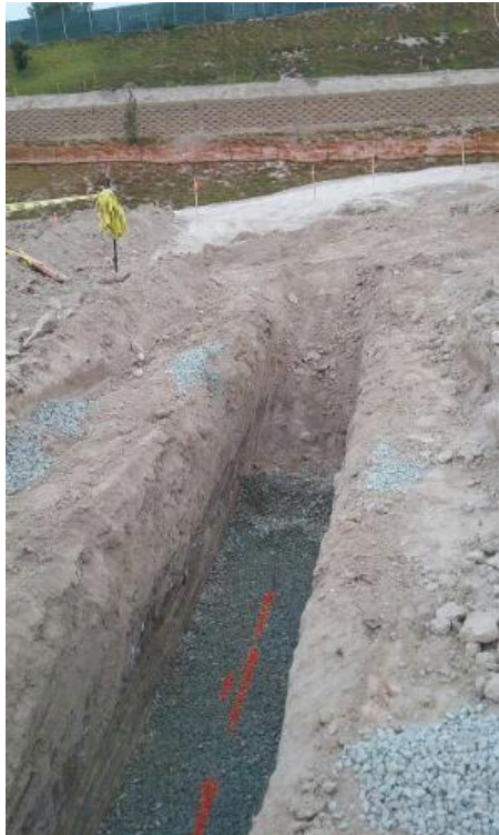
Caption Small animal exit ramp in trench for drainpipe.
