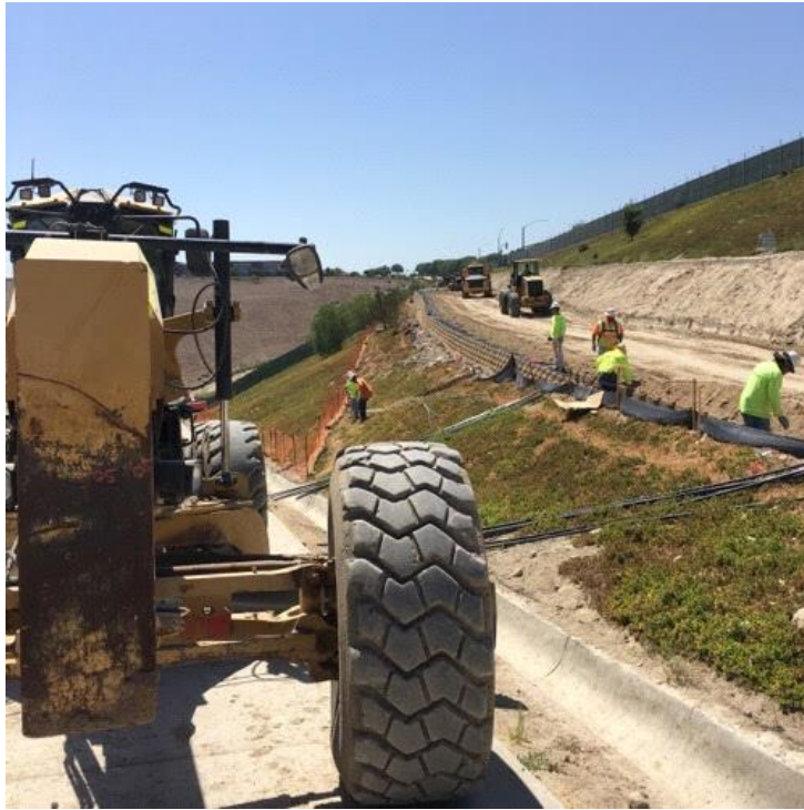
Caption Retaining wall construction
