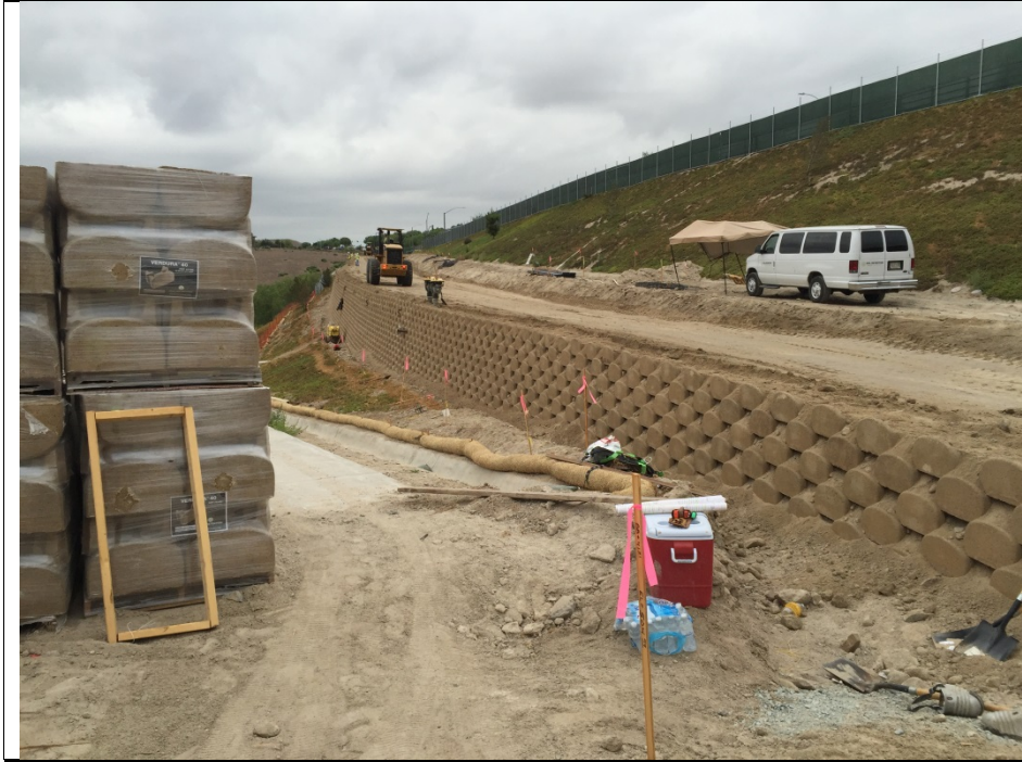
Photograph 3: Construction of the Verdura wall occurred during the week of September 12, 2016.
