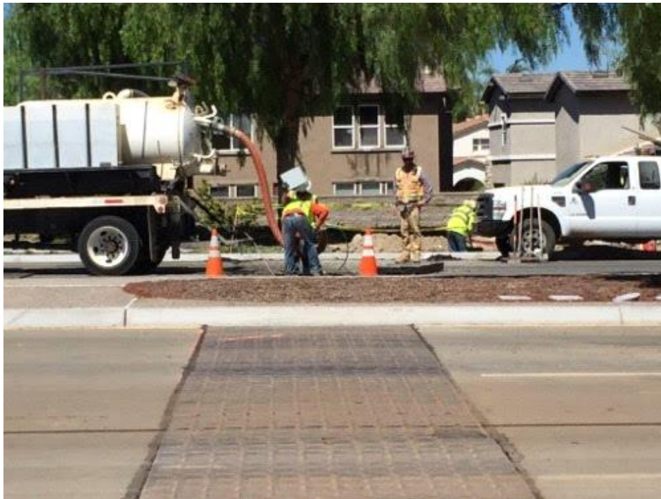
Caption Trenching on Hunte Parkway for temporary power line
