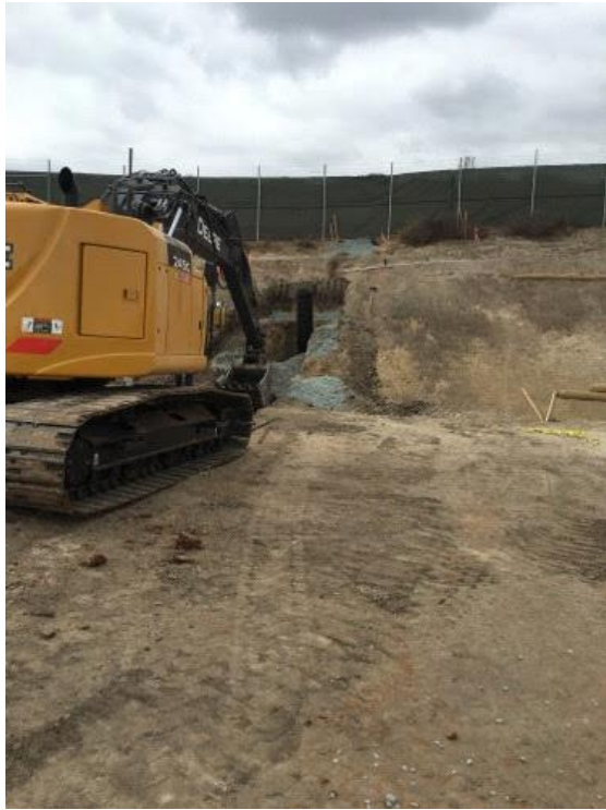
Caption Storm drain install
