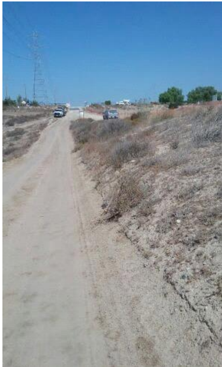
Caption North access road.
