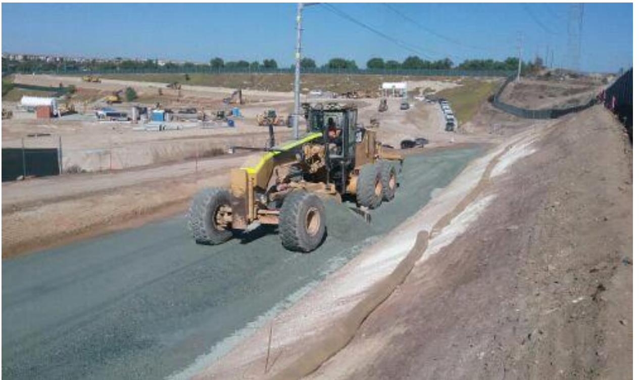
North access road grading.
