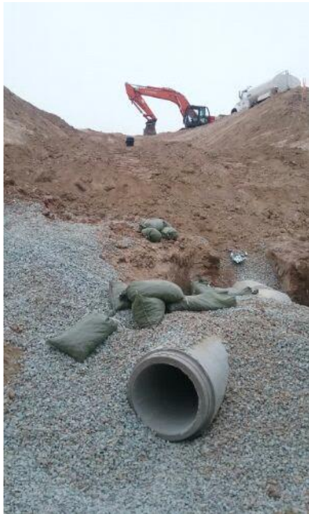
Caption Storm drain in NE part of site.
