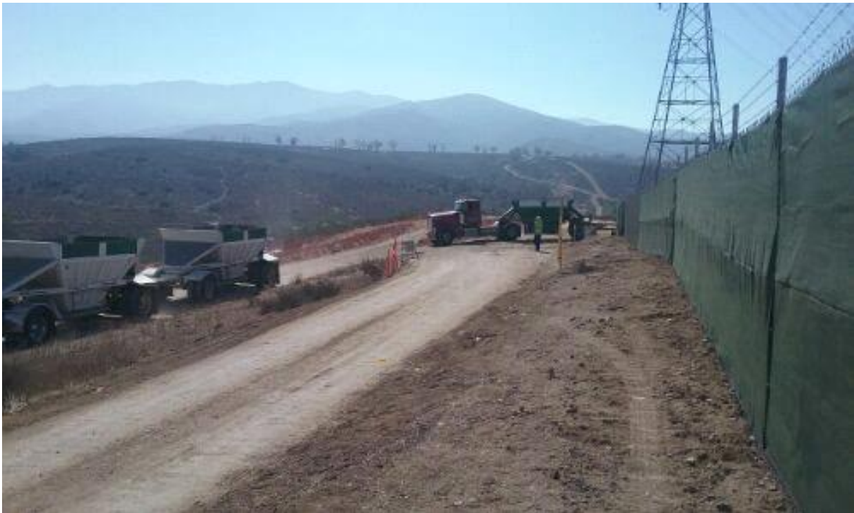
Caption Worker directing gravel truck traffic into / out of site.
