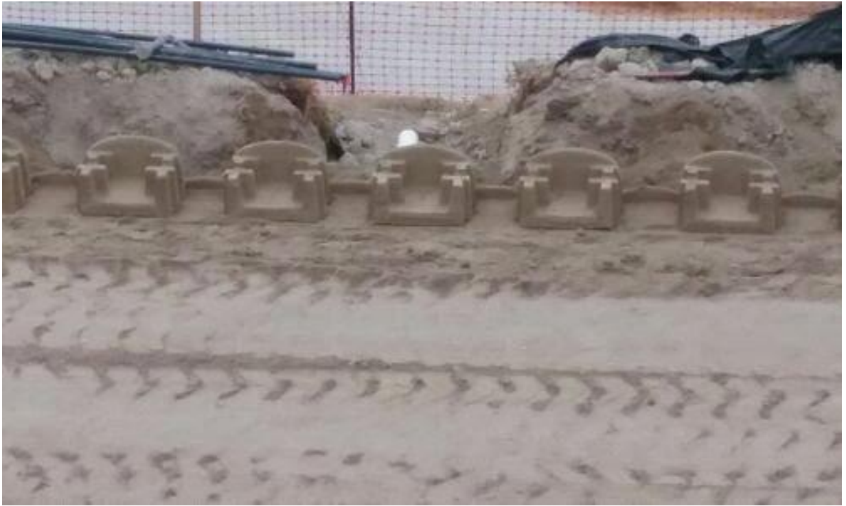
Caption Blocks for retaining wall.
