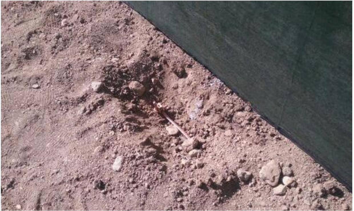
Caption Grounding wire installed along north fence.
