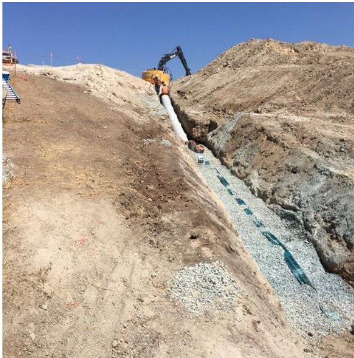
Caption Storm drain installation
