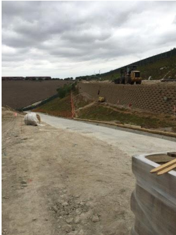
Caption Retaining wall close-up
