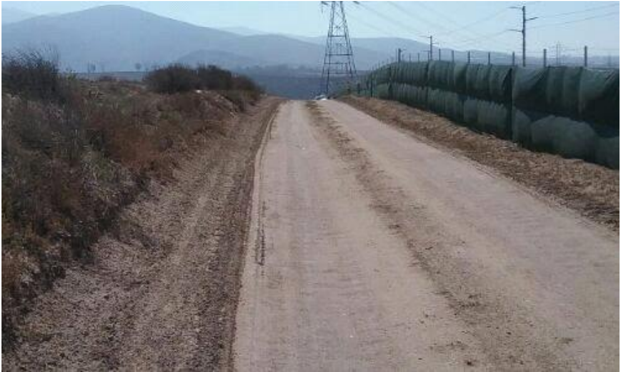
Caption North access road.
