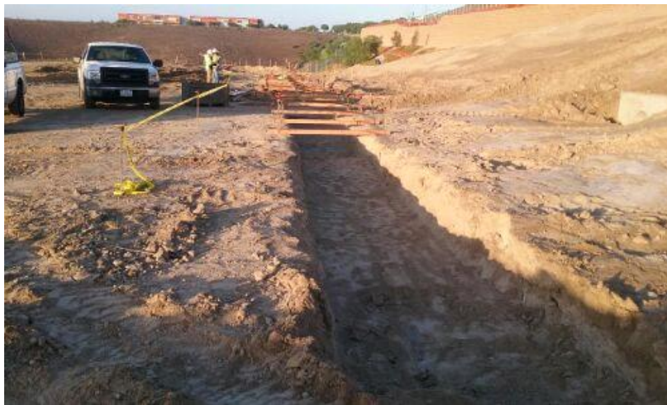
Caption Trench for screening wall.
