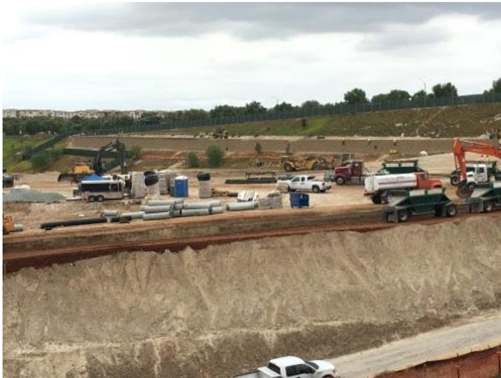
Caption Retaining wall
