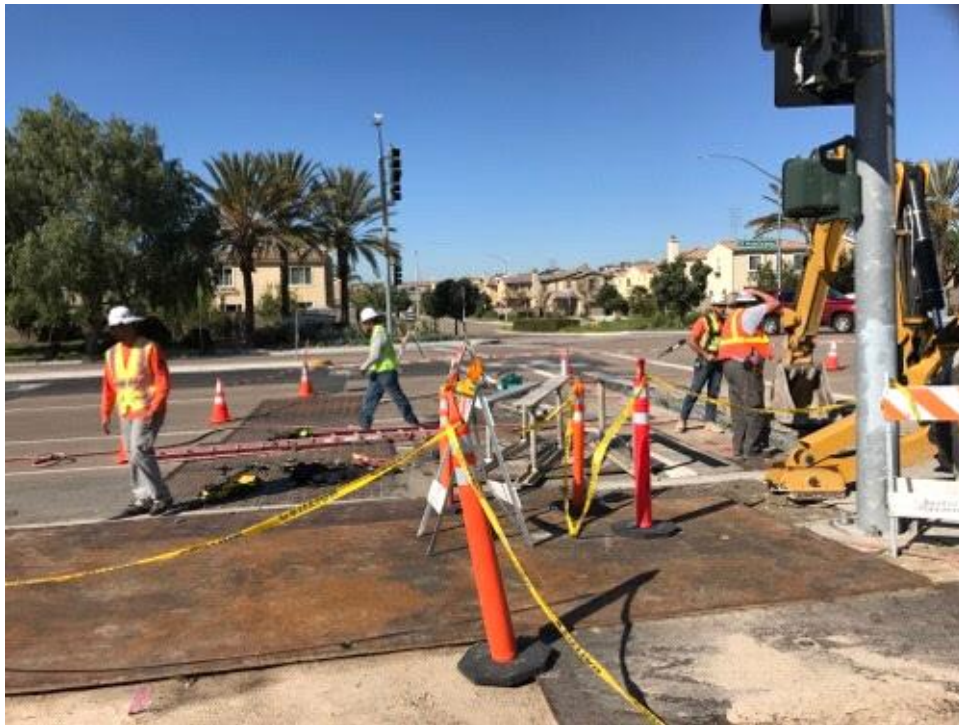
Caption Trenching on Hunte Parkway.
