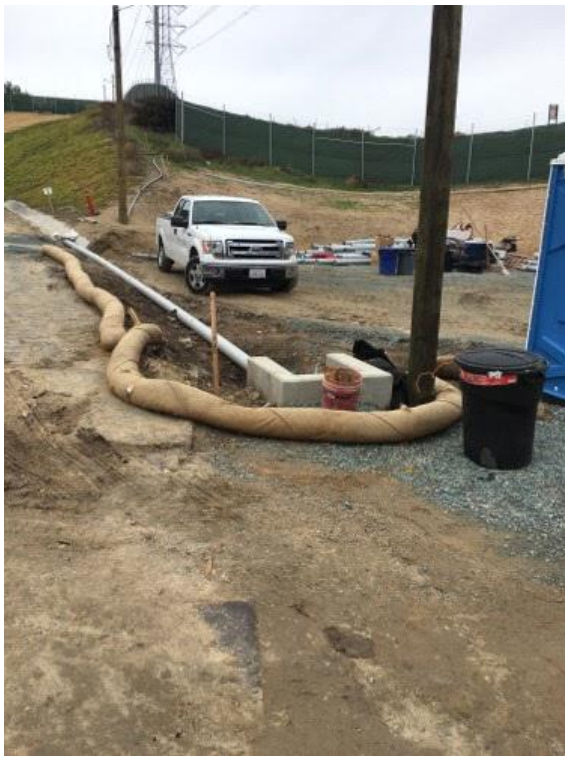
Caption Trench work complete
