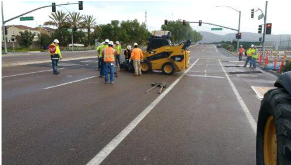
Caption Grinding pavement in Hunte Parkway for conduit trenches
