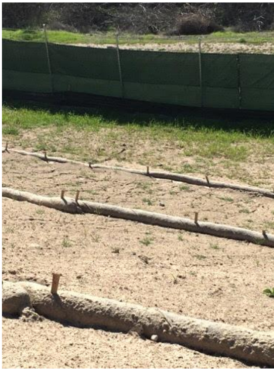
Caption Lower fiber roll on western slope needs maintenance
