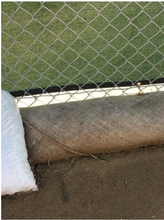
Caption BMPS along fence line actively filtering sediment. No sediment offsite at this area.
