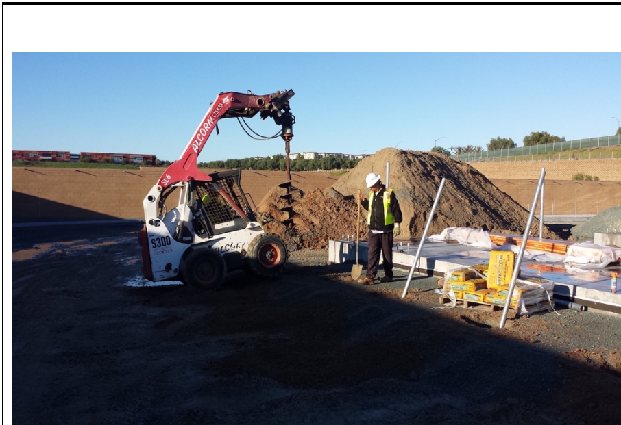
Photograph 2: Substation equipment pad fence installation occurred during the week of January 28, 2017.
