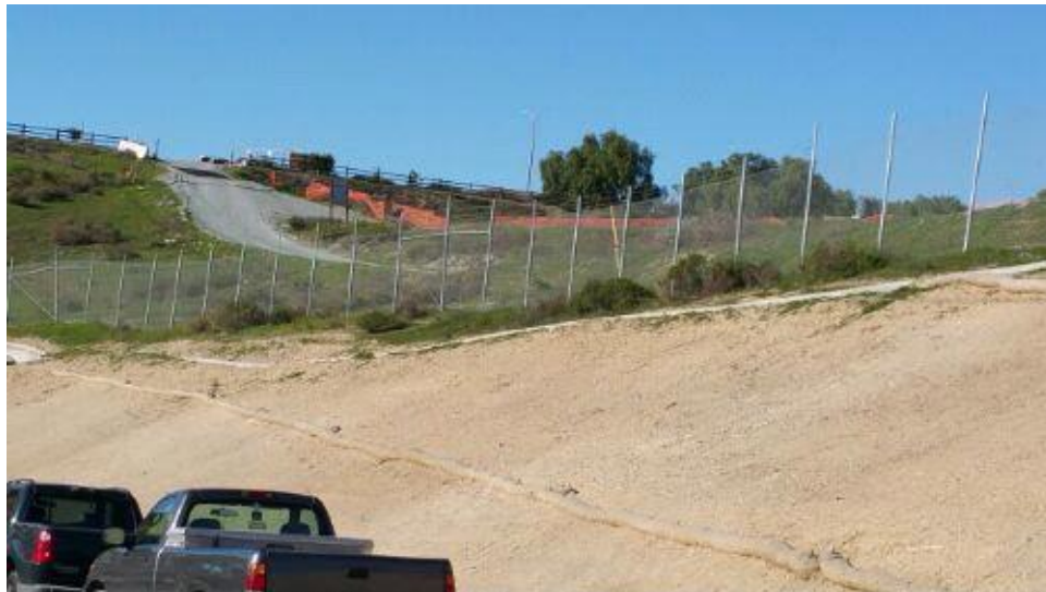
Caption Screening fence along east access road has been removed after wind caused damage to chain link fence.
