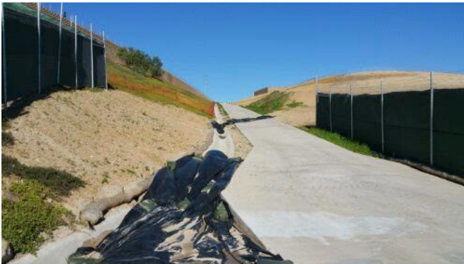
Caption Main brow ditch has been cleared of sediment.
