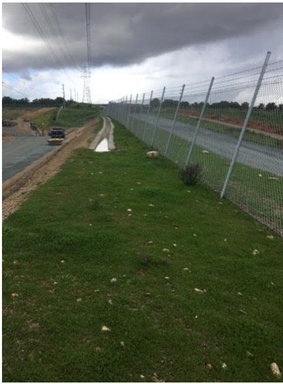
Perimeter fence without green screening
