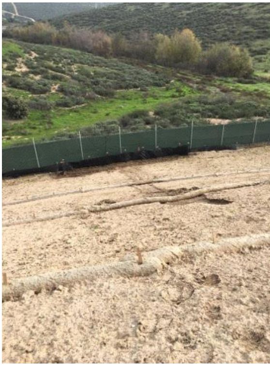
Caption New silt fence downslope of erosion area
