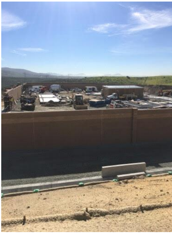
Caption Internal site overview
