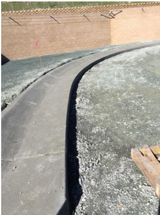
Caption New curb and gutter inside the substation pad area.
