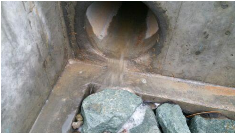
Caption Water flowing off-site from Line B (south side) appears to be within acceptable opacity.
