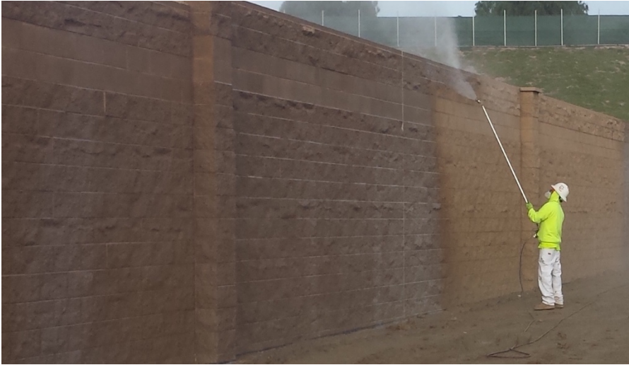
Photograph 1: Substation masonry wall water-proofing occurred during the week of January 21, 2017.
