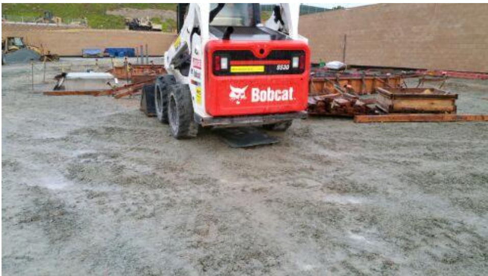
Caption Drip pan in place.
