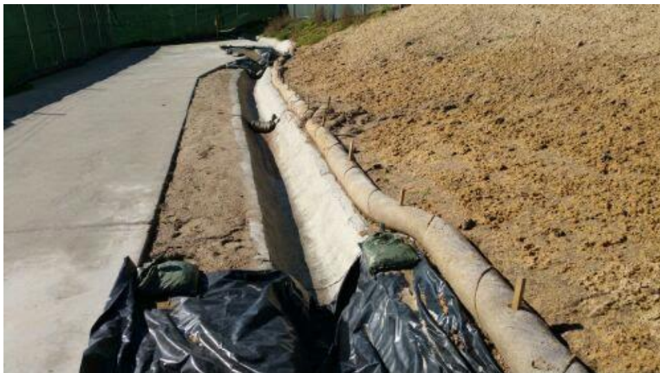
Caption Gravel bag check dams captured sediment in main brow ditch.
