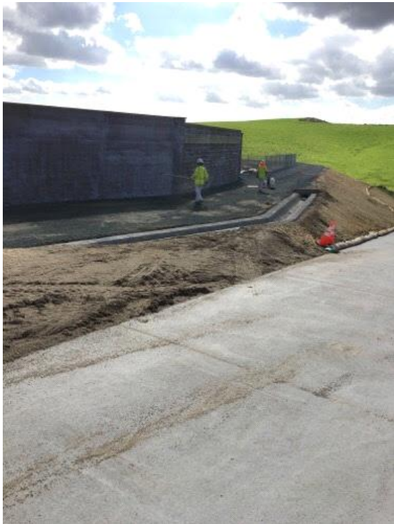
Caption Sealant being applied to walls
