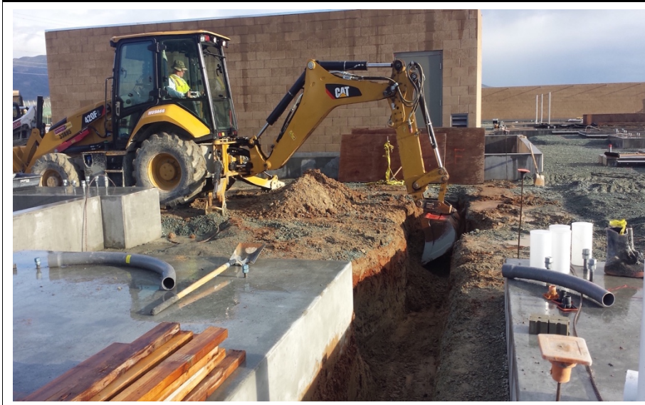
Photograph 1: Trenching for substation 69kV conduit occurred the week of January 28, 2017.
