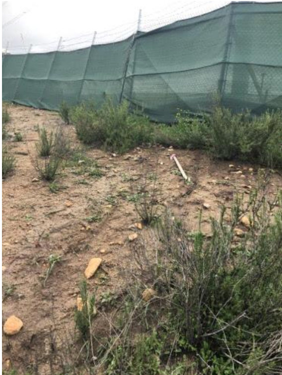
Caption Offsite runoff and erosion
