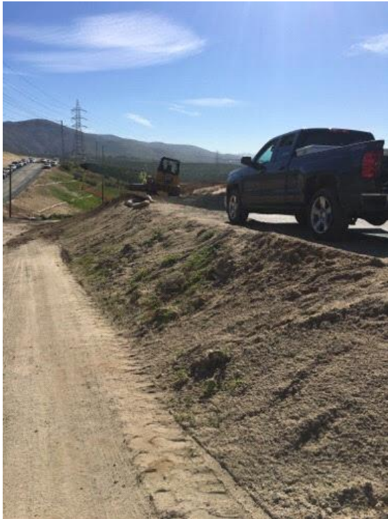
Caption Final pad grading
