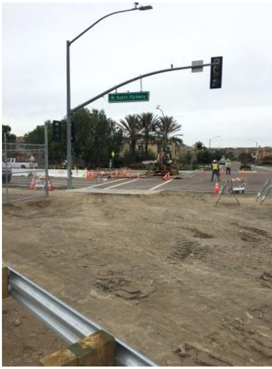
Caption Trench work in Hunte Parkway
