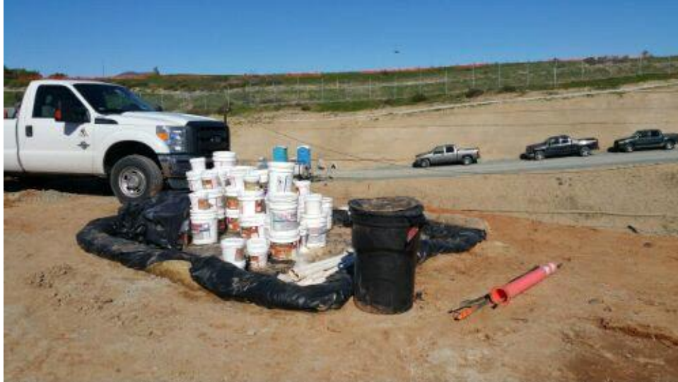
Caption Secondary containment of hazardous materials: anti-graffiti paint.
