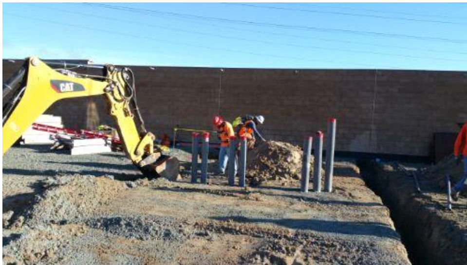
Caption Paleontological monitor inspecting excavated soil.
