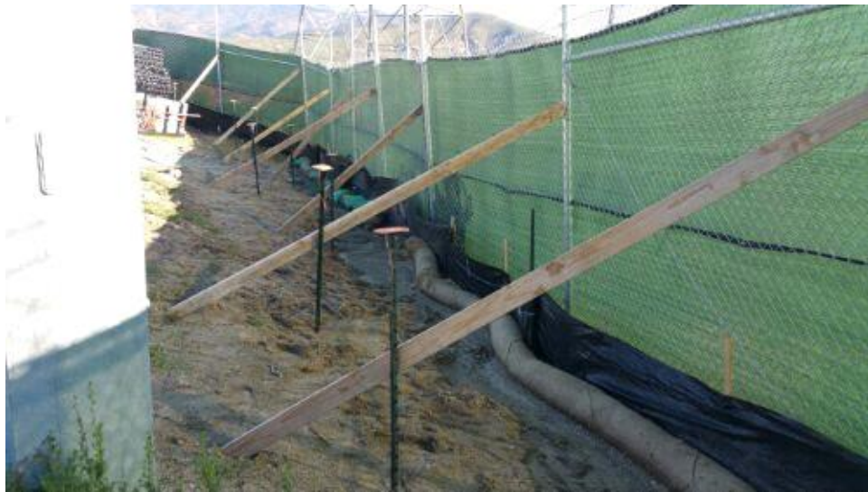
Caption Repairs to erosion control BMPS and fence near east entrance.
