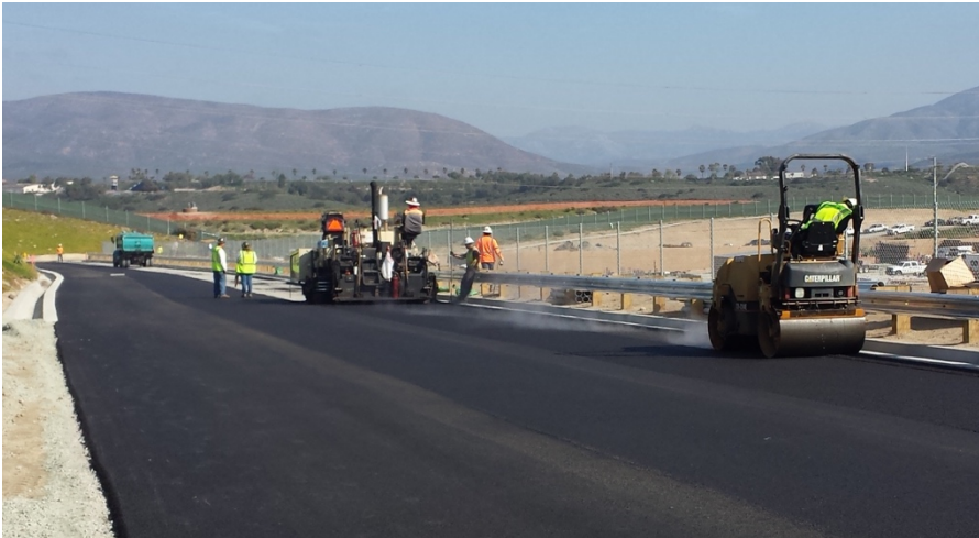
Photograph 2: Paving of Road A occurred during the week of January 21, 2017.
