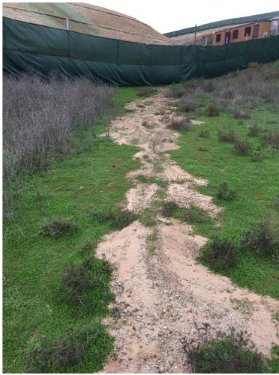
Caption Offsite erosion area, previously reported. Area of siltation grew by about 10-12 feet since original photo was taken.
