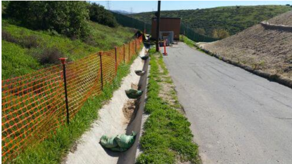
Caption Brow ditch near trailer has been cleared but for one wet area.
