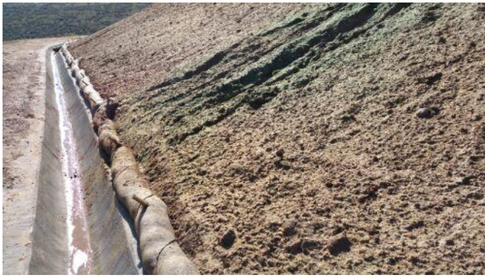
Caption Sediment removed from above straw wattle on east slope.
