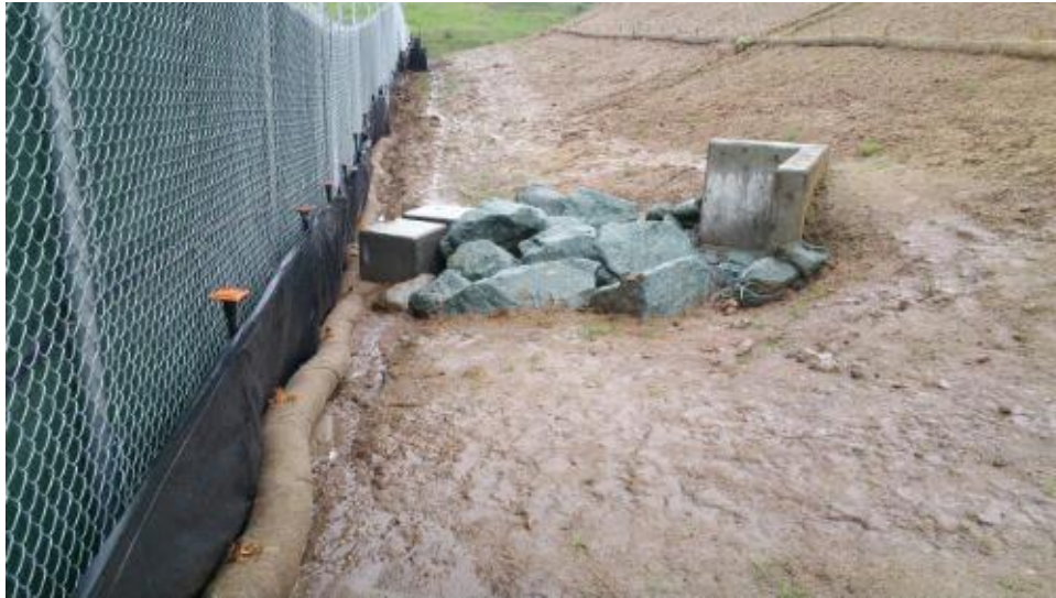
Caption BMPS near outfall on south side.
