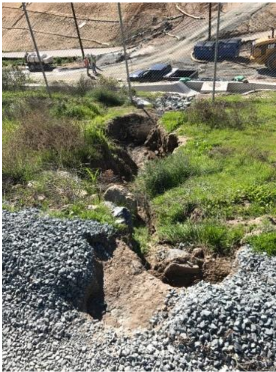
Caption Area where concrete spillway will be constructed in MPR #7
