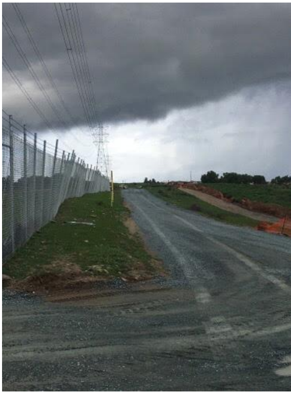
Caption Access road with safety/traffic control stationed at Hunte Parkway.
