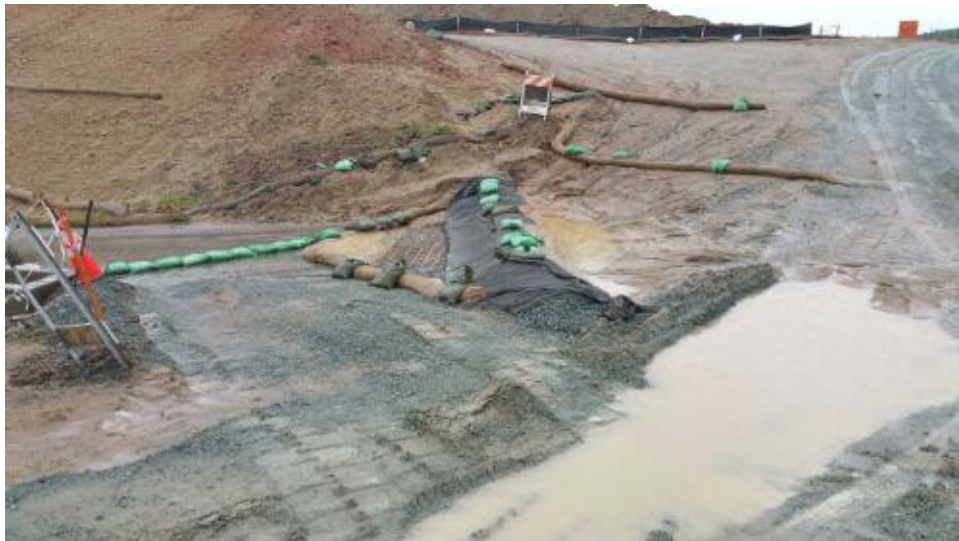
Caption BMP below largest disturbed area captured most sediment.
