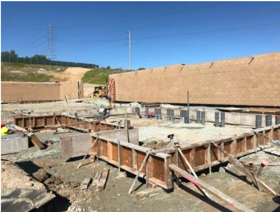
Caption Foundation work for substation switch gear pad.
