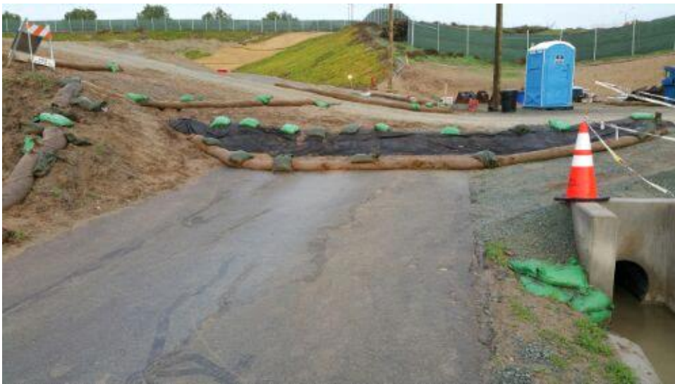
Caption Erosion control "burrito" with little sediment below it.
