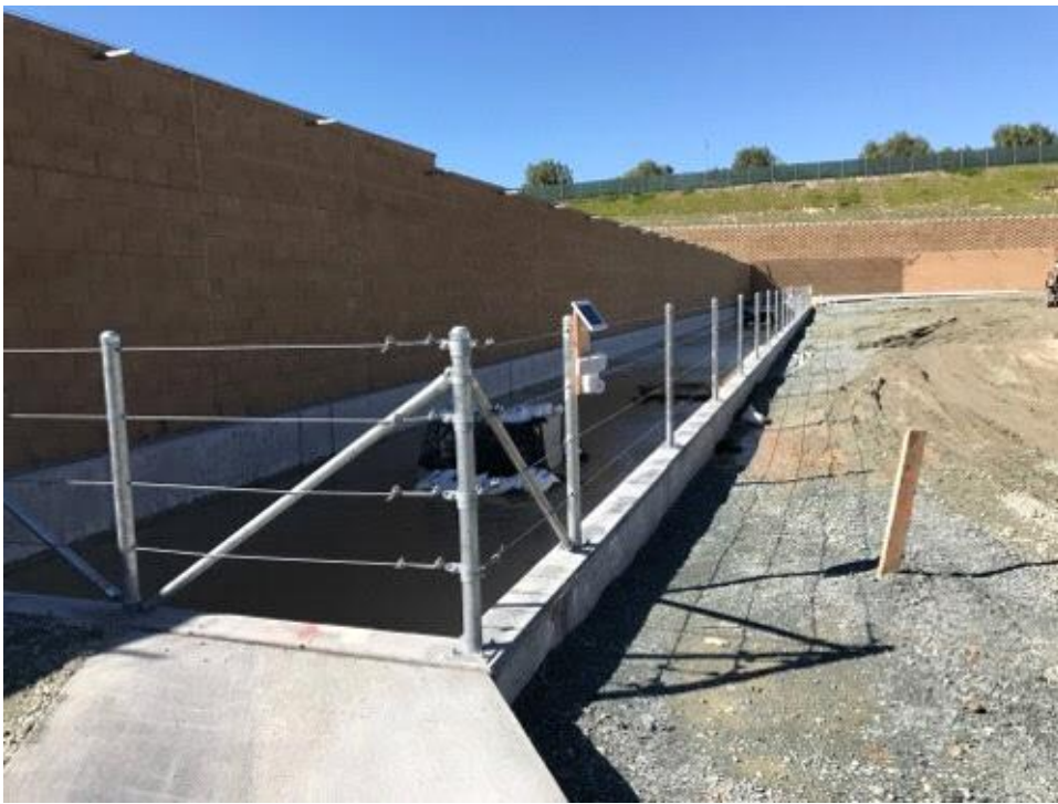
Caption Oil detention basin complete.
