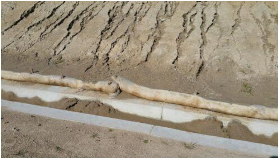
Caption Sediment buildup behind fiber rolls on west slope.
