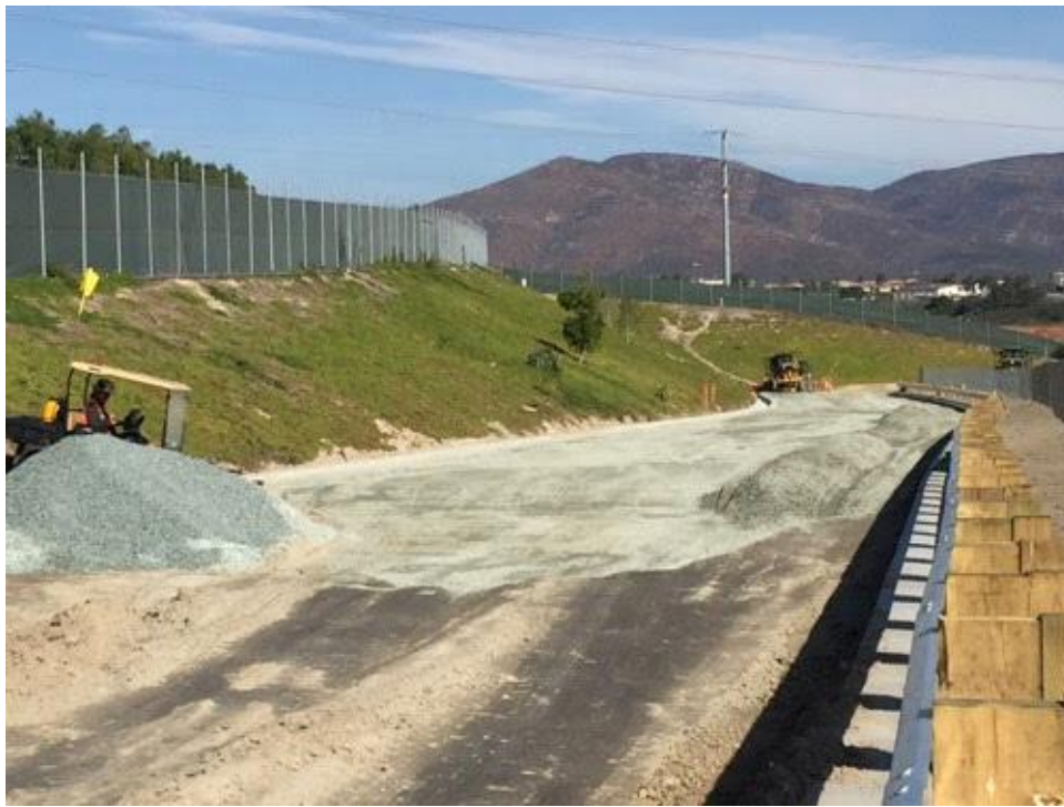
Caption Laying base rock on Access Road A.
