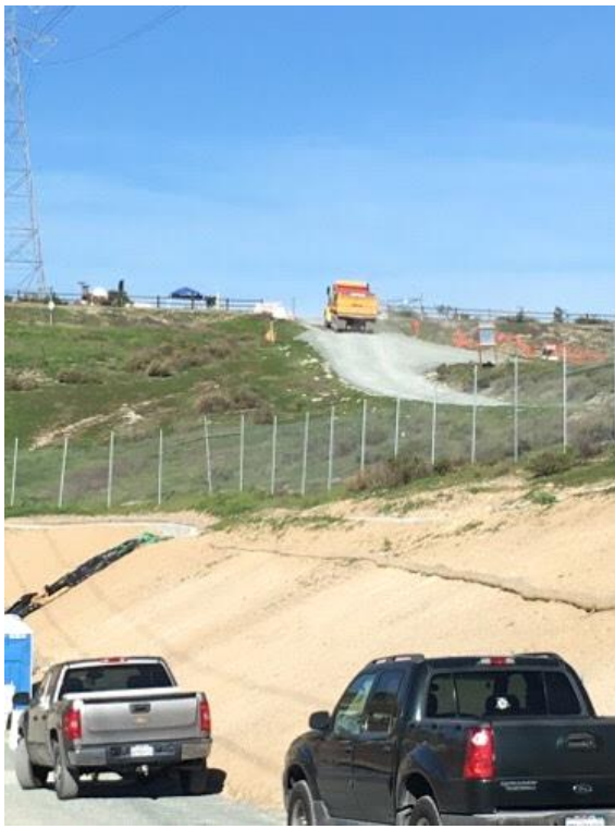
Caption Dump truck and safety flagger at Hunte Parkway.
