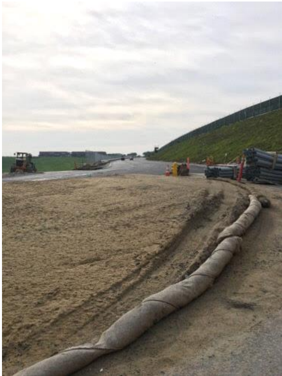
Caption Paved access road
