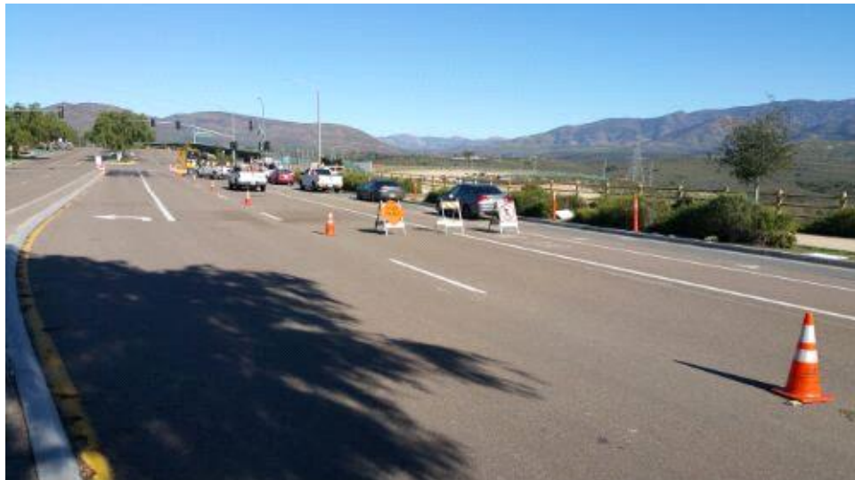
Caption Traffic controls in place during trenching in Hunte Parkway.
