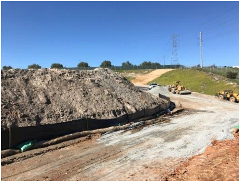
Caption Spoils from substation pad excavation with BMP protection.
