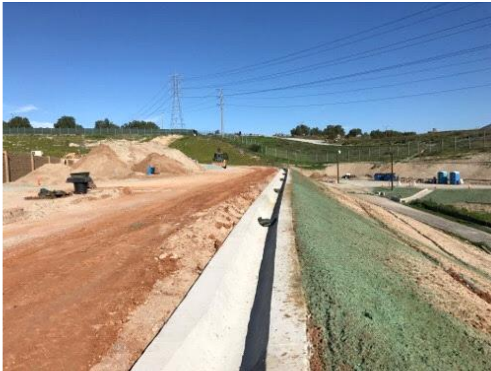
Caption New brow ditch along edge of substation pad.
