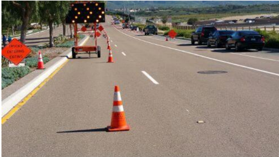
Caption Traffic controls for work on Hunte Parkway.
