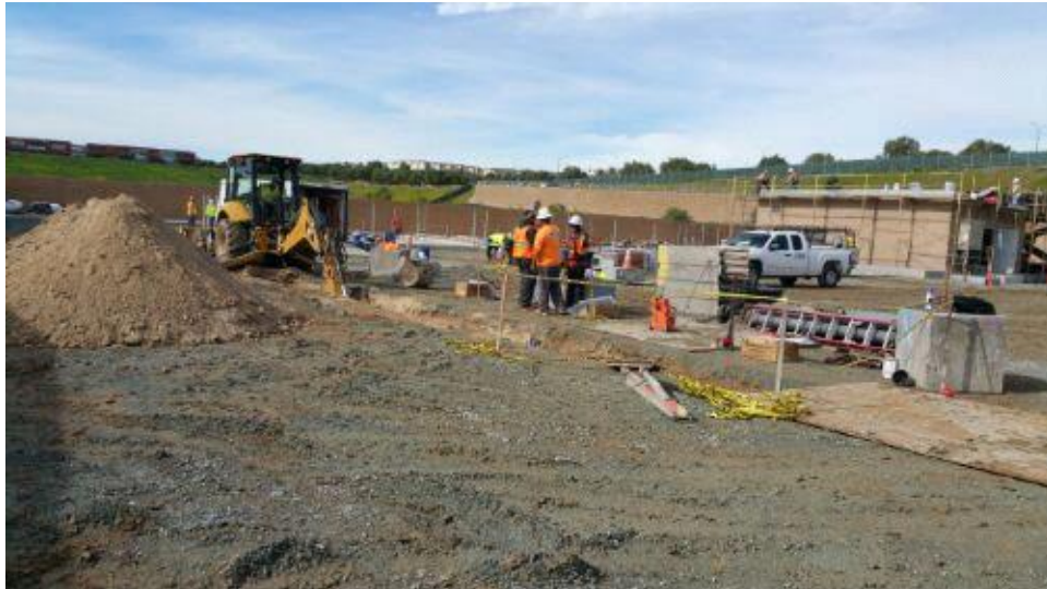
Caption Trenching for conduits within substation yard.
