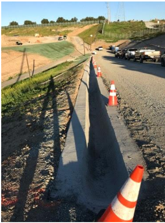
Caption New brow ditch along eastern access road.
