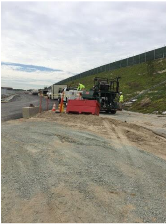
Caption Hydroseed BFM contractor
