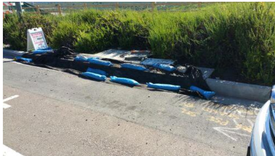
Caption Filter fabric at drain in Hunte Parkway to capture construction waste is removed prior to rains to avoid flooding road.
