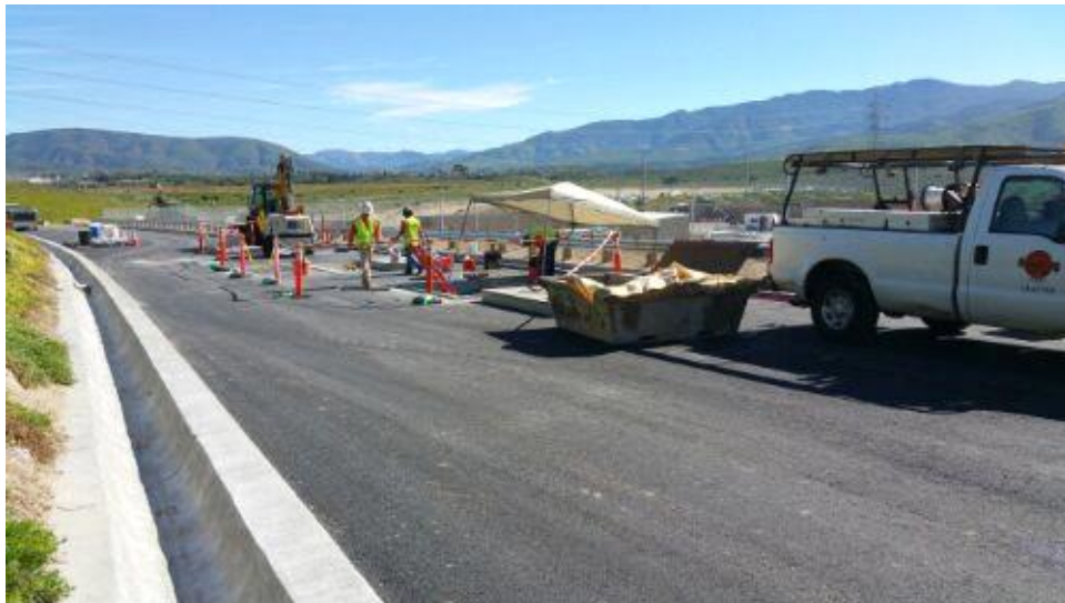
Caption Vault work in permanent Access Road A.
