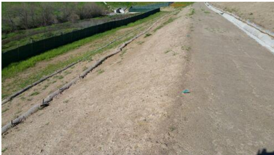
Caption Lower slope on west side.
