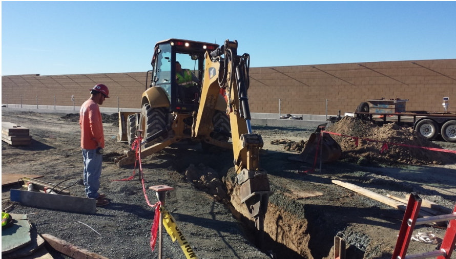
Photograph 1: Trenching for substation 69kV conduit occurred the week of February 4, 2017.
