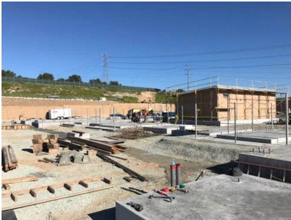
Caption Substation pads being constructed.
