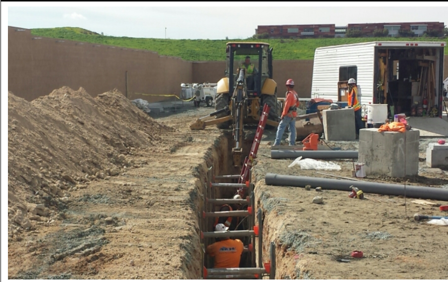
Photograph 1: Trenching for substation 69kV conduit occurred the week of February 10, 2017.
