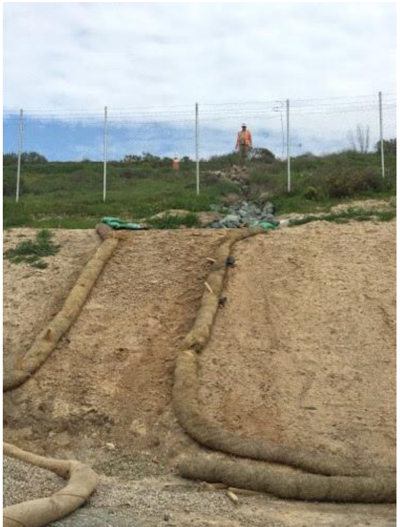
Caption Temporary riprap BMPs at MPR #7 location
