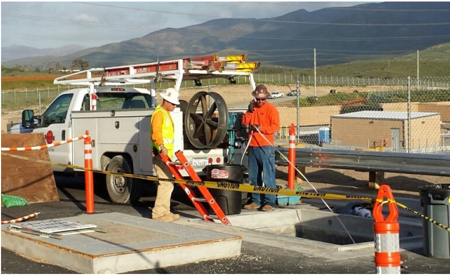
Photograph 1: Proofing 12kV conduit occurred the week of March 04, 2017.
