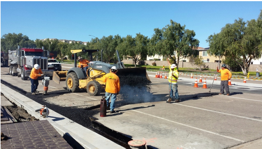
Photograph 2: Patching asphalt on Hunte Parkway occurred during the week of March 04, 2017.
