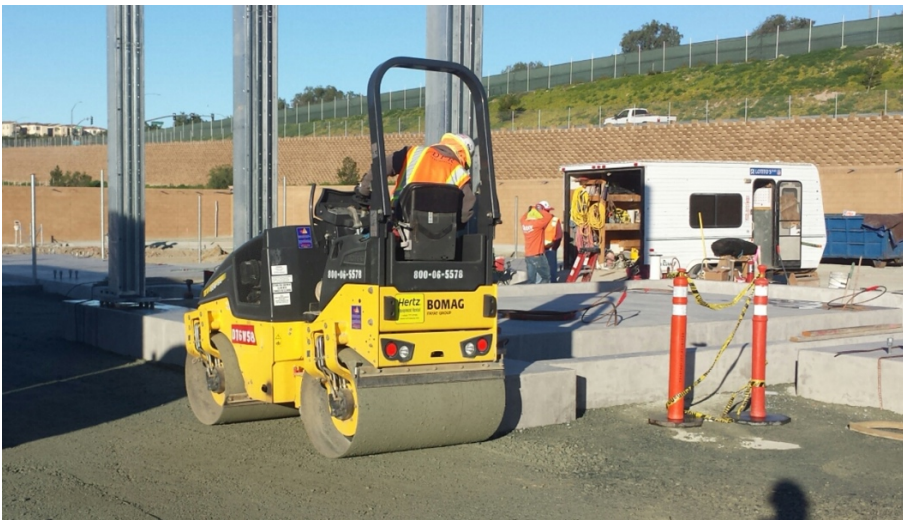
Photograph 2: Installing base within the substation occurred during the week of March 18, 2017.
