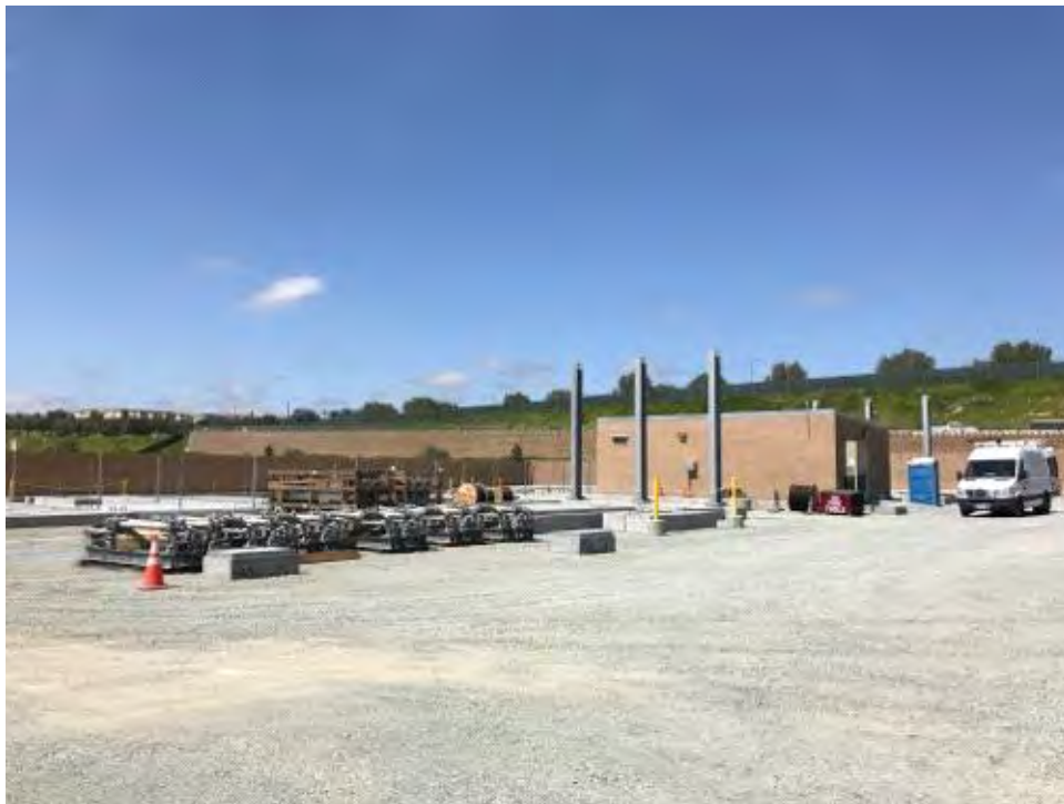
Caption Substation interior.
