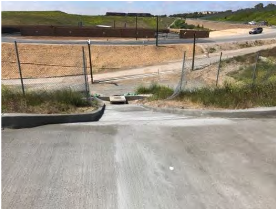
Caption MPR #7Spillway to catch basin
