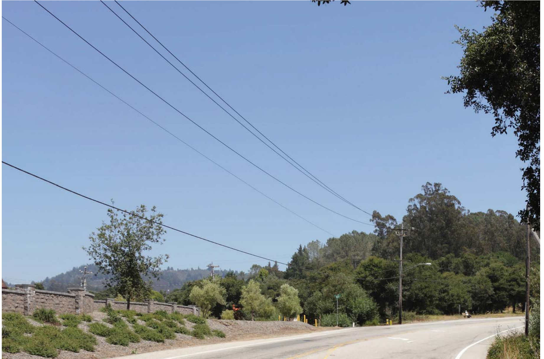
View from Freedom Boulevard near Rob Roy Substation looking north (VP 21)
