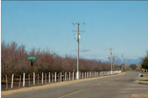
Photo #11: View looking north from N. Sunnyside Avenue near the intersection with Lexington to substation site. Date of photograph: January 11, 2011.
