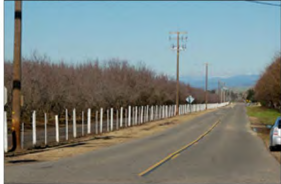
Photo #12: View looking north from intersection of N. Sunnyside Avenue with E. Shepherd Avenue to substation site. Date of photograph: January 11, 2011.
