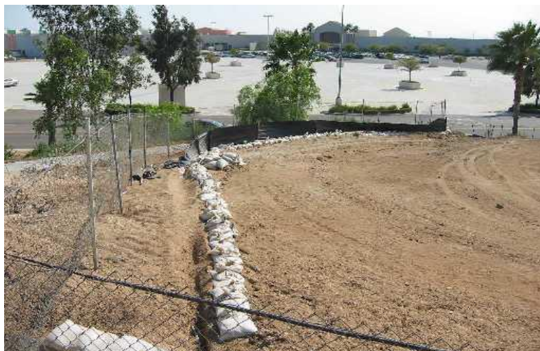
Gravel bags used as perimeter control.
