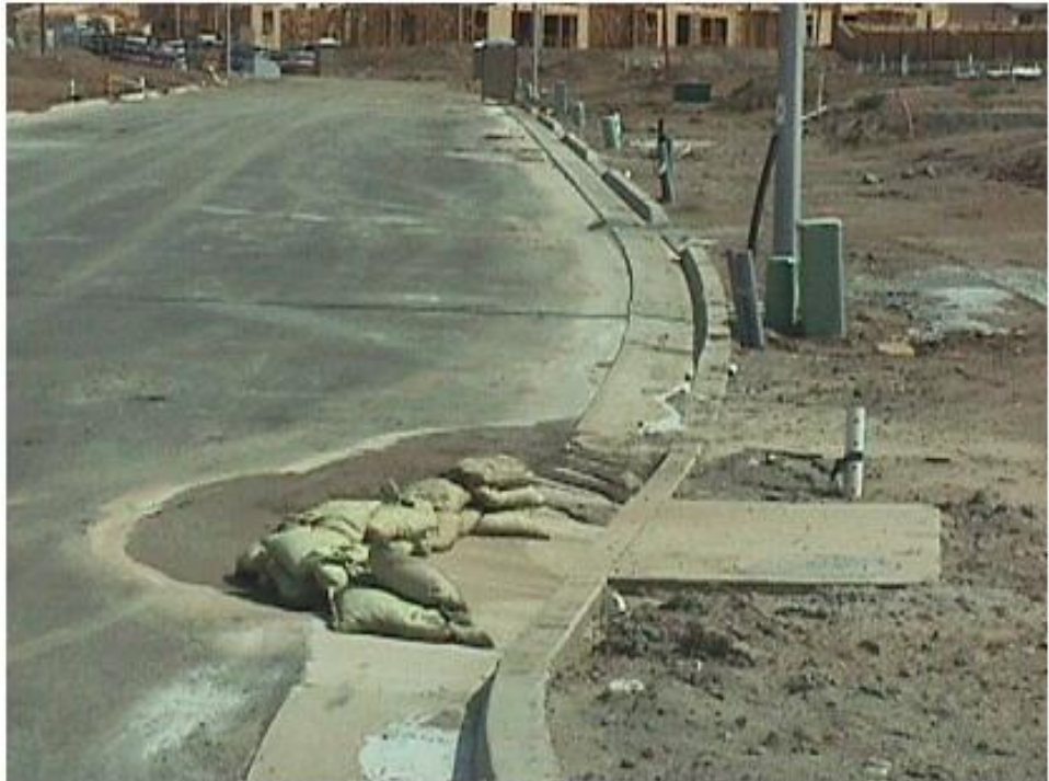
Gravel bag inlet protection.
