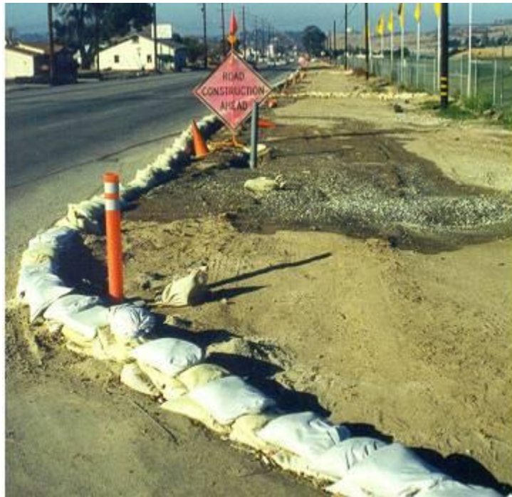
Sand bags used as perimeter control.
