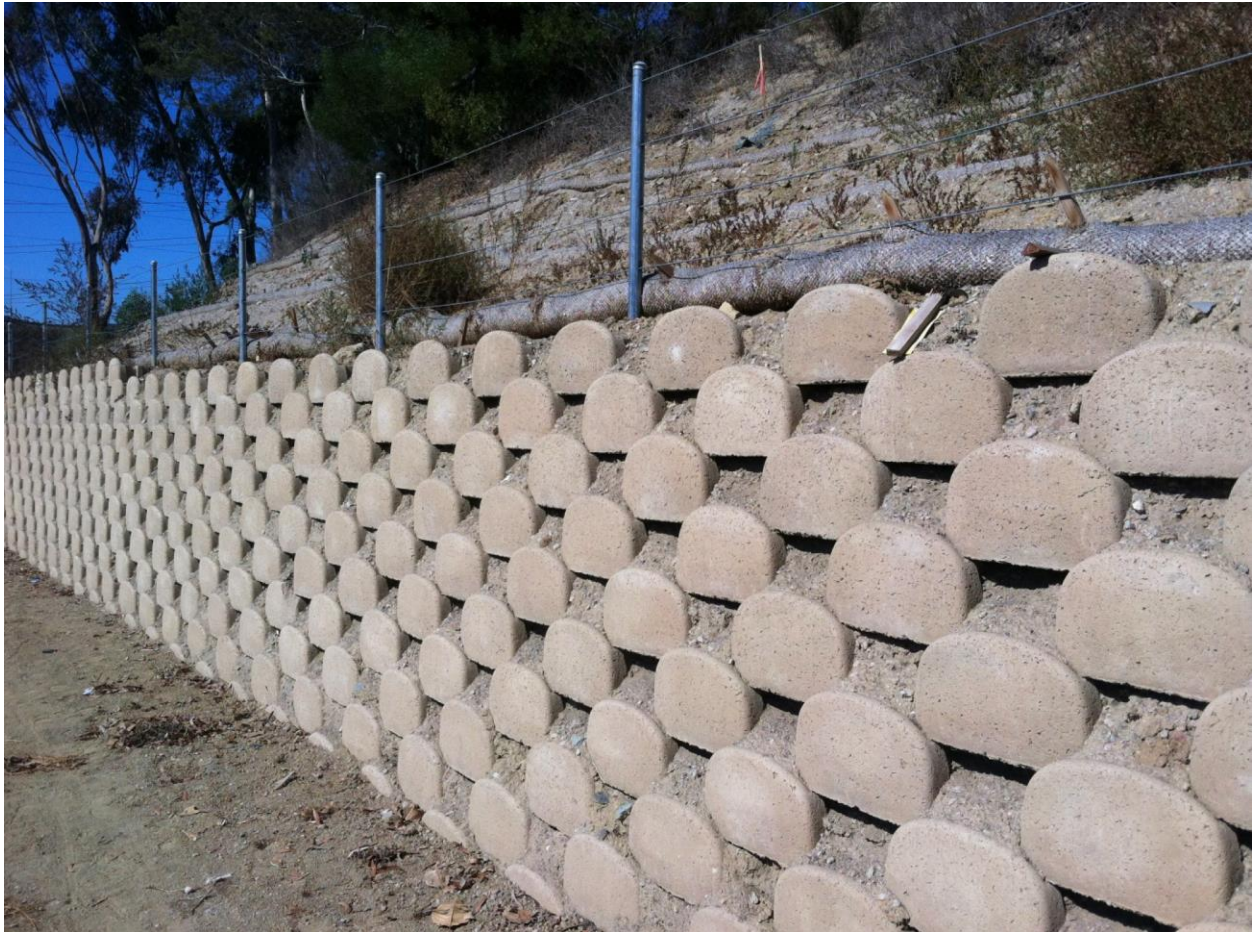
Figure 2.3-2 Typical Retaining Wall Face
