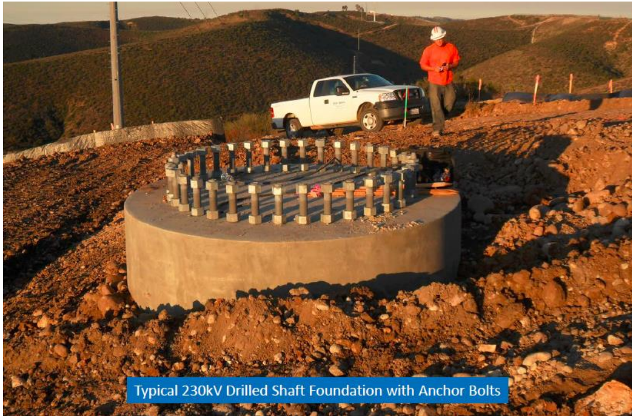
Figure 2.2-14 Representative Photographs of Concrete Pier and Micropile Foundations
