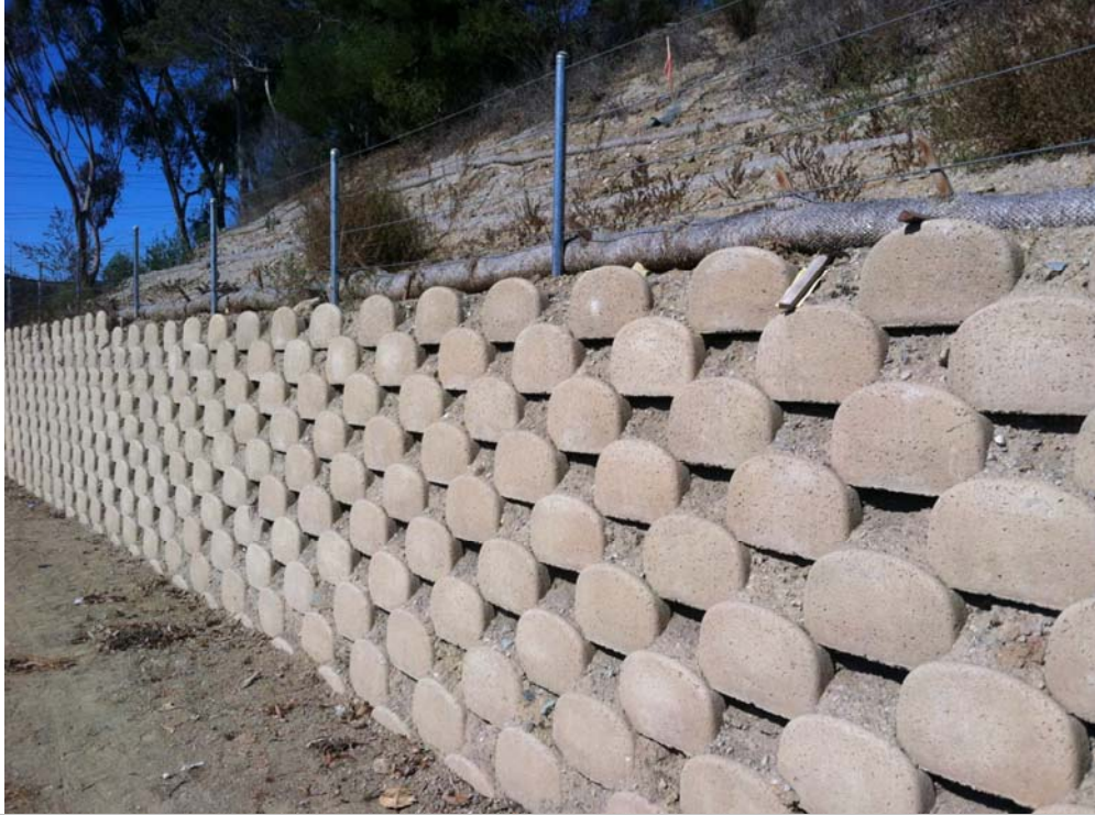
Figure 2.4-2: Typical Retaining Wall Face
