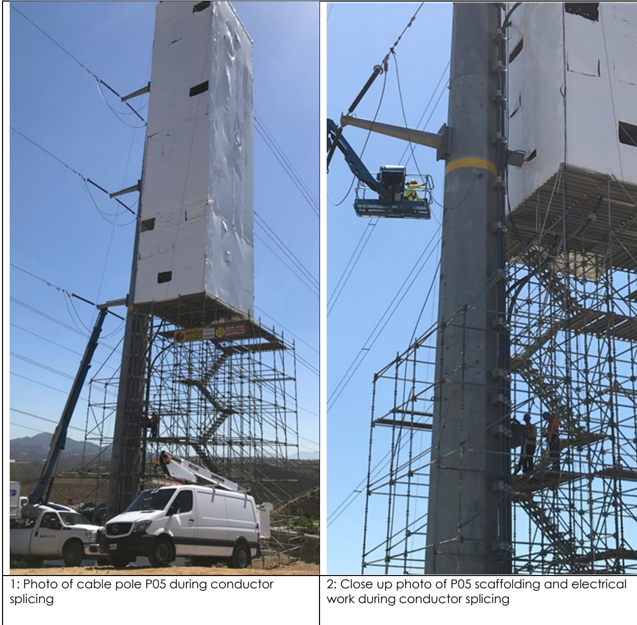
Figure 2.2-3 Shrouds Used for Conductor Splicing at Cable Poles
