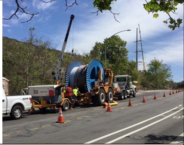
2: Conductor on reels for installation
