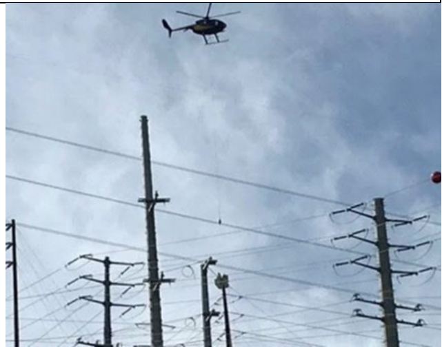
4: Helicopters were used to string the conductor
