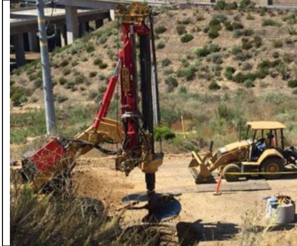
1: Drilling a TSP foundation
