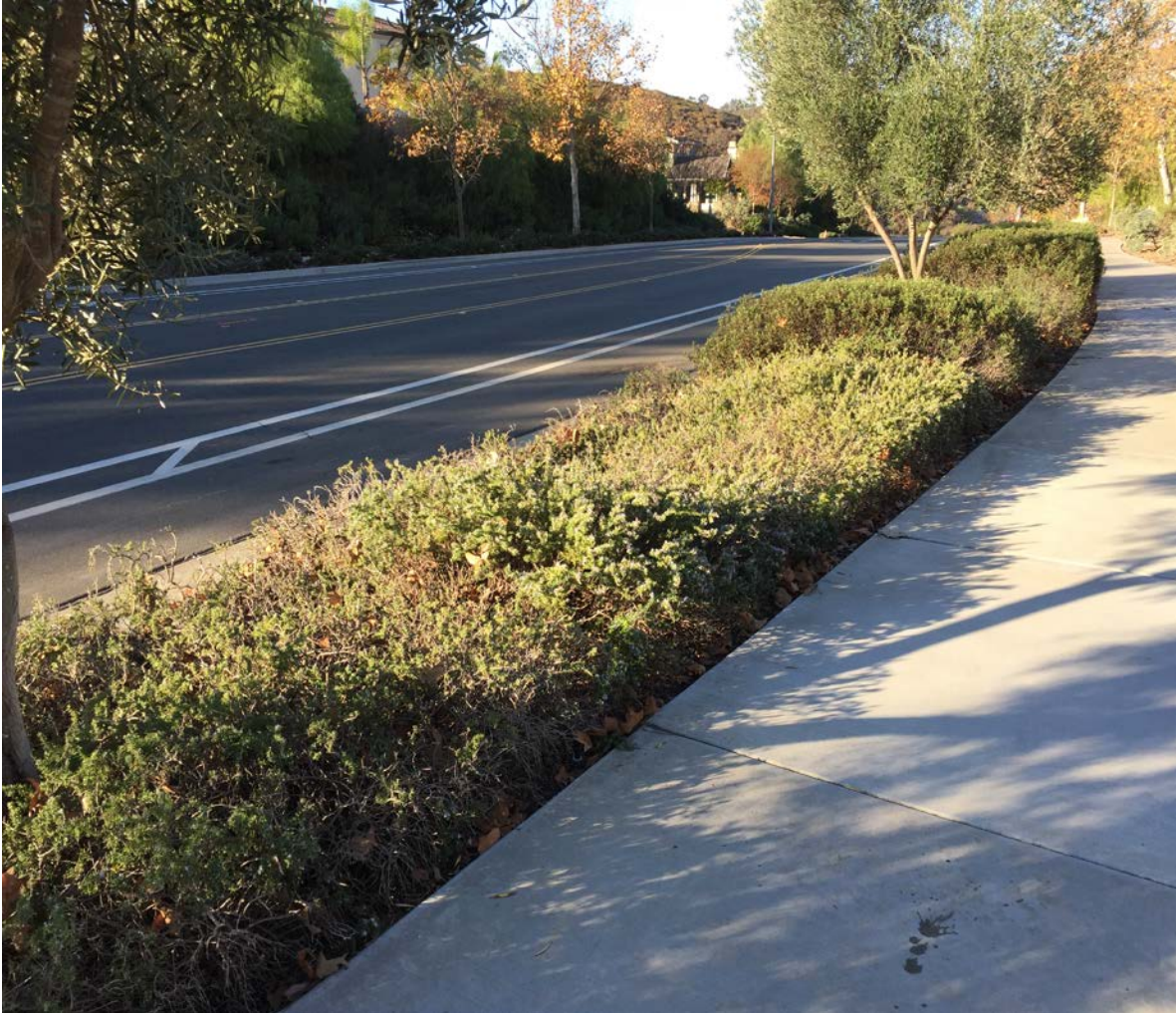
West facing view of the ornamental landscaping along Stonebridge Parkway where two steel plates will be placed to support crane outriggers.
