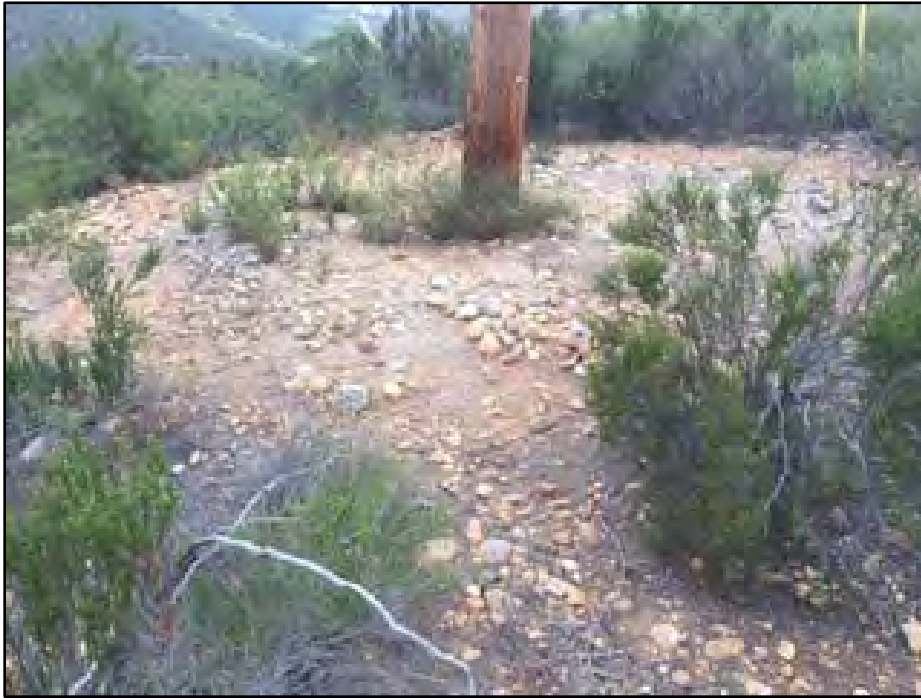
Photo 3: R3 (facing northwest towards existing 138 kV wood monopole to be removed and transitioned underground).
