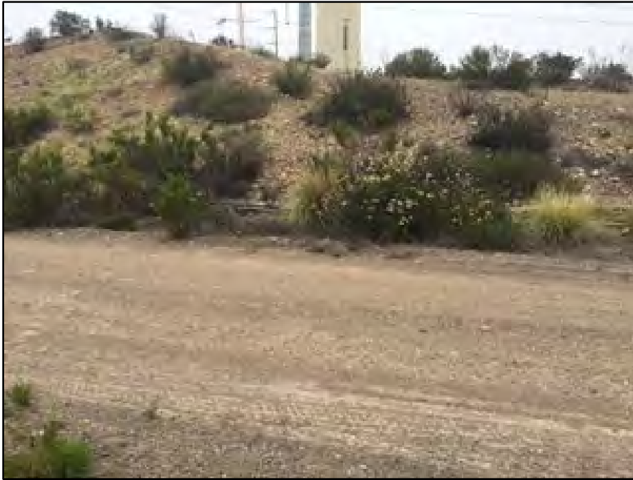
Photo 7: Underground Trenching (facing north towards portion of underground trenching in revegetated coastal sage scrub north of Sycamore Canyon Substation).
