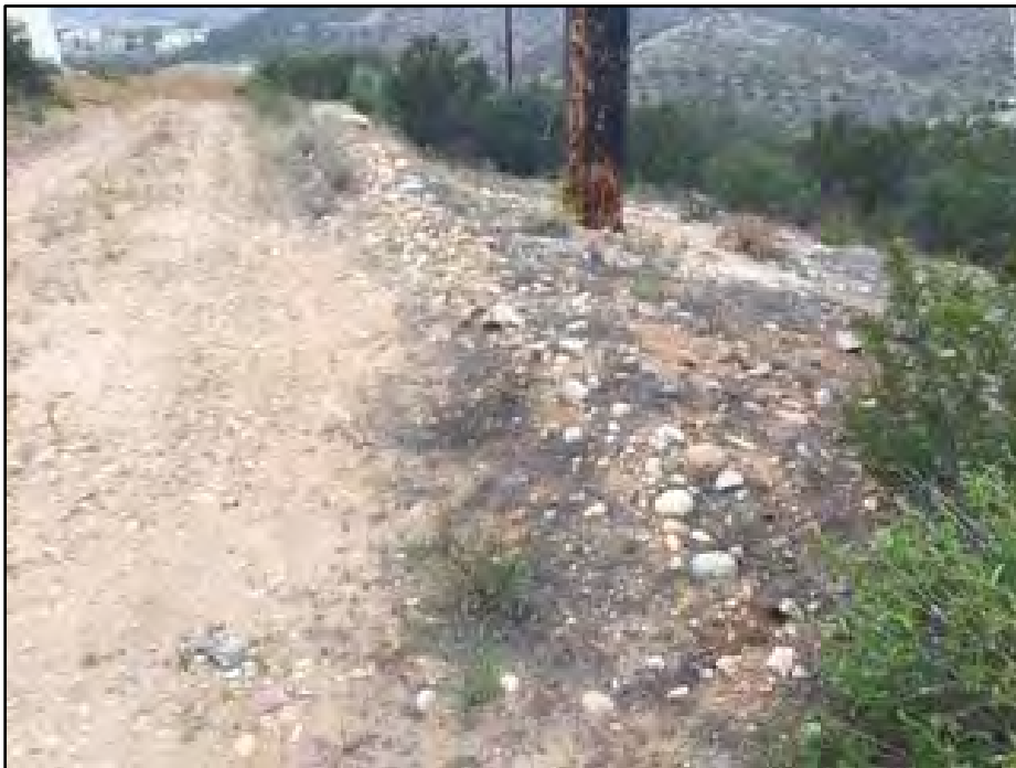
Photo 2: R2 (facing north towards existing 138 kV wood monopole to be removed and transitioned underground).
