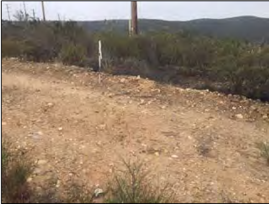
Photo 5: P03A/B (facing south towards proposed double-circuit 230 kV/138 kV steel monopole location of installation).
