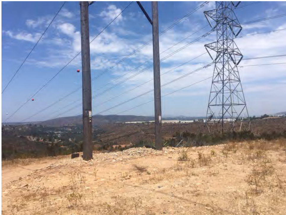
Figure 6: Northwest-facing view of proposed structure P06 and structure R6 to be removed.
