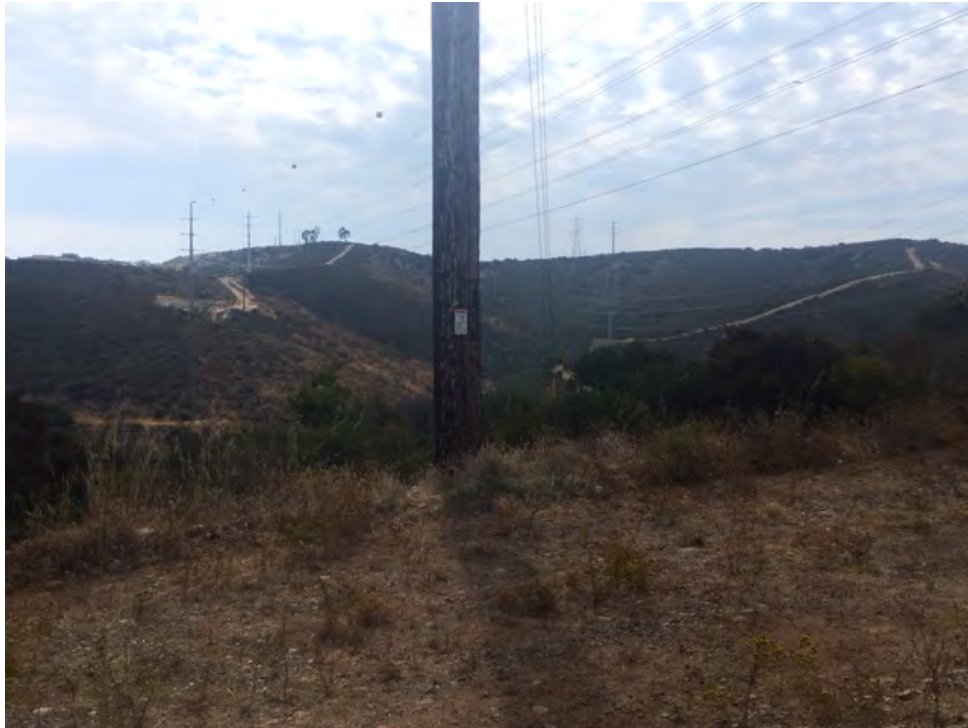
Figure 3: Southeast-facing view of structure R2 to be removed at location P03.
