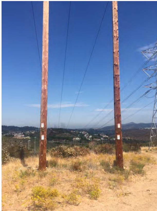
Figure 1: Northwest-facing view of structure R4 to be removed at location P04.
