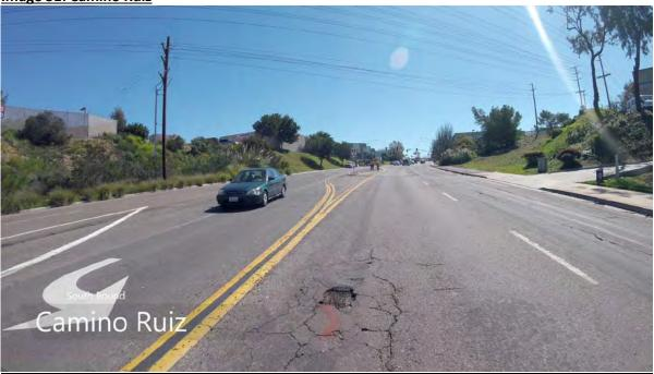
53) Activity Rd. and Camino Ruiz: west bound at 11:52, excessive wear and cracking at the intersection to the concrete drainage channel.
