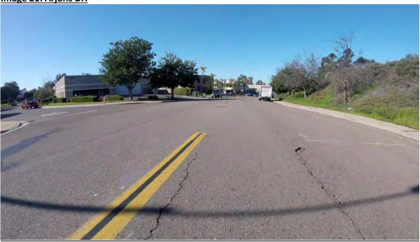
32) Trade Pl.: south bound at 19:24, excessive wear, damage, cracking entire length of road.
