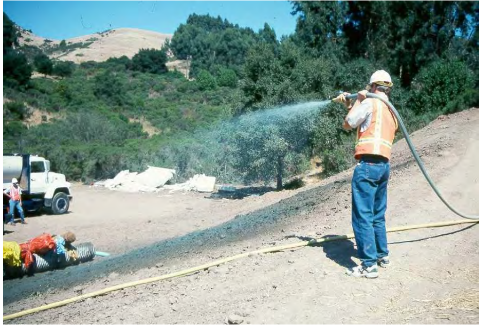
Applying hydroseed.
