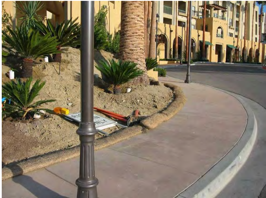
Fiber rolls as perimeter control.
