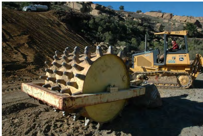
Sheepsfoot used for soil preparation
