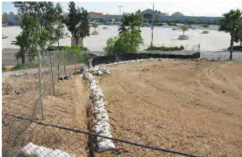
Gravel bags used as perimeter control.
