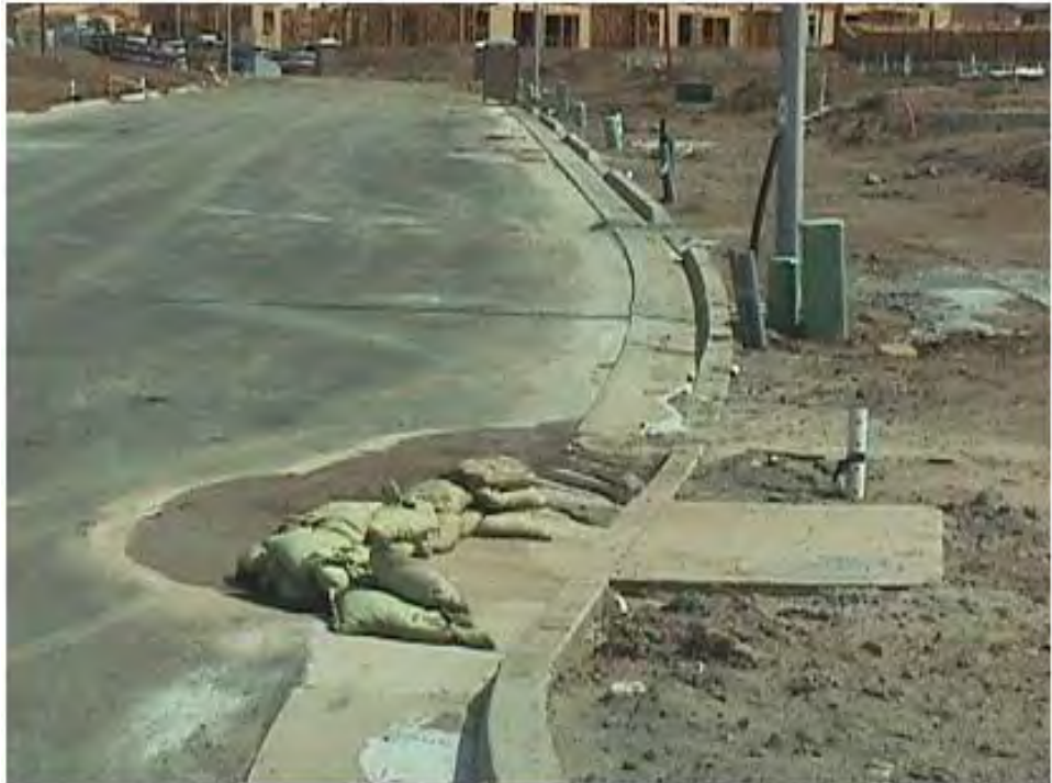
Gravel bag inlet protection.
