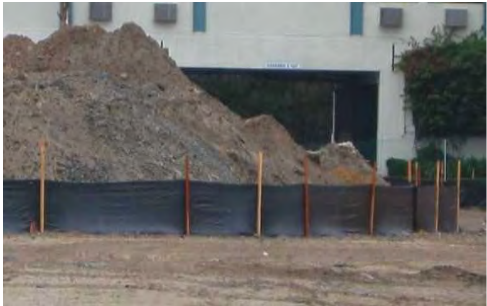
Silt fence used for stockpile perimeter control.
