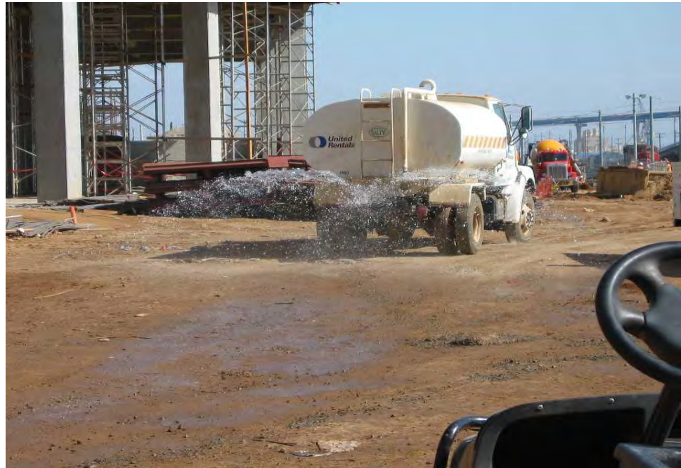
Water being applied for dust control.
