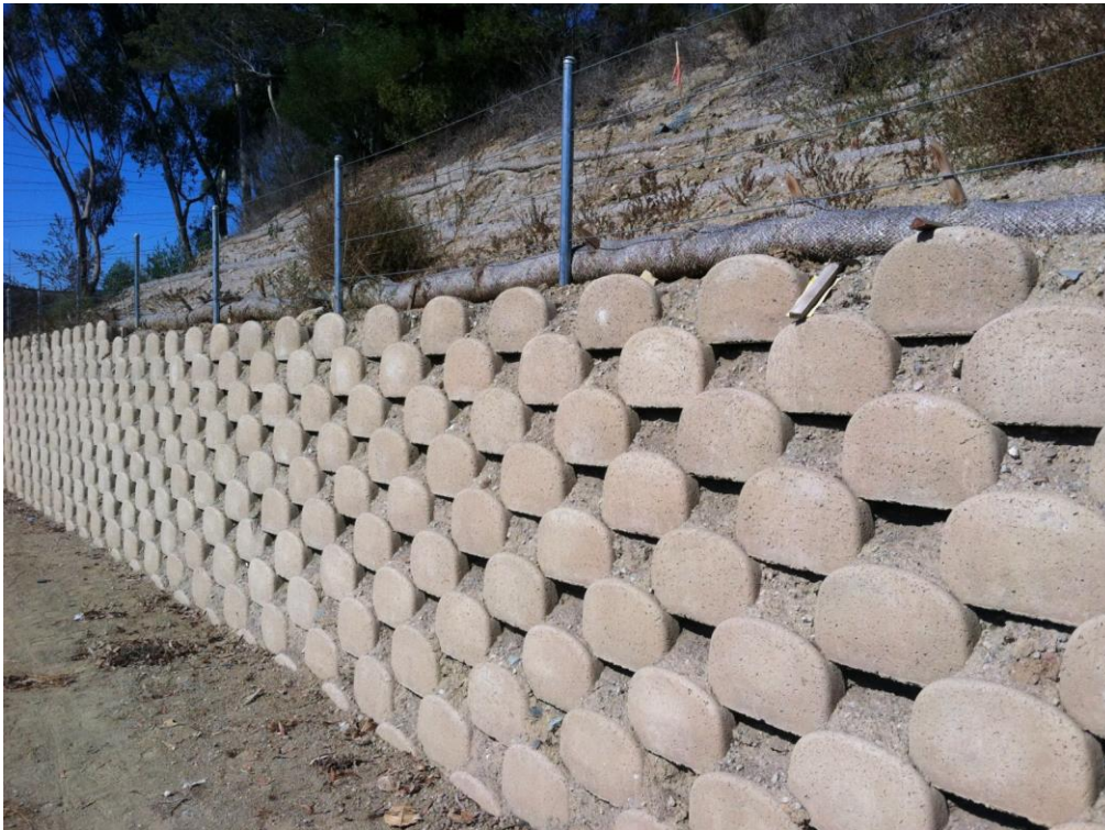
Figure 2.3-2 Typical Retaining Wall Face
