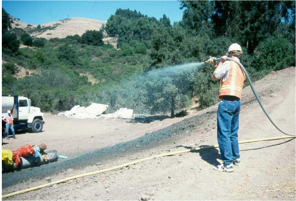
Applying hydroseed.
