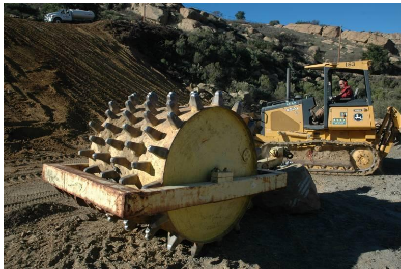
Sheepsfoot used for soil preparation
