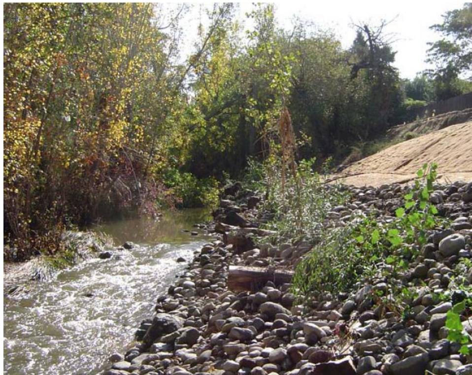
Cobble or gravel armor used for streambank stabilization.
