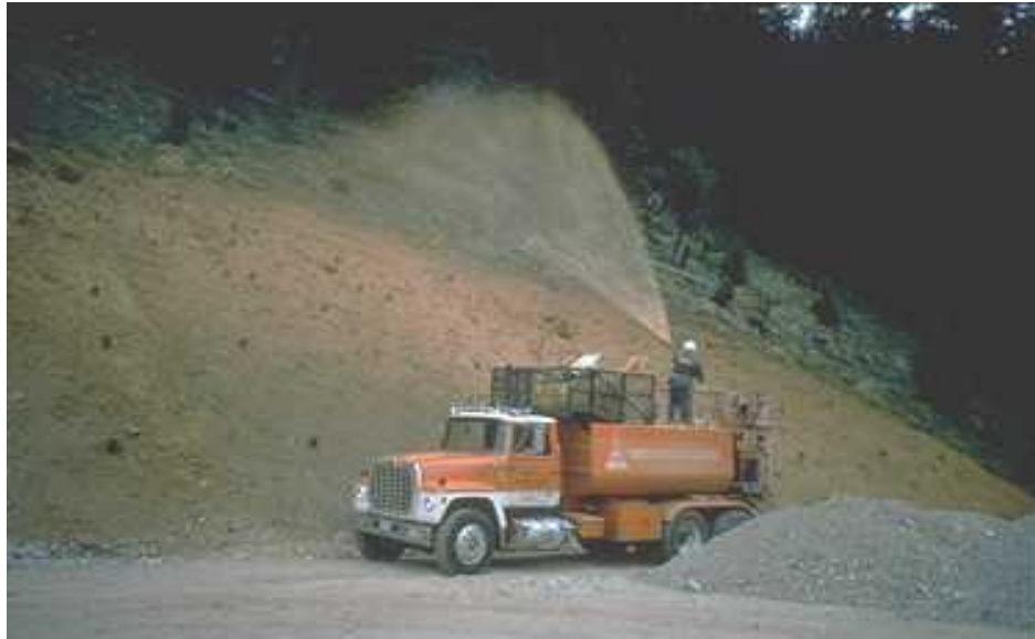
Applying hydraulic mulch.
