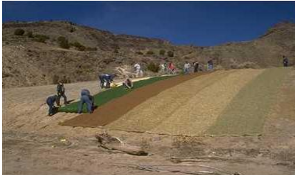
Several types of erosion control blankets.
