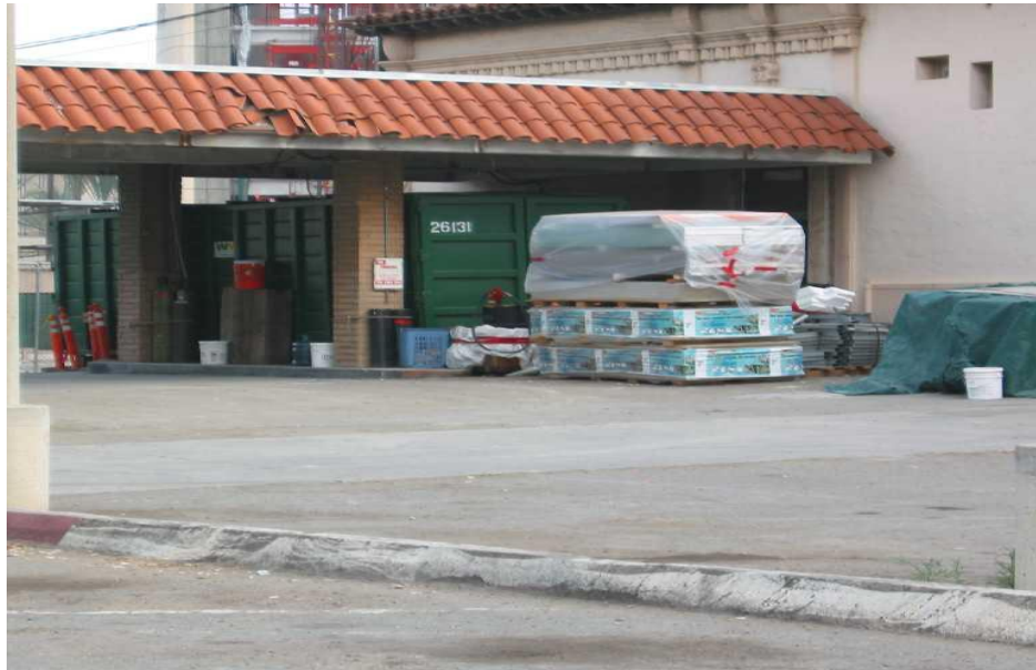
Materials are covered and neatly stored within a curbed area.
