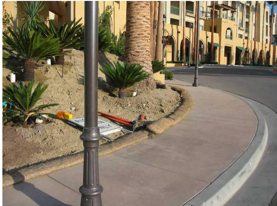
Fiber rolls as perimeter control.
