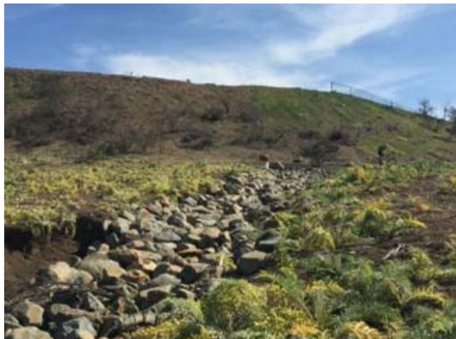
Photograph 21. Exempt, non-jurisdictional riprap-lined swale from constructed detention basin.
