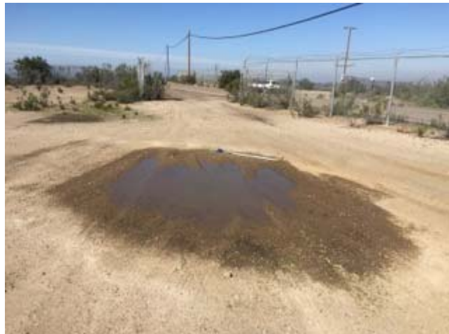
Photograph 15. Basin 1 within dirt road edge.
