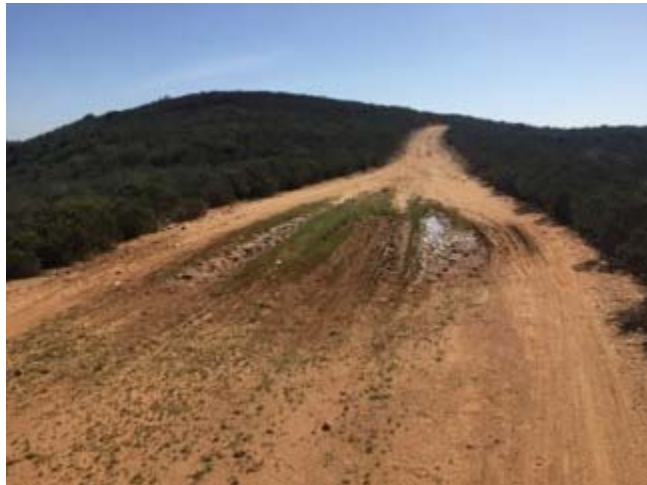
Photograph 17. Basin 15 within dirt access road.
