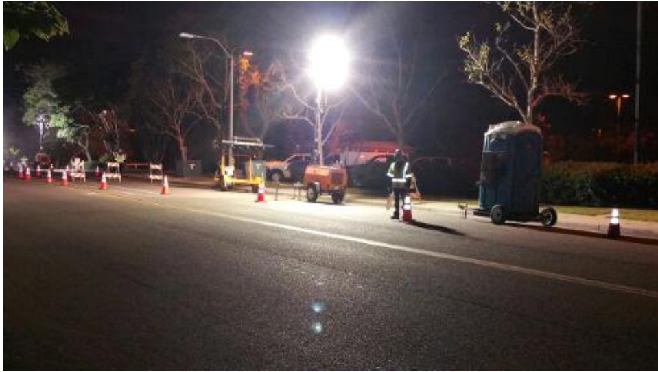
Caption Flaggers at west end of work area.
