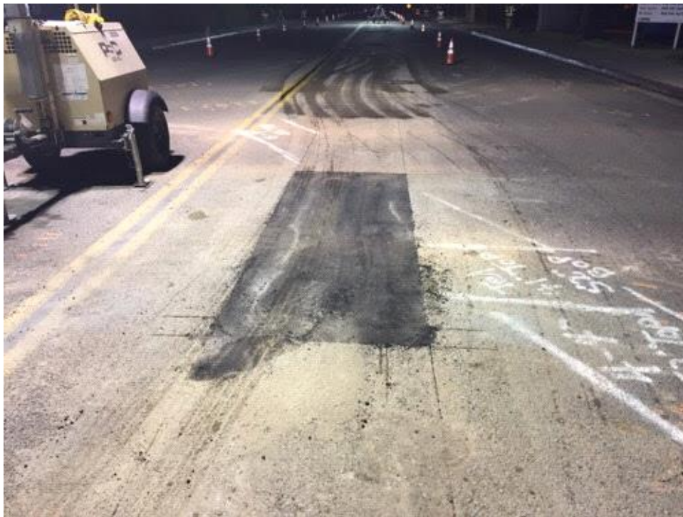
Caption Roadwork patched after completion.
