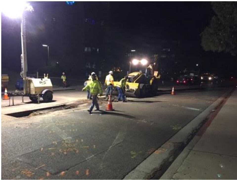
Caption Removing asphalt debris from the street
