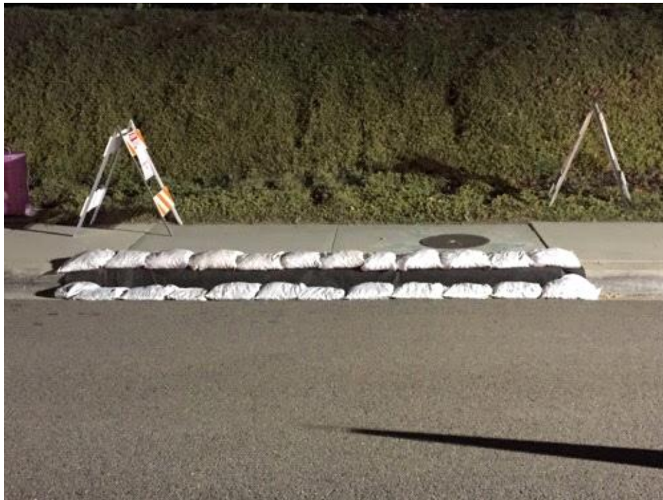
Caption SWPPP BMP's were in place
