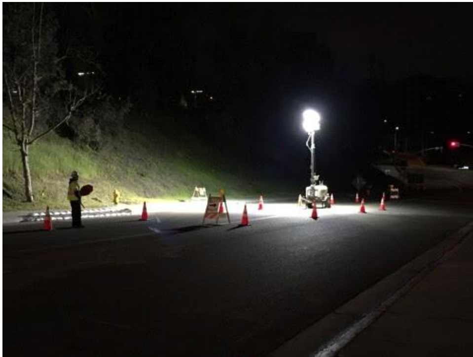
Caption Lighting, cones, traffic safety monitors in place.
