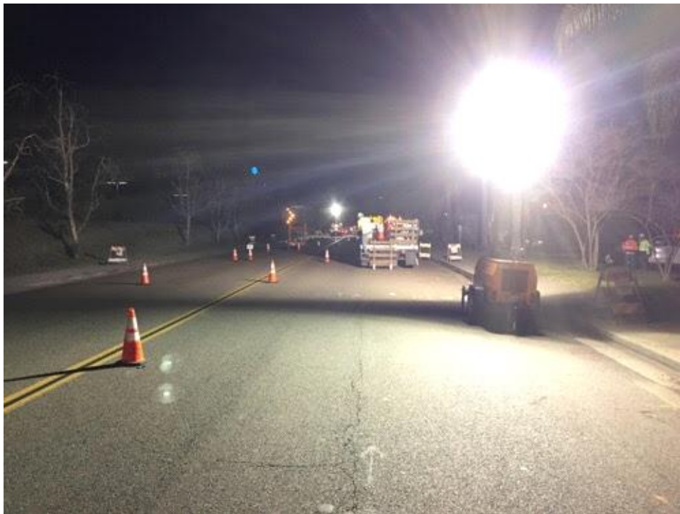
Caption Lighting was in place and work areas were well lit.
