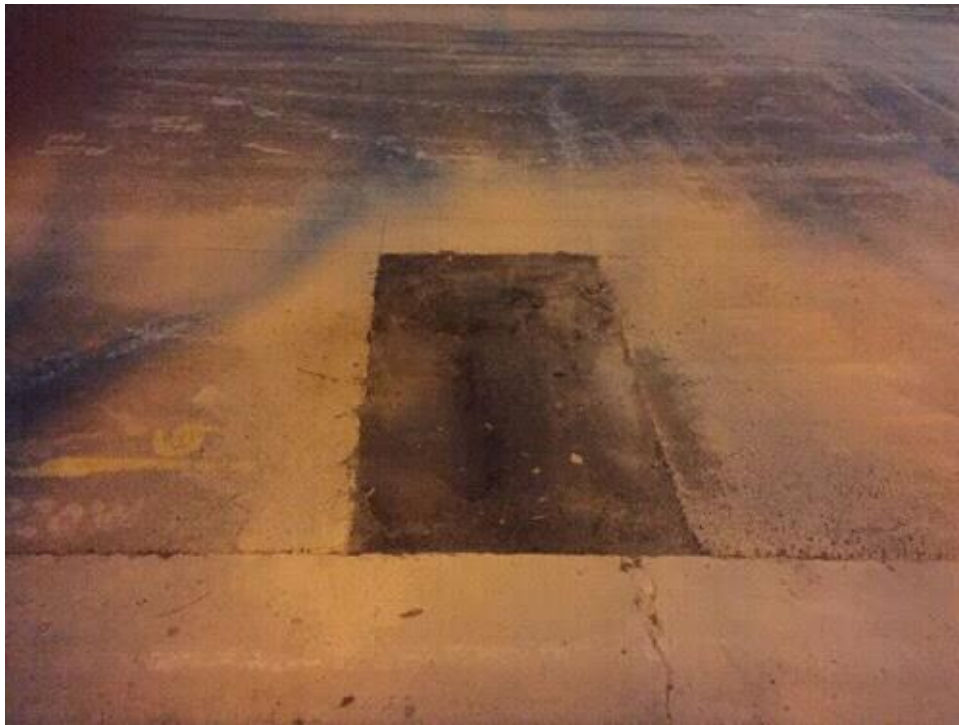
Caption Excavations restored to original condition
