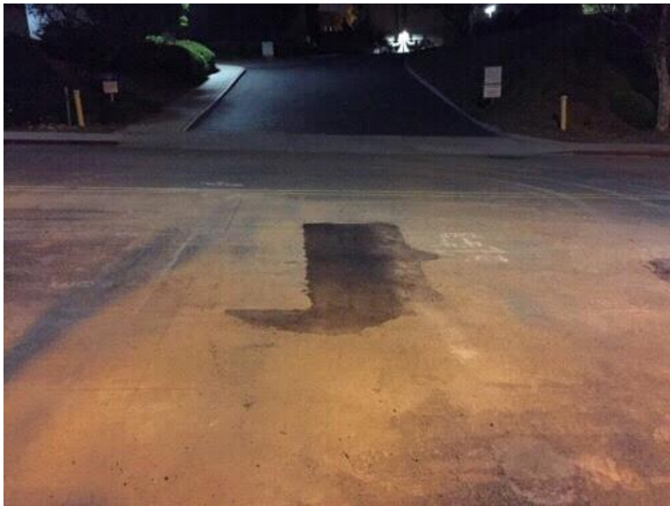
Caption Road work repaired to previous condition
