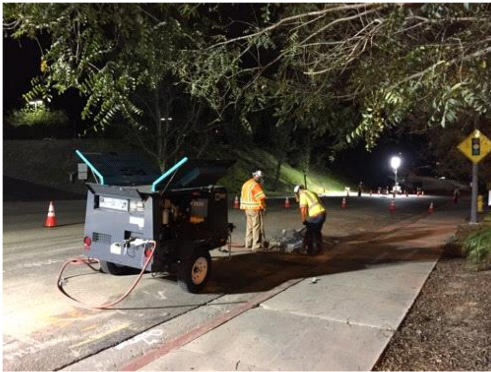
Caption Removing asphalt with jack hammer
