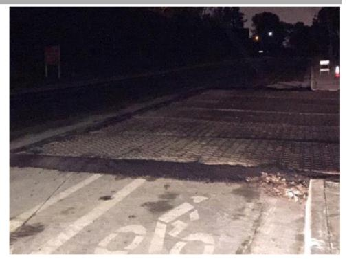
Caption Steel plates in place to cover trench. All sides patched with asphalt to seal the trench.
