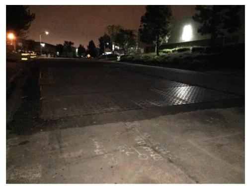
Steel plates covering trenches and seams filled with asphalt to cover completely. Caption
