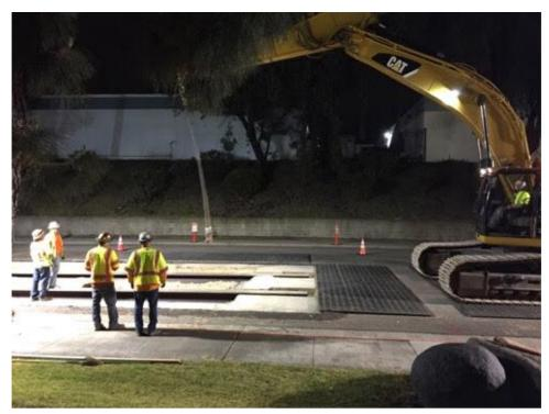
Caption Removing steel plates for shoring/ trench work.
