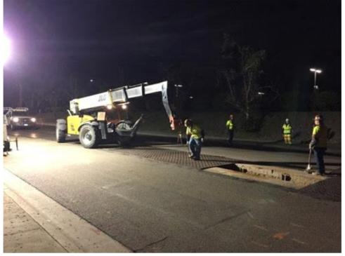
Removing steel plates from over the trenches. Capture Date/Time: Mon May 15 2017 20:44:08 GMT-0700 (PDT) Coordinates: 32.888773, -117.162770 Photo Attributes
