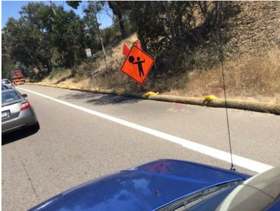
Caption BMPs in place on Pomerado Road.
