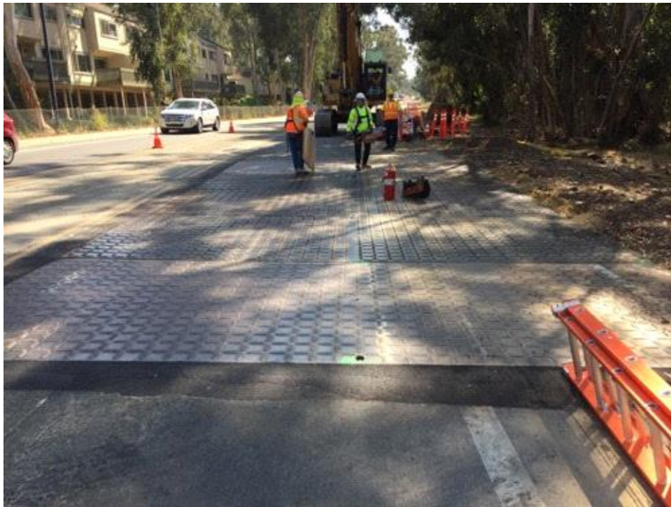
Caption Steel plates covering vault on Pomerado Road.
