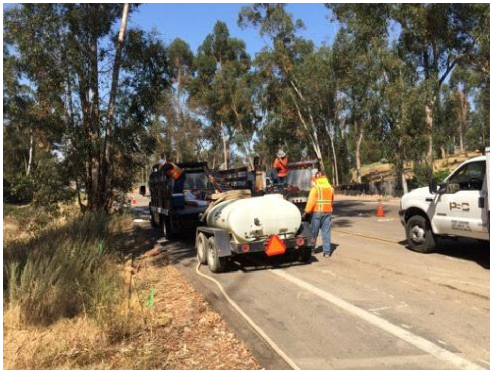
Caption Fire safety tech on site on Pomerado Road.
