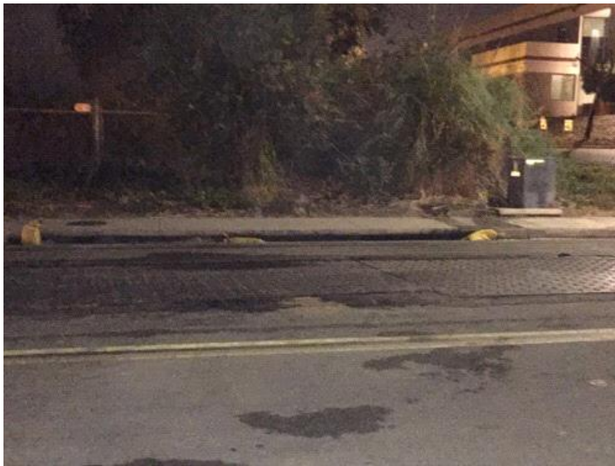
Caption BMPs in place and in good working order on Arjons Drive.
