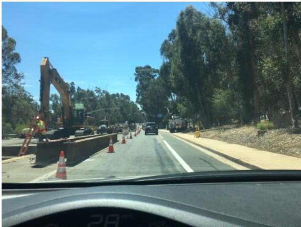
Caption Vault work on Pomerado Rd.
