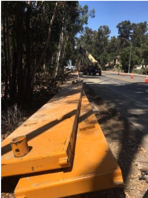
Caption Site storage and prep work for vault, Pomerado Road.
