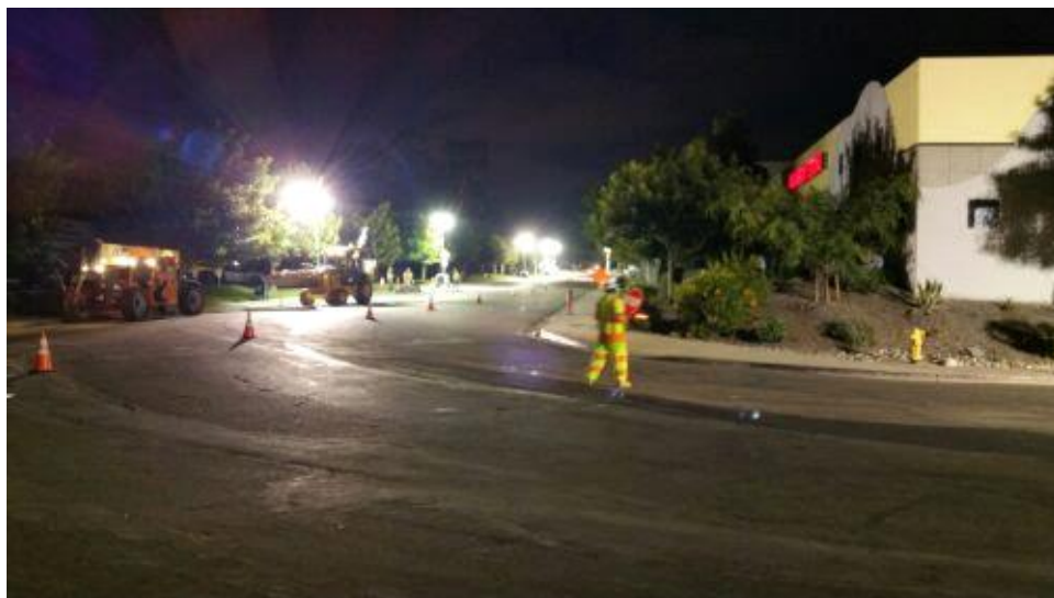
Caption Traffic control set before start of work.
