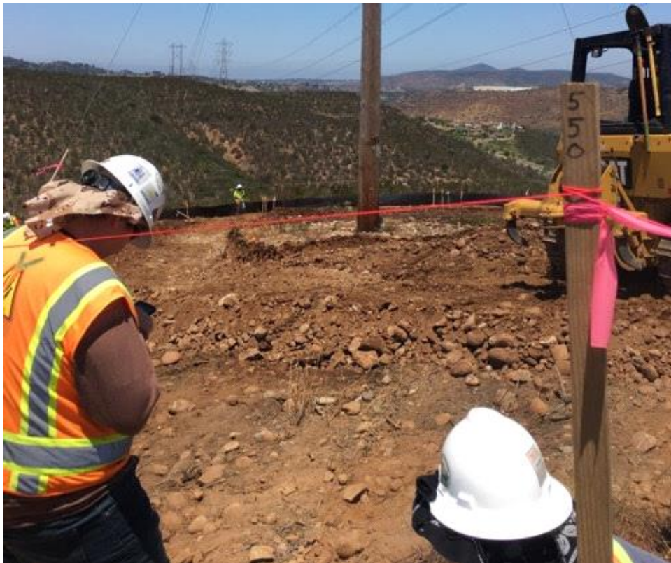
P03 clearing and grubbing...with silt fence in background.
