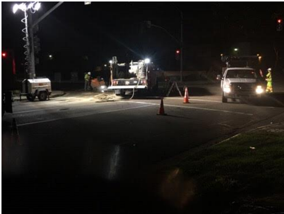
Caption Asphalt cutting Arjons Dr/Miraloni Dr intersection.
