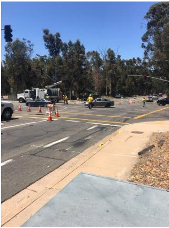
Caption Traffic control and potholing on Ave Nations/Pomerado Road intersection.
