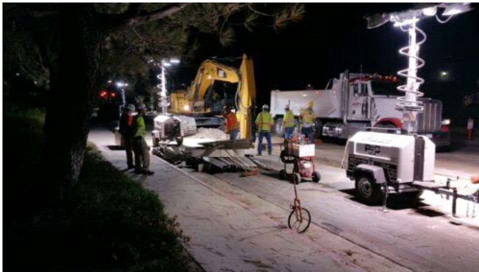
Caption Excavation (Miralani Dr.). Cultural resource monitors present.
