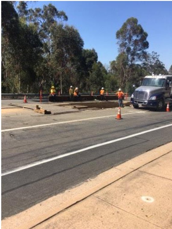
Caption Vault work on Pomerado Road.
