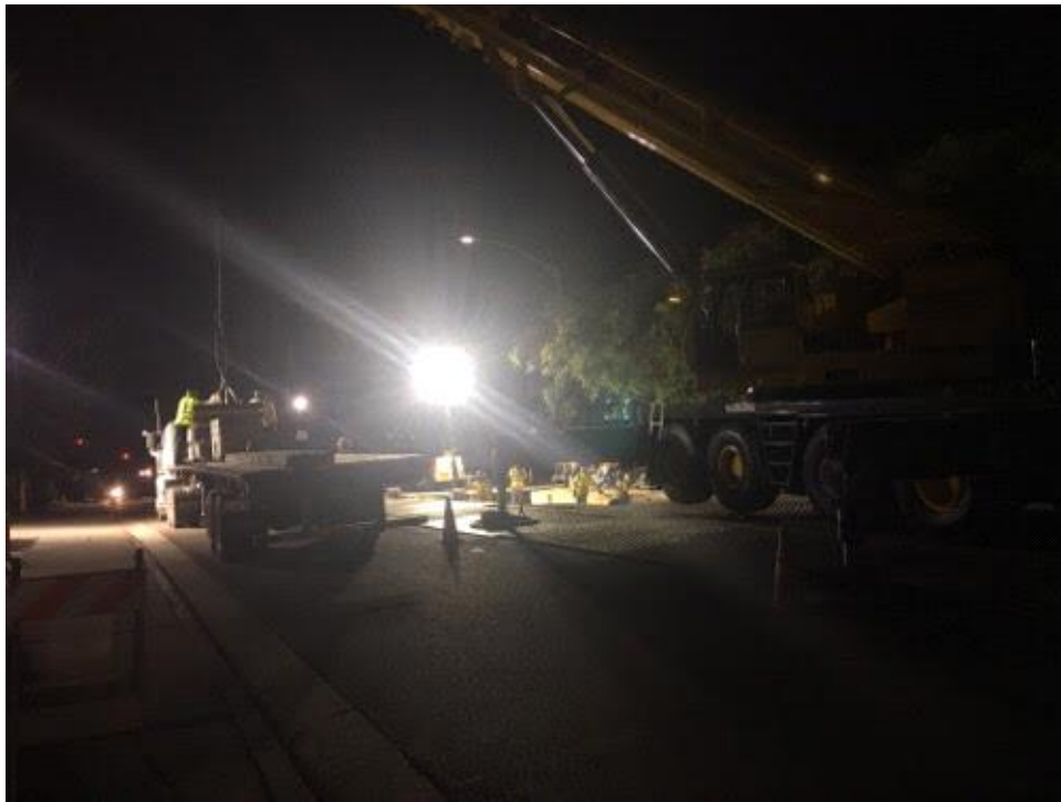
Caption Crane and vault installation
