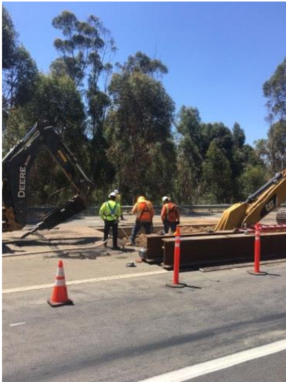
Caption Excavation and paleo monitoring on Pomerado Road.
