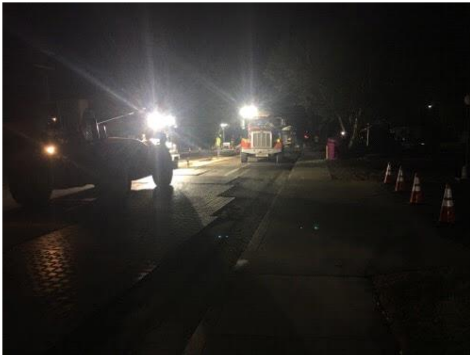
Caption Concrete work on Carrol near Crestmar Pt.
