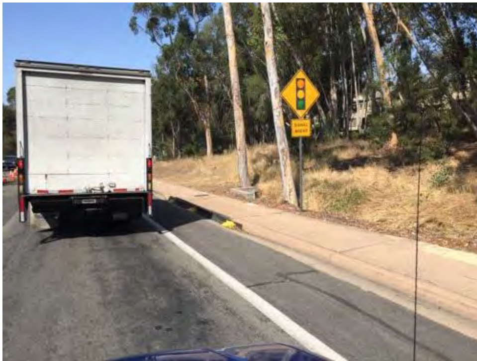
Caption BMPs in place on Pomerado Road.
