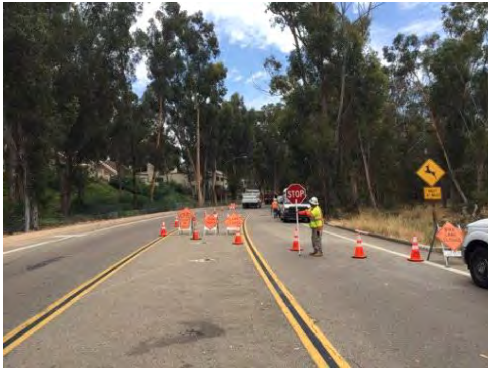
Caption Traffic flaggers on site at Pomerado Road.
