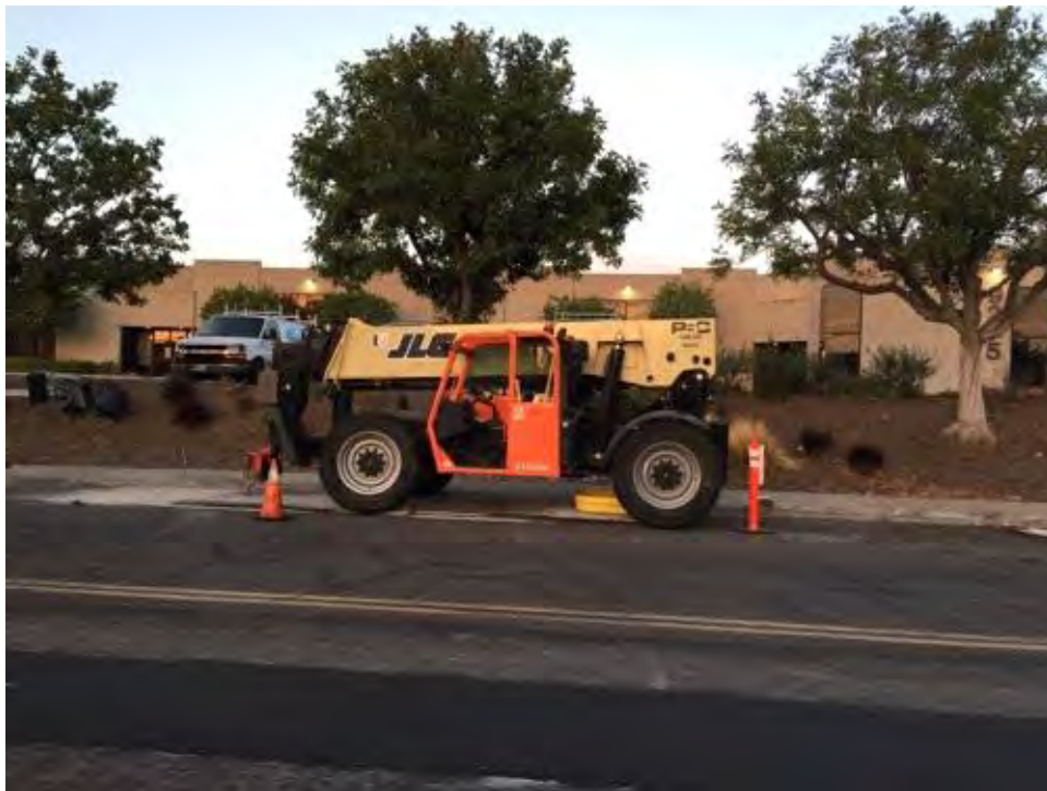
Caption Drip pans in place on Trade Place.
