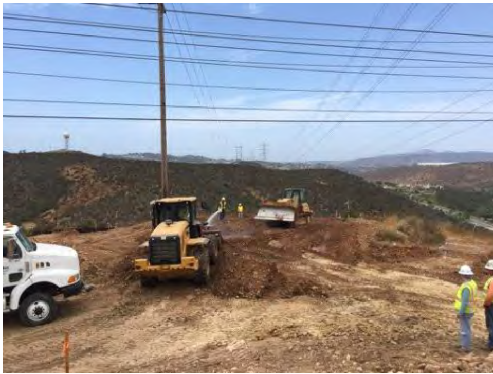
Caption Dust control measures in practice at Pole site 03.
