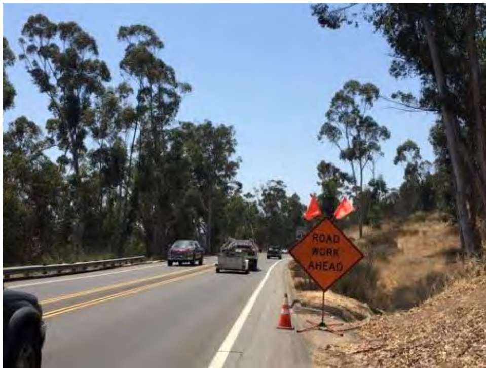
Caption Work areas clearly marked on Pomerado Road.
