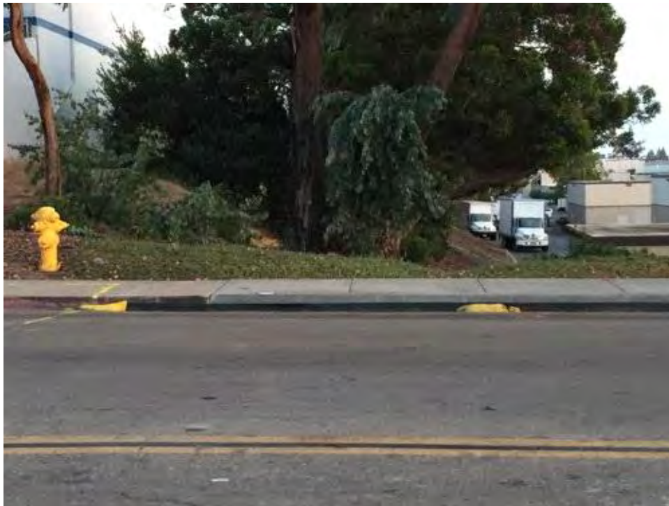
Caption BMPs in place on Arjons Drive.
