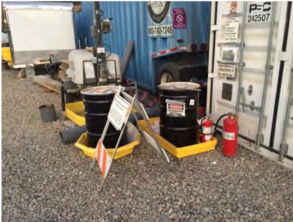
Caption Hazardous materials clearly labeled and stored within secondary containment.
