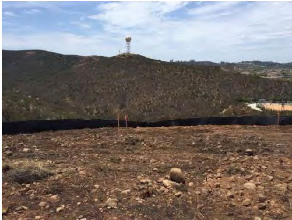
Caption Silt/erosion fencing installed at Pole 04.
