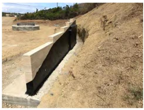
Caption Waterproofing on retaining wall at CC MM CP.
