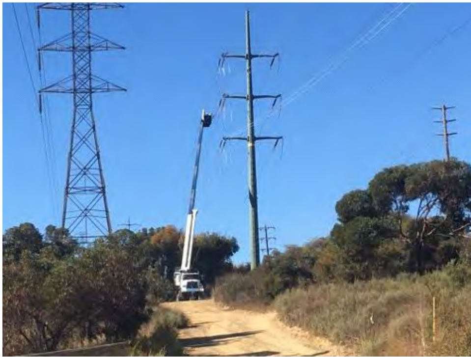
Caption Wire work on middle arm of pole north of CC MM CP.
