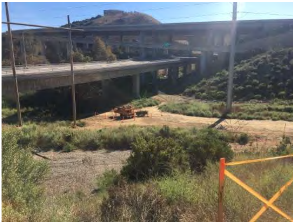
Caption Wire machine not in use and staged just north of Carroll Canyon Road bridge.
