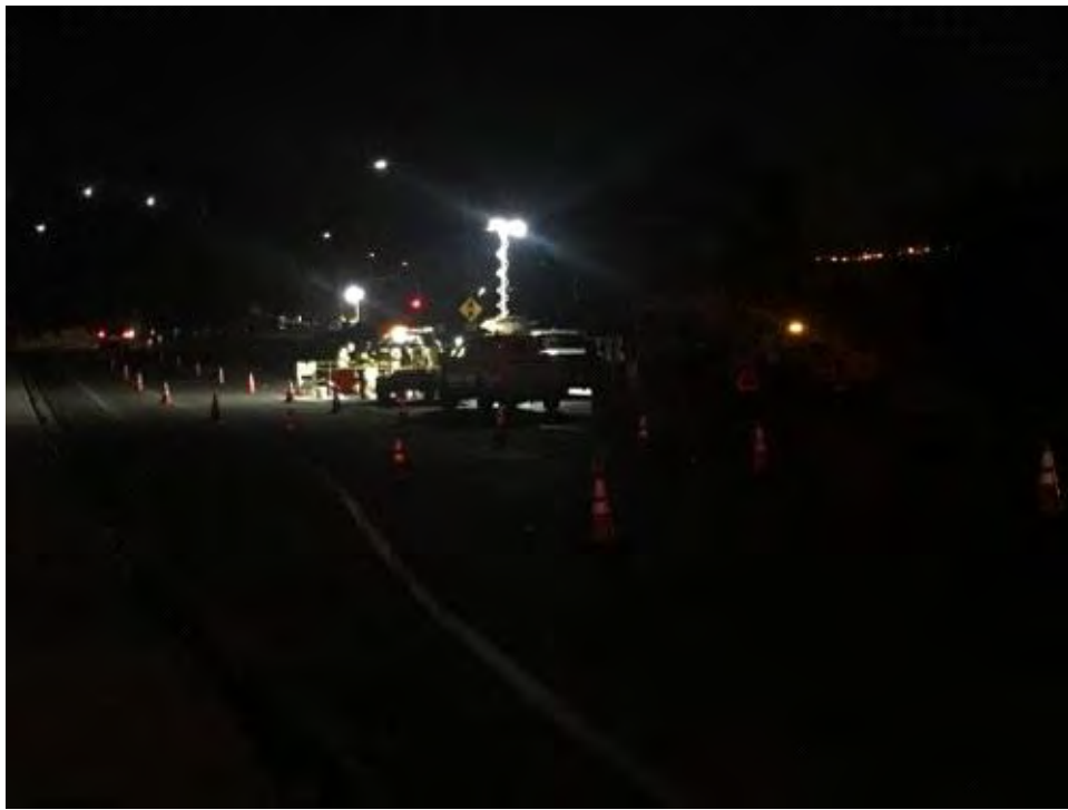
Caption Vault work on Carroll Canyon Road.
