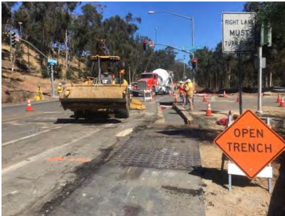
Caption Backfill at Chabad Center and Pomerado Road.
