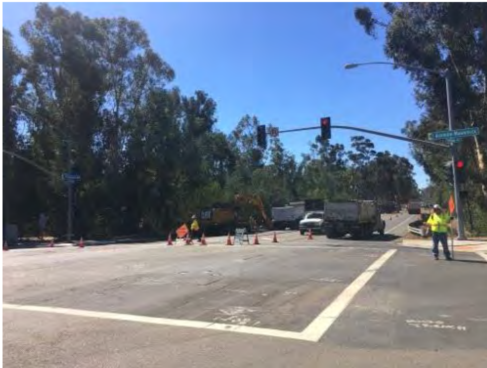
Caption Excavation on Pomerado Road, monitors onsite.
