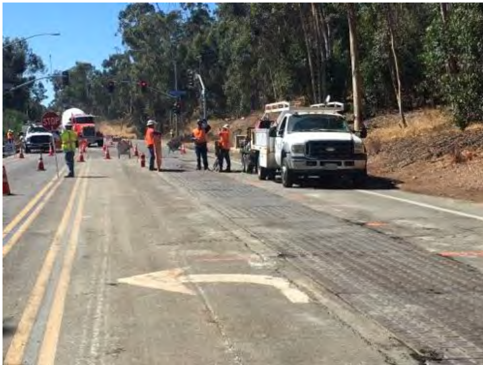
Caption Steel plate welding, note fire shield in use.
