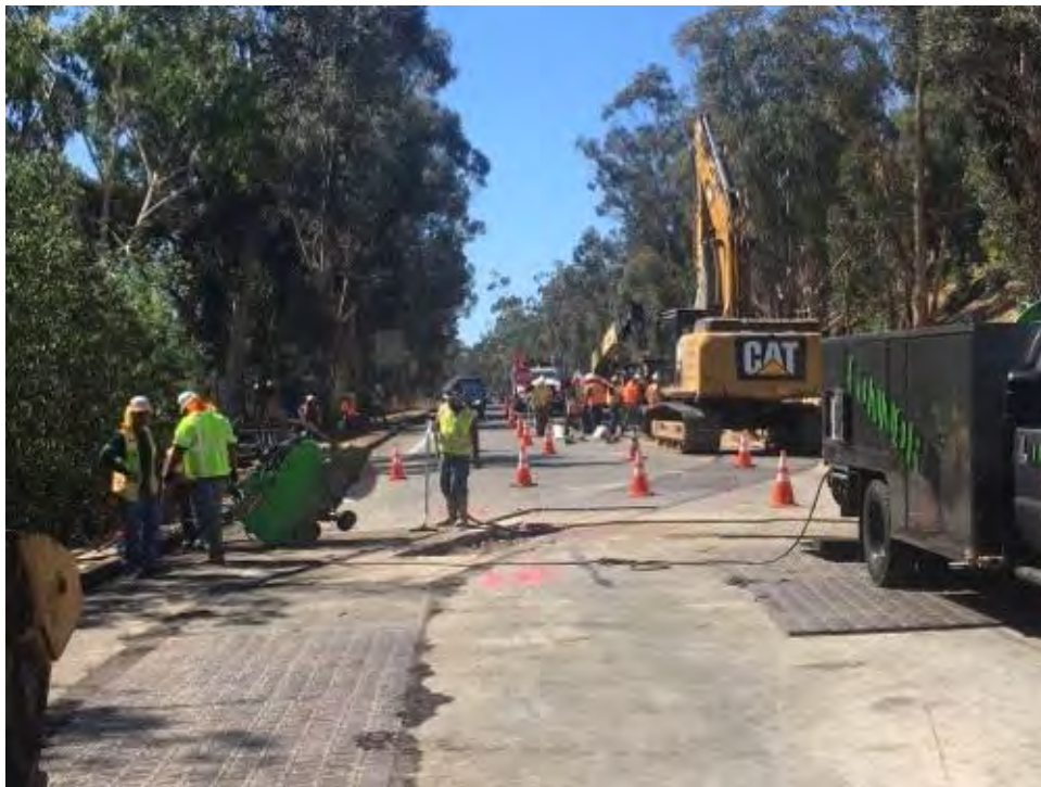
Caption Concrete work on Pomerado Road.
