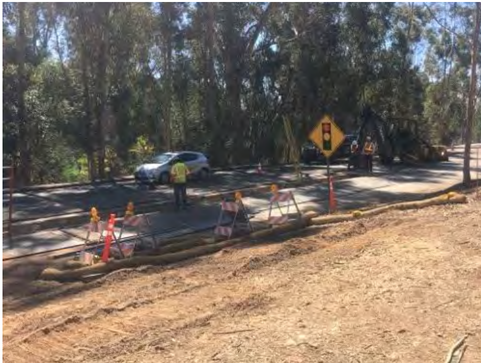
Caption Conduit install east of Chabad Center.
