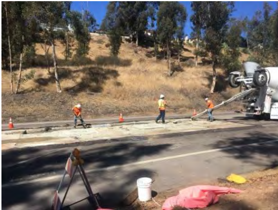
Caption Vault concrete work east of Fairbrook Road.
