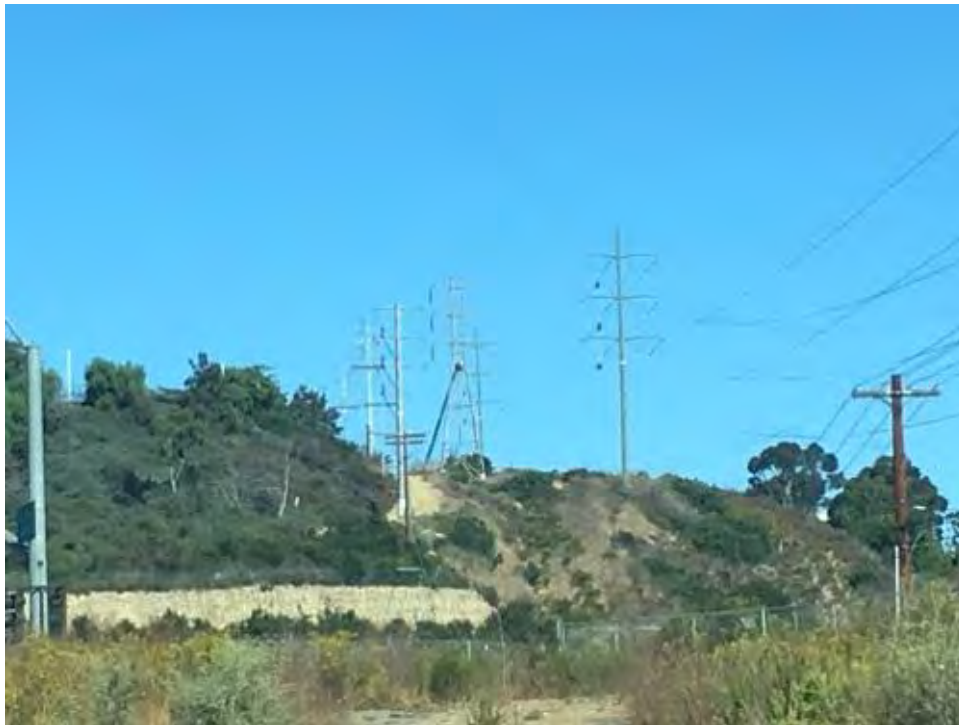
Caption Wire work north of Penasquitos substation.
