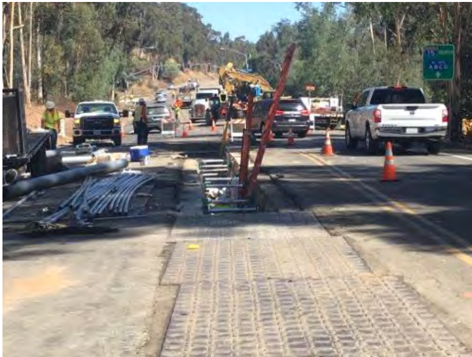
Caption Conduit install on Pomerado Road.
