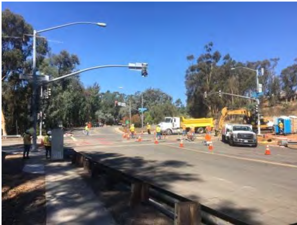
Caption Avenida Magnifica and Pomerado Road, excavation monitors are onsite.
