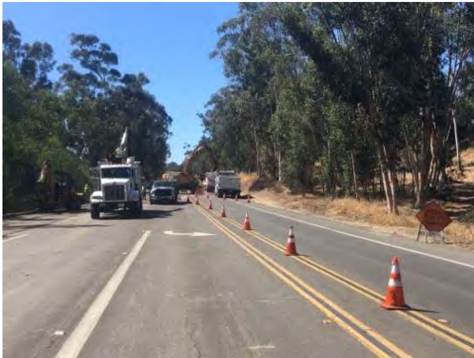
Caption Excavation west of Avenida Magnifica.
