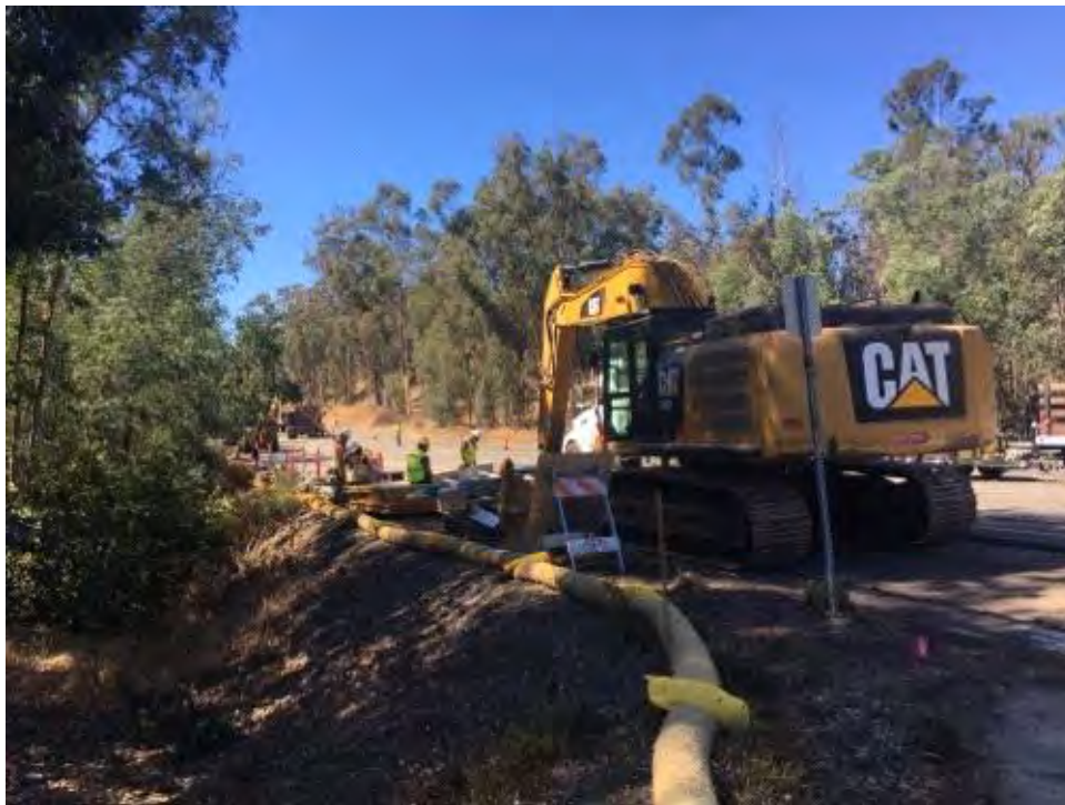
Caption Monitors, BMPs and fire safety personnel onsite at excavation on Pomerado Road.
