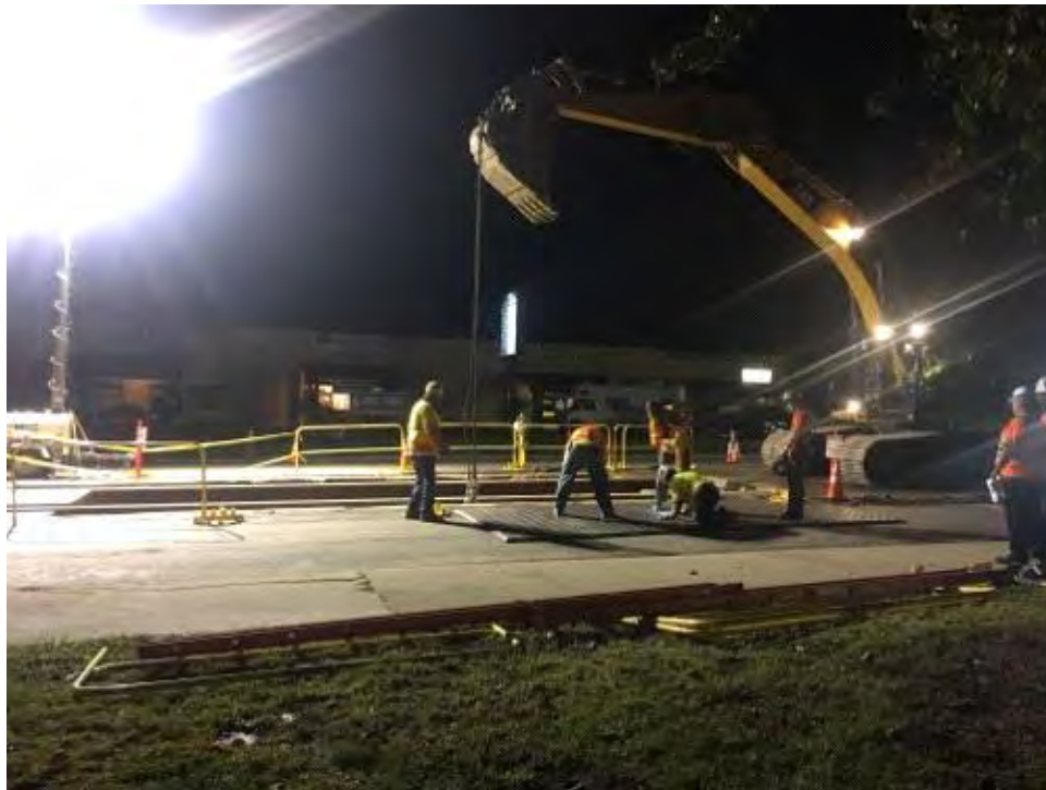
Caption Site prep for vault location.
