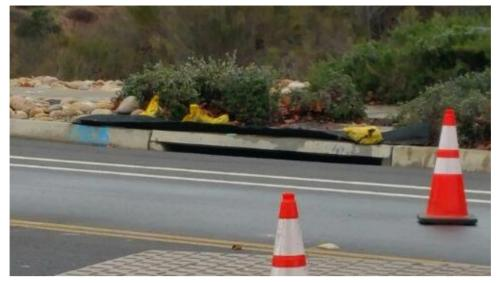
Caption Storm drain at bottom of hill on Stonebridge uncovered during rain event to prevent water back-ups.
