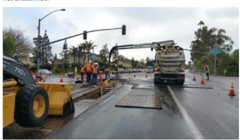
Caption Removing stormwater from trench on Pomerado Road corner.
