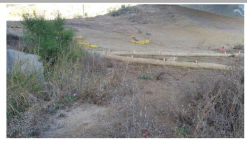
Caption Sediment flow past last project BMPS at bottom of roadway below CC MM CP site. Appears to be minor portion of total
