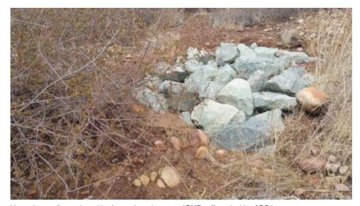
Caption Very minor sediment deposition beyond erosion control BMPs off south side of PO4.
