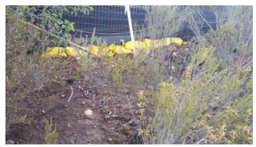
Caption Erosion control BMPs below main work area of PO4 intact, with minimal or no sedimentation below them.
