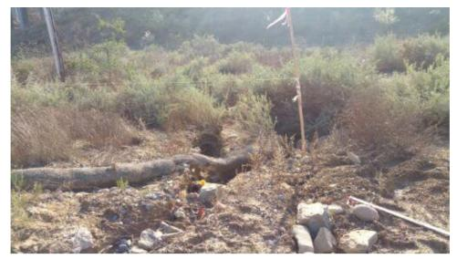
Caption Erosion gully breached BMPs at CC MM CP. Series of wattles and plastic had been in place per foreman,
