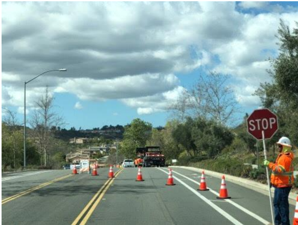
Caption Traffic control on Stonebridge Parkway.
