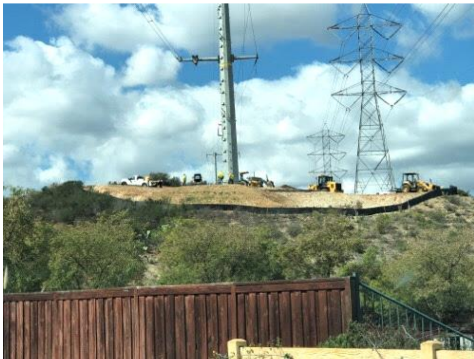
Caption P05 work site.
