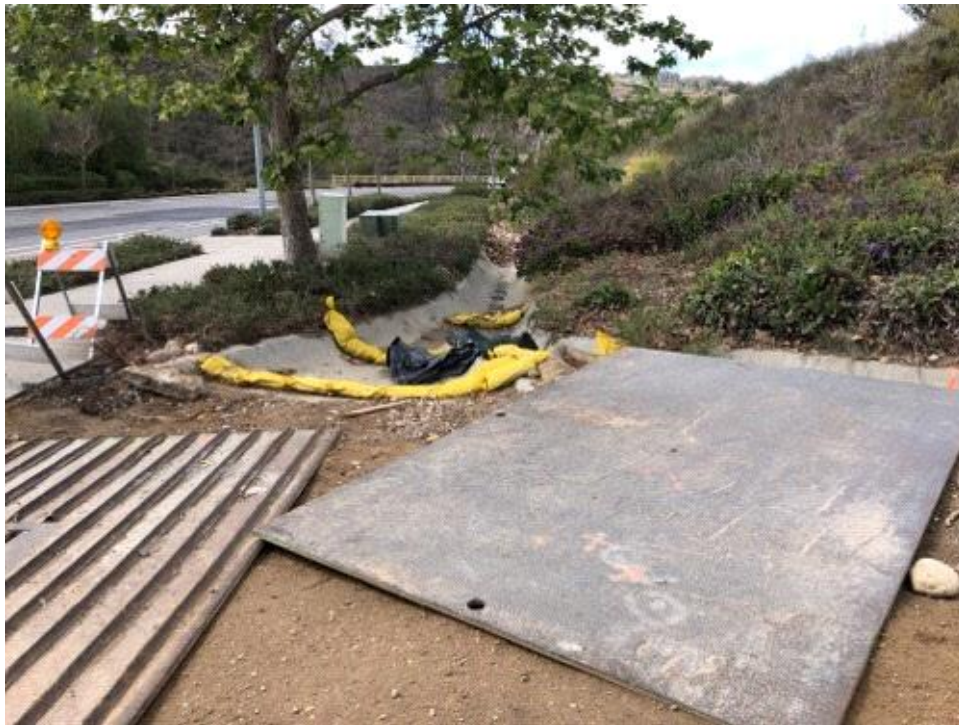
Caption BMPs at entrance to P05.
