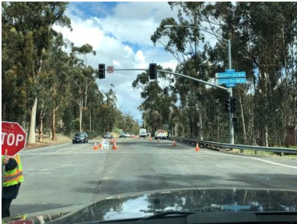
Caption Vault work and traffic control on Pomerado Road.
