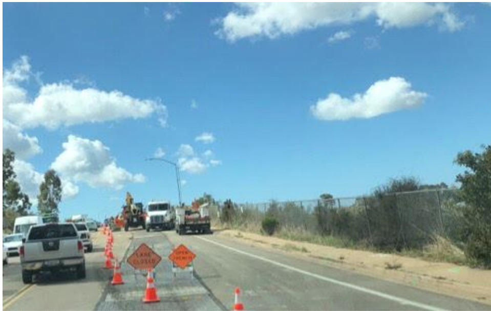
Caption Trench work on Pomerado Road.
