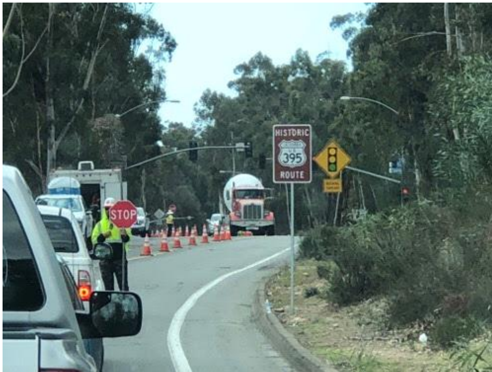
Caption Traffic control and vault work on Pomerado Road.
