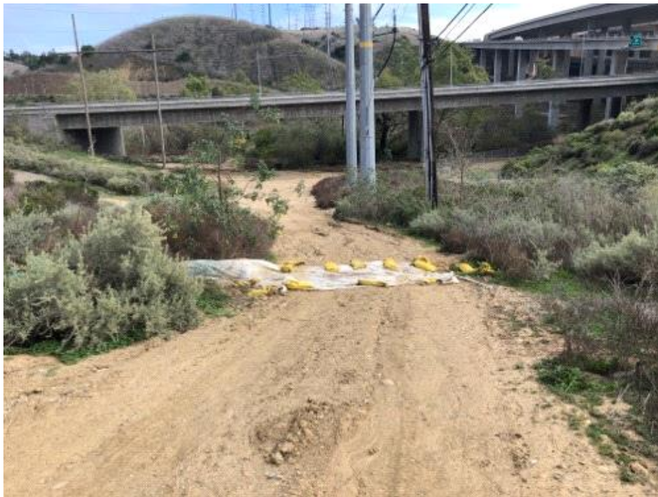
Caption Water berm/bar on road west of CC MM CP.
