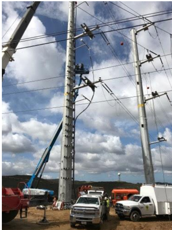
P03 with one line getting positioned for the transformer.
