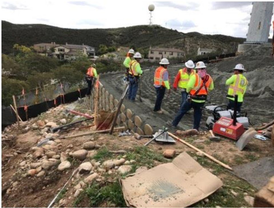
Caption Installing Verdura block retaining wall at P05.
