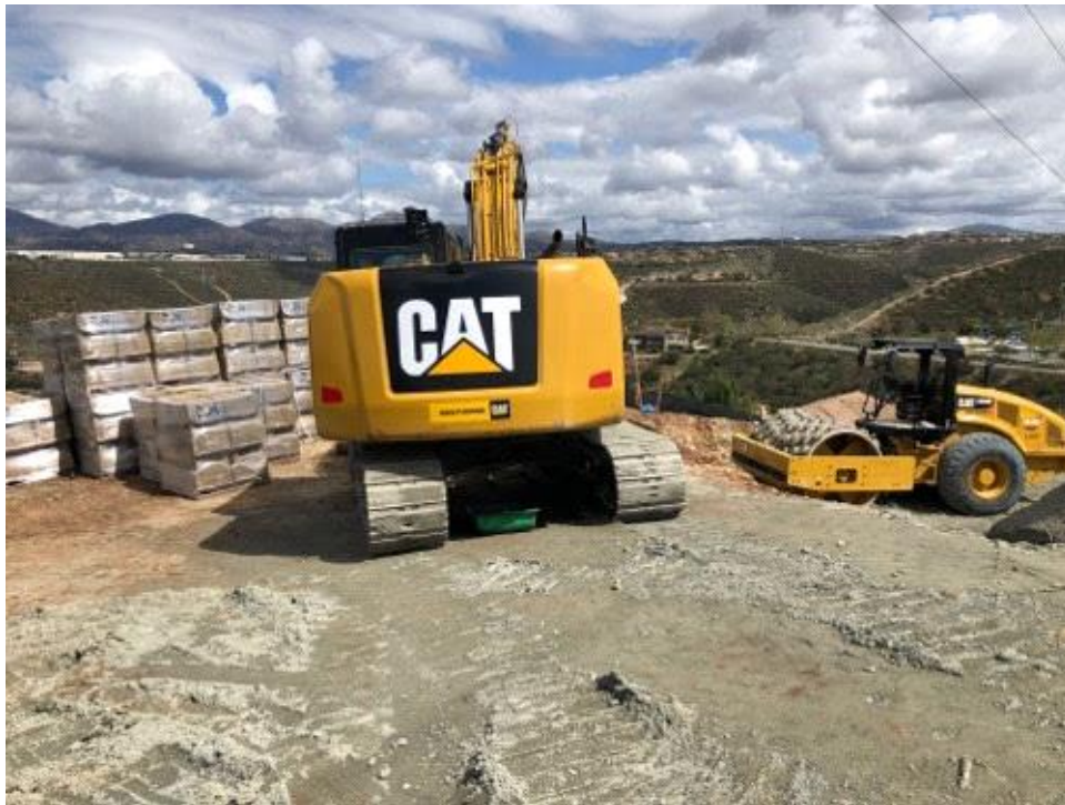
Caption Excavator with drip pan.
