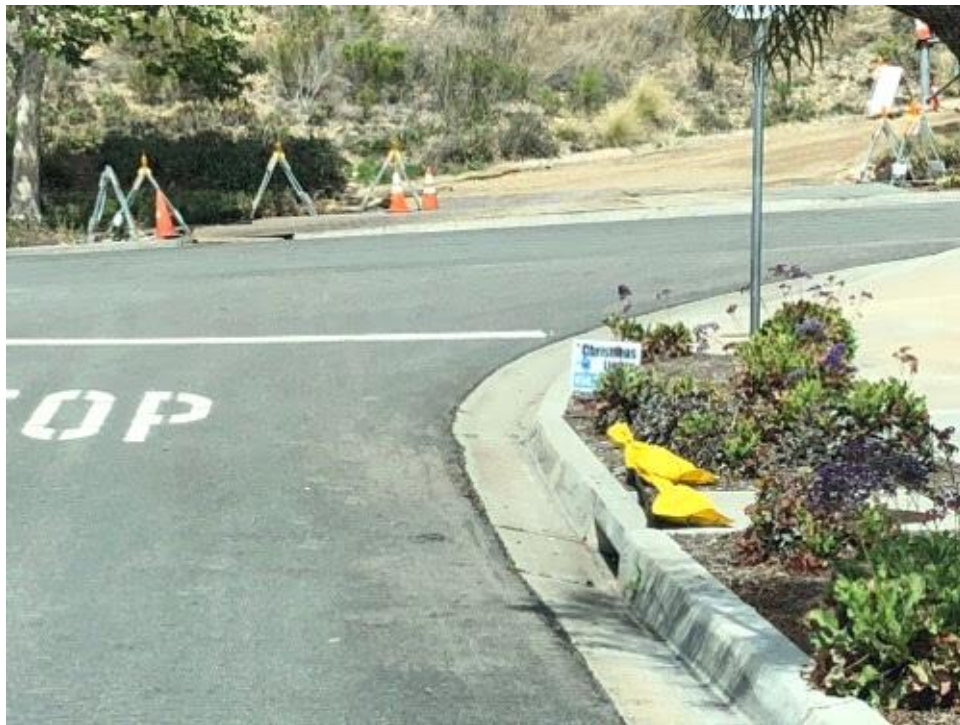
Caption BMPs pulled away from storm inlet to allow normal water flow during storm event.
