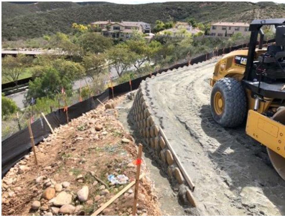
Caption Retaining Wall at P05.
