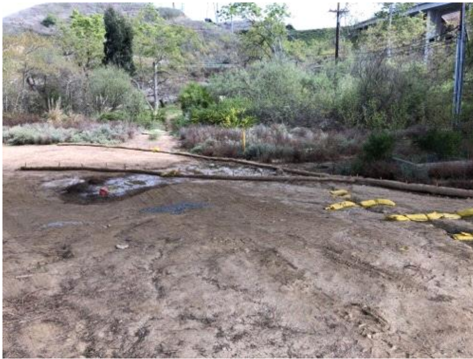
Caption BMPs beneath Carroll Canyon Bridge.
