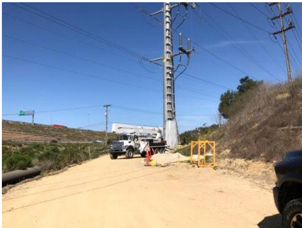
Caption Overhead work at CC MM CP.
