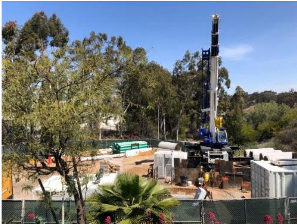
Caption West I-15 bore pit staging area.
