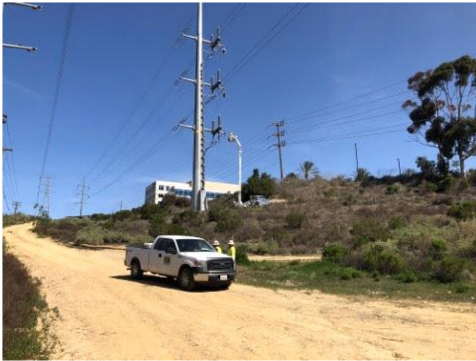
Caption Wire pull prep work with lift at CC MM CP.
