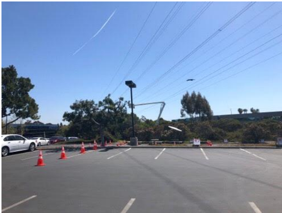
Caption Safety and traffic control measures implemented for overhead work.
