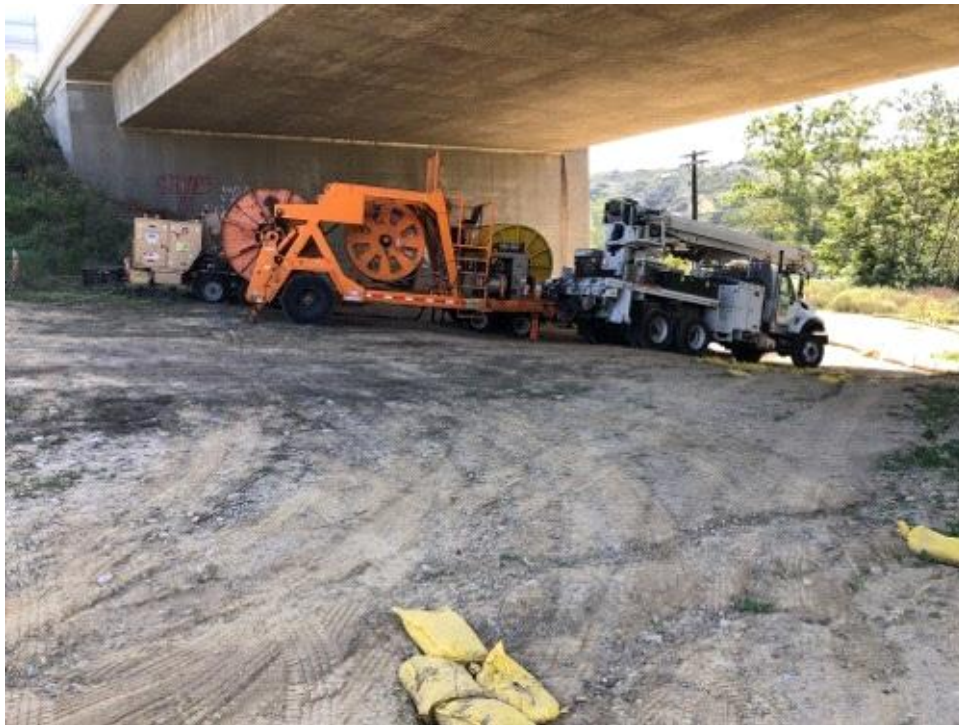
Caption Wire pull equipment beneath Carroll Canyon Road bridge.
