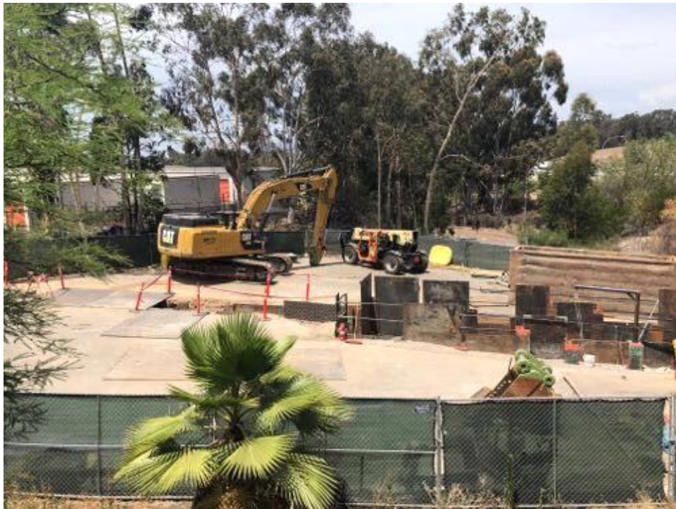
Caption Western bore pit.
