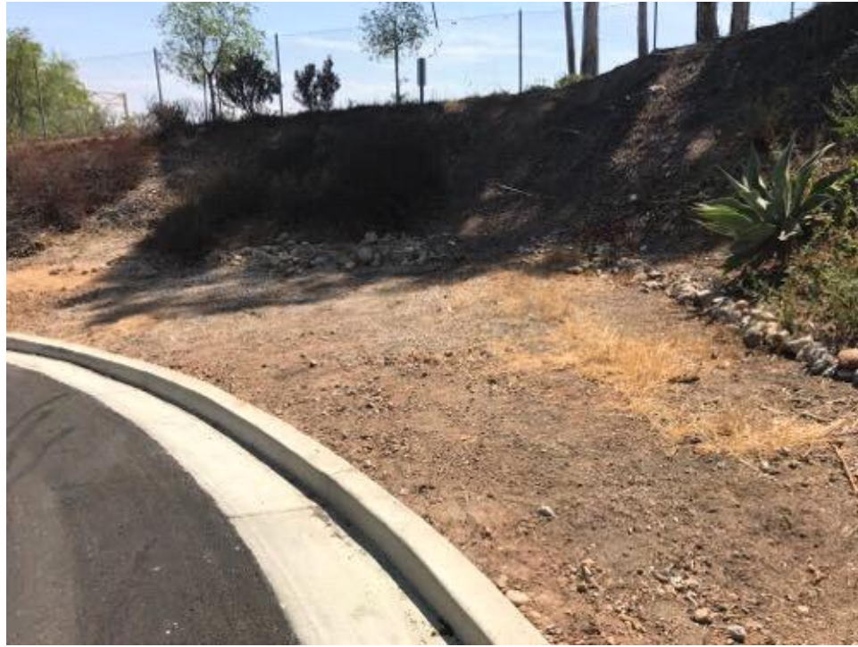
Caption East bore pit location will be sprayed with hydromulch on Sept. 5 for stabilization.
