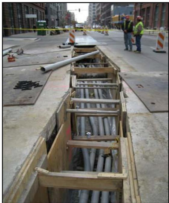
Figure 3 – Trench Installation
