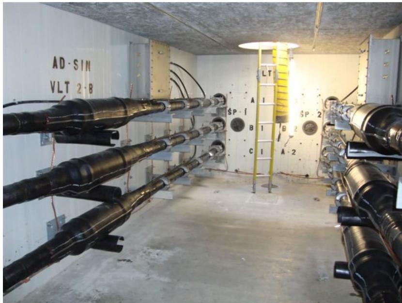
Figure 13 - Typical Cable Splice Vault
