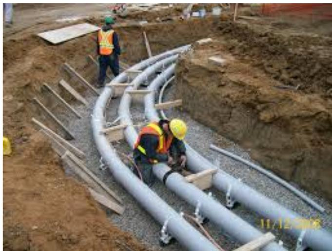
Figure 11 – Conduit Installation at a Corner
