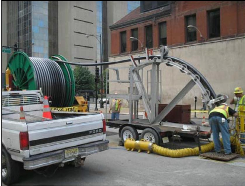
Figure 12 – Cable Pulling Arrangement
